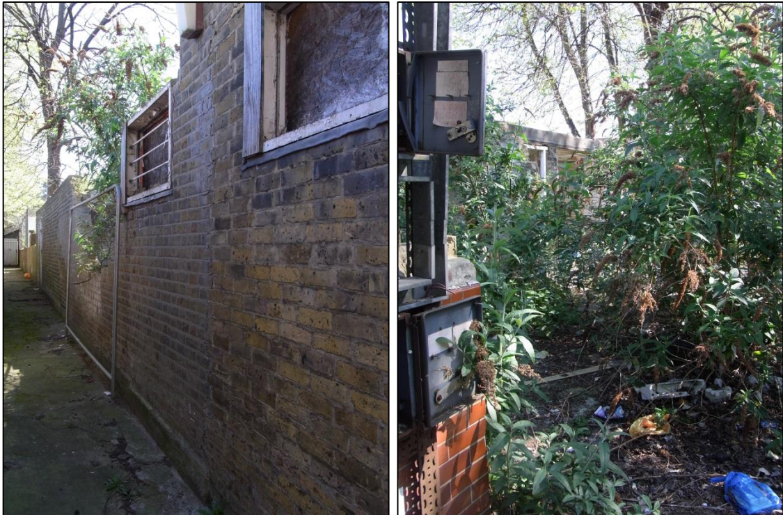
Plate 4: View along the eastern elevation of the ambulance station noting straight joint in fabric (left)
