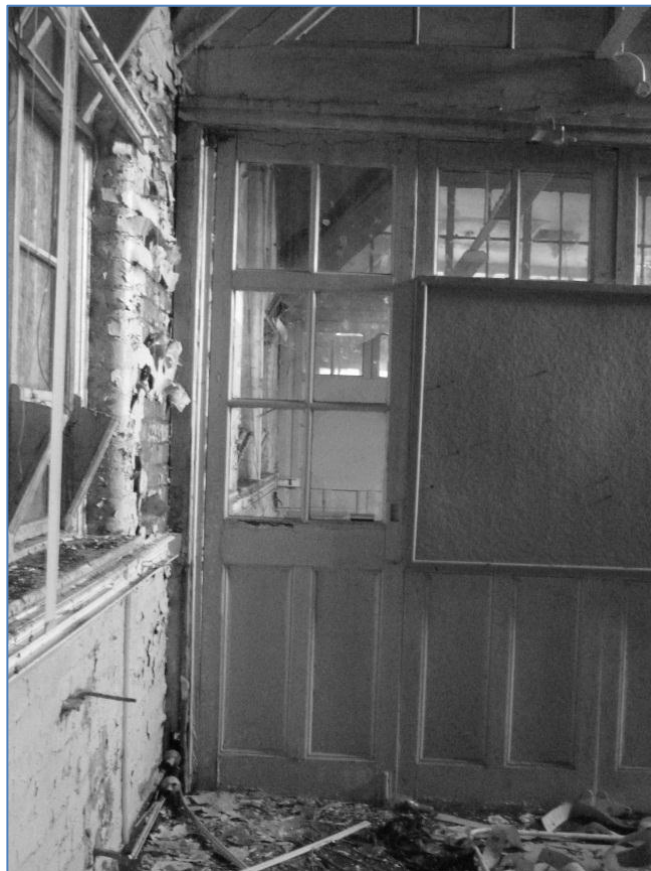
Plate 14: Detail of glazed partition panel (Digital 60)
