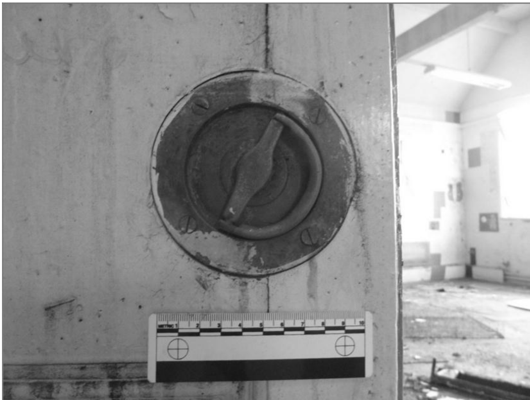
Plate 16: Detail of recessed door handle on glazed partition (Digital 56).
