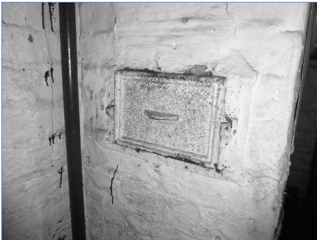
Plate 8: Detail of ash box in room B1 (Digital 46).
