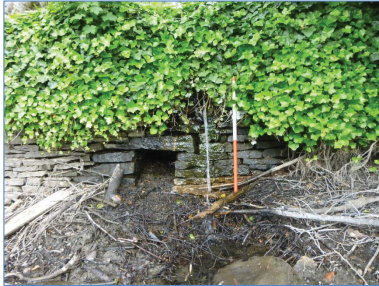
Plate 16: View of an inlet within the northwest corner of the dam, looking west.
