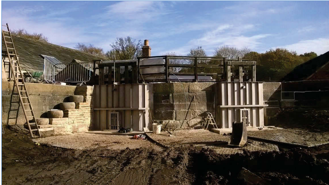
Plate 5: Penstocks following completion of works (image courtesy of J.N. Bentley)
