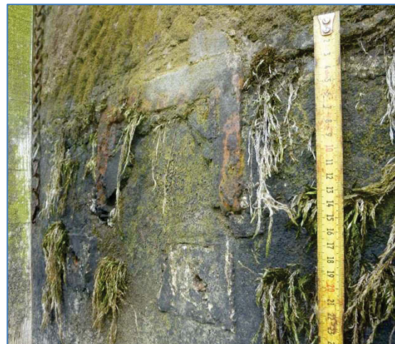
Plate 6: Detail of truncated 'C' section bar and two bolt holes below.
