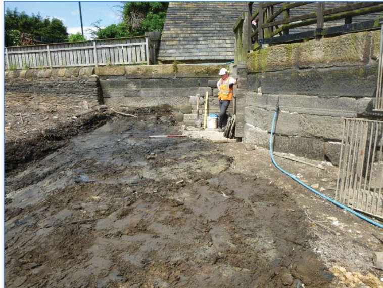
Plate 13: View of the exposed clay in front of the penstocks, looking north.
