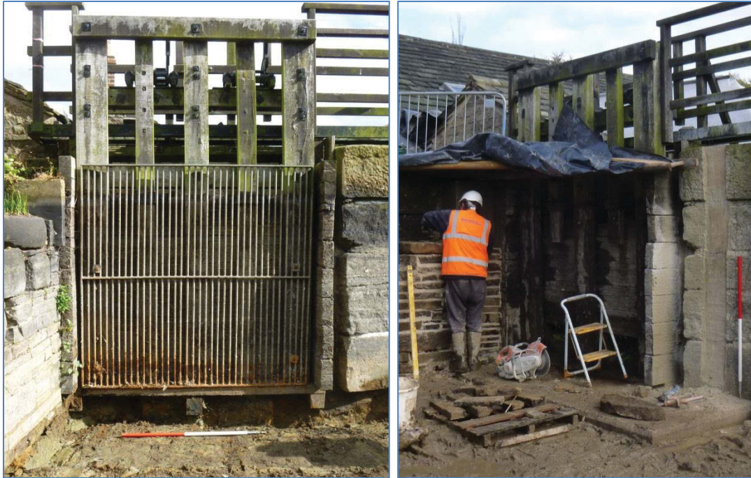
Plates 1-2: Detail of Penstock 1 as cleared and following pre-fit works
