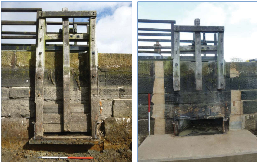
Plates 3-4: Detail of Penstock 2 as cleared and following pre-fit works
