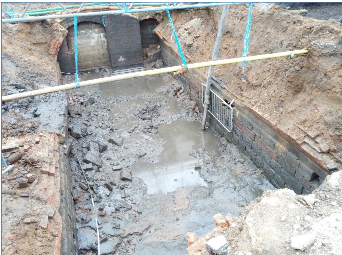
Plate 6: General view of the interior of the canal tunnel following the removal of the arch, looking south
