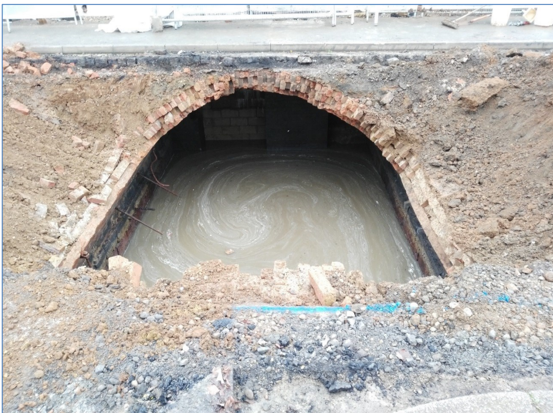
Plate 9: Image taken during breaking out of the arch, looking south, illustrating its construction
