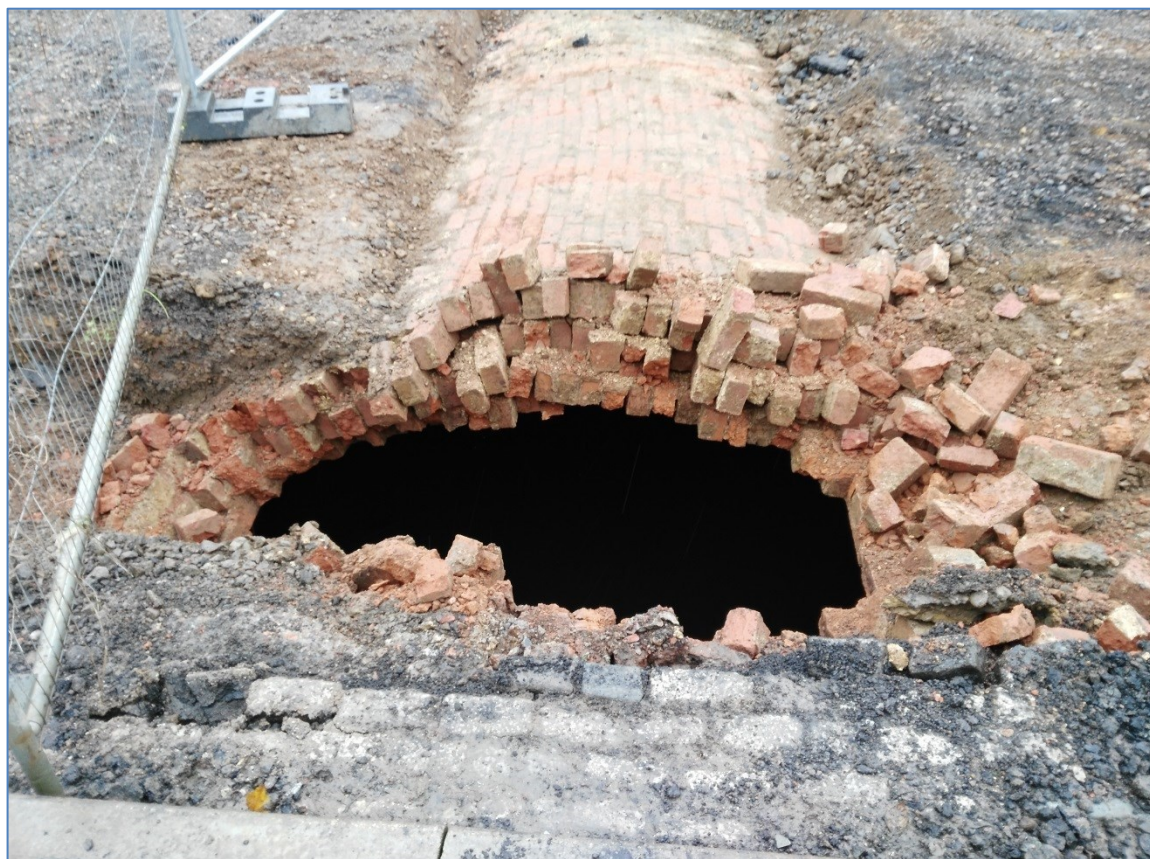
Plate 3: View of section through the top of the tunnel facing south
