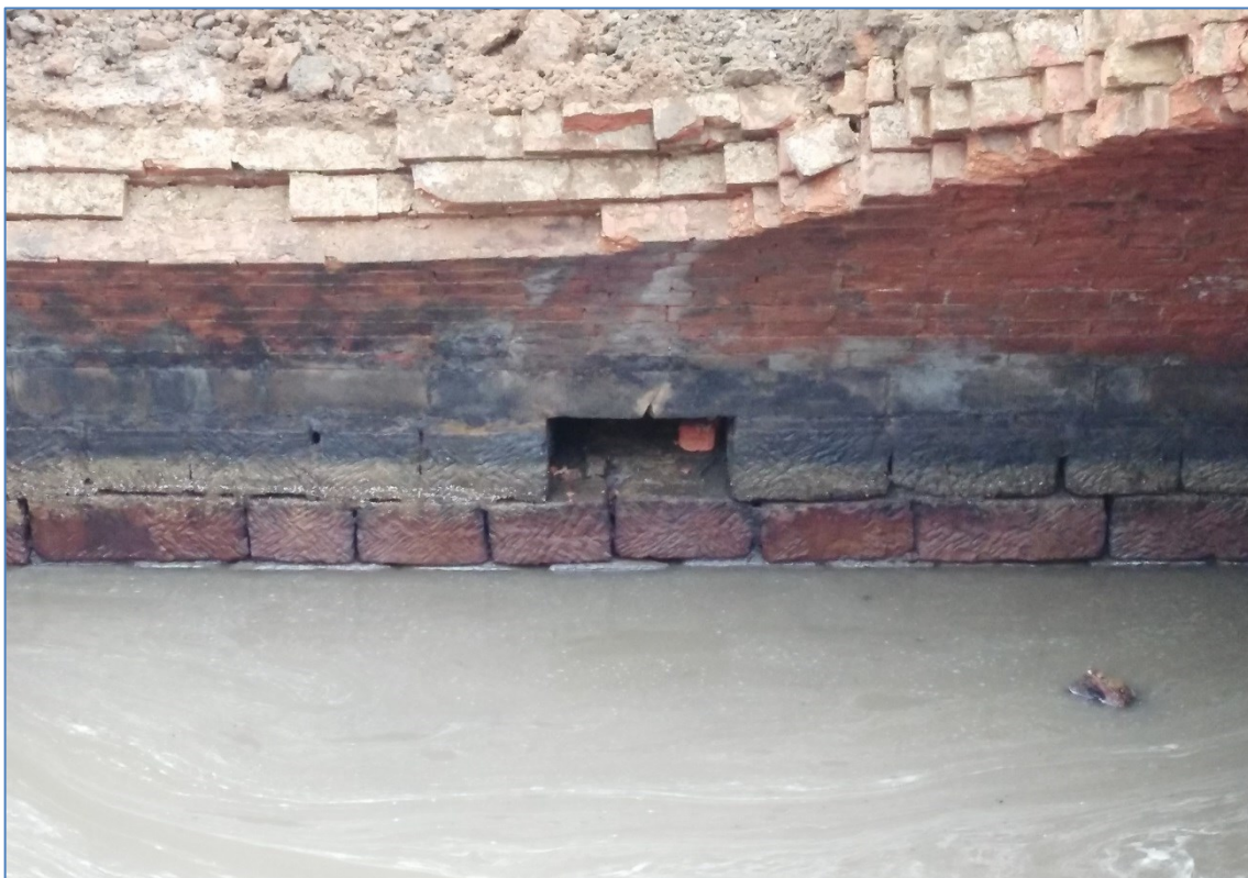
Plate 8: View of the rectangular void within the centre of the west facing elevation of the canal tunnel wall. An identical void was present within the opposite wall.
