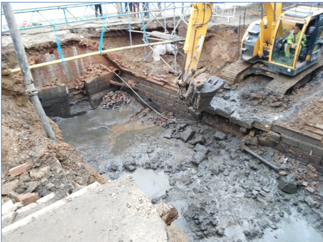
Plate 7: General view of the interior of the canal tunnel following the removal of the arch, looking north
