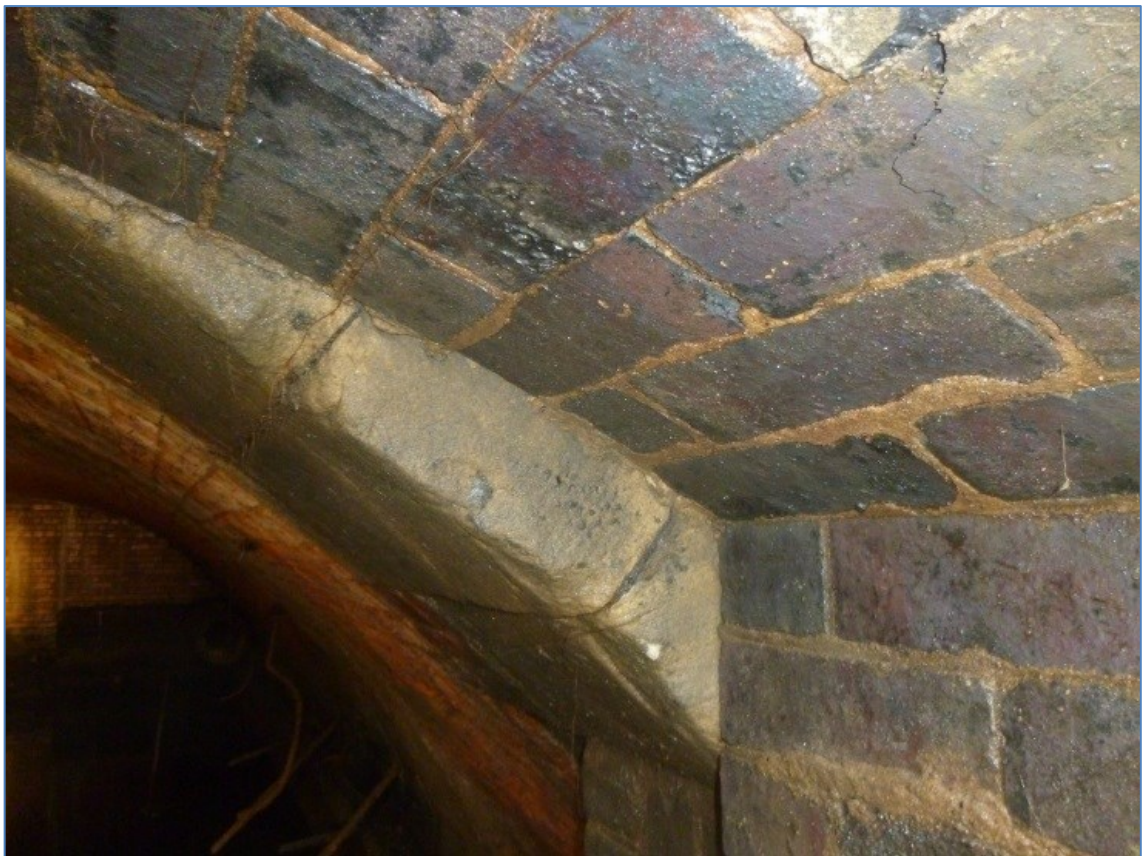
Plate 5: Detail of sandstone voussoirs of the canal portal (2014)
