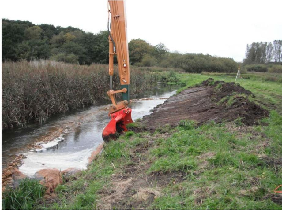
Plate 1 Excavation during of creation of berm
