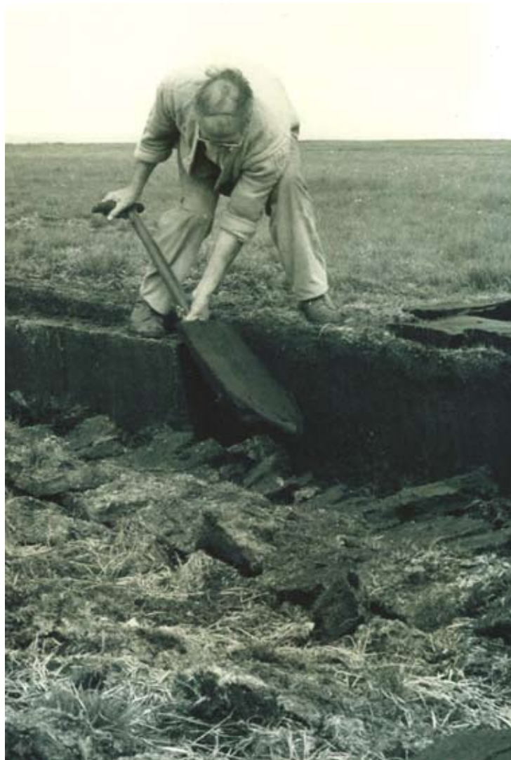
Fig 11 (left) Sante Lafuente demonstrating the craft of turf cutting to Ernest Mold, c 1980, probably on Brendon Common. He is standing on the cleared area ('bench') which is exactly the right width for working the peat face (Lyn and Exmoor Museum)
