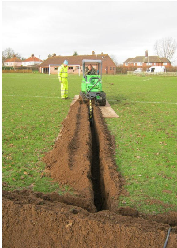
Plates 2 & 3: Cable trenching across the football pitch (looking north-north-west) and the eastern half of the GSHP ground loop installation trench (looking south).
