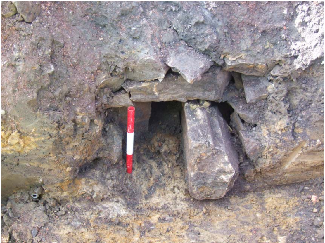
Fig. 3 Section through the stone-lined culvert.
