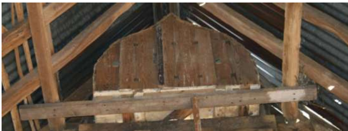
Clinker built dovecote with hinged panels for access to the rear.
