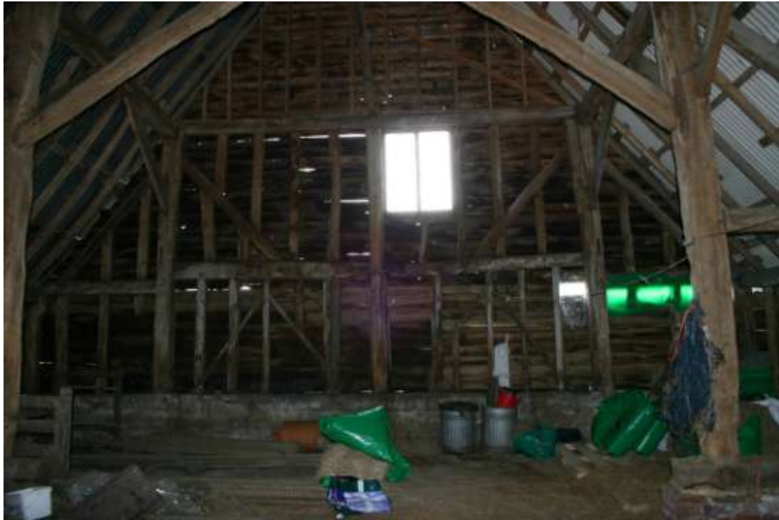
Photo showing the sag of the rafters and the rebuilt south wall.
