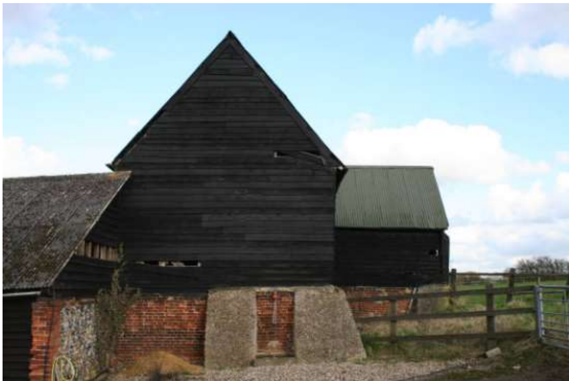
Western elevation showing concrete buttresses.
