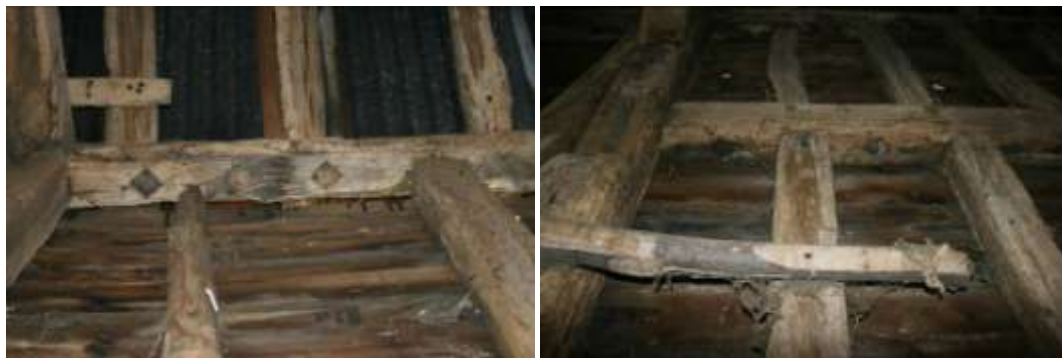
Top-plate (left) in Bay 1 and midrail in Bay 4 have diamond mortices for heavy mullions.
