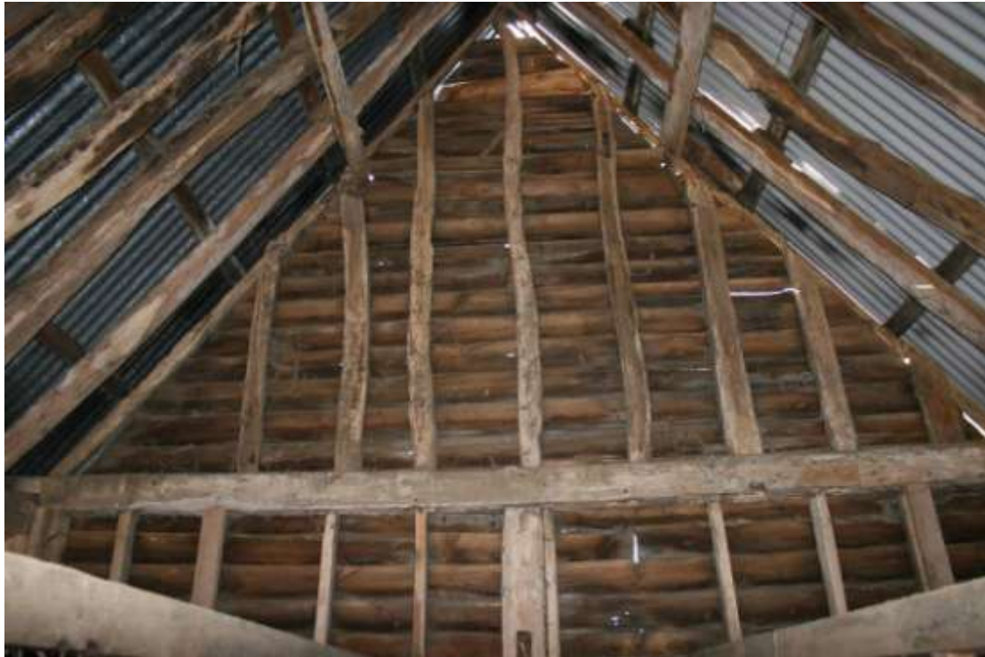
The upper sections of the gable ends have old rafters used as studs. Looking W.
