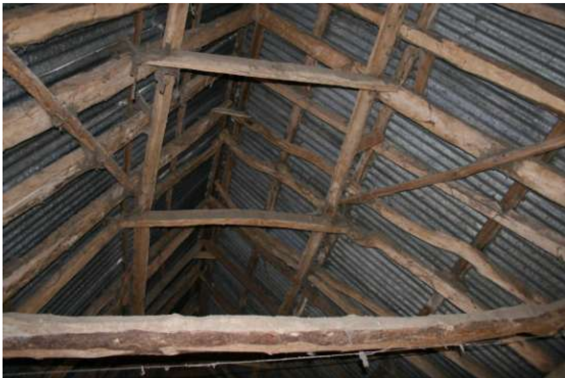
Clapsed side purlin roof with reused rafters and tree poles. Looking E.
