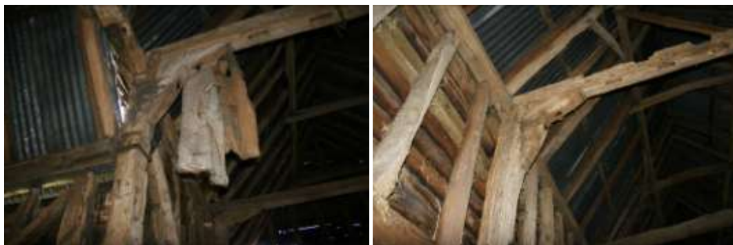
Wrought iron tie on the midstrete post. Square headed bolts on the hanging knees.
