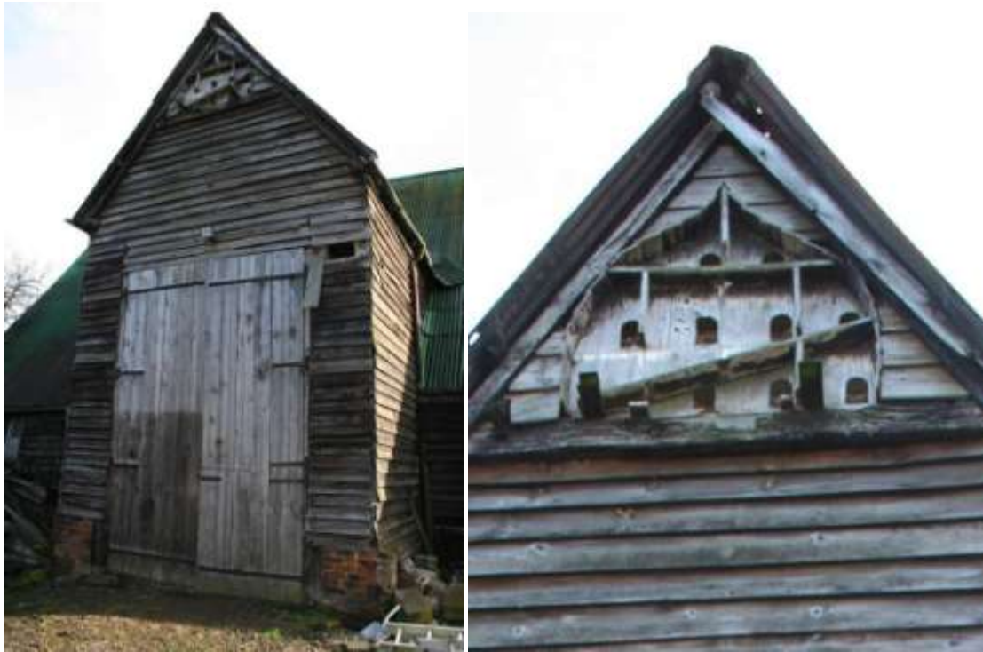
Full height doors and above a dovecote made from an upturned boat hull.
