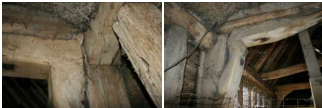
Square post in the north wall has tiny upstand. Hanging knees made from tree roots.
