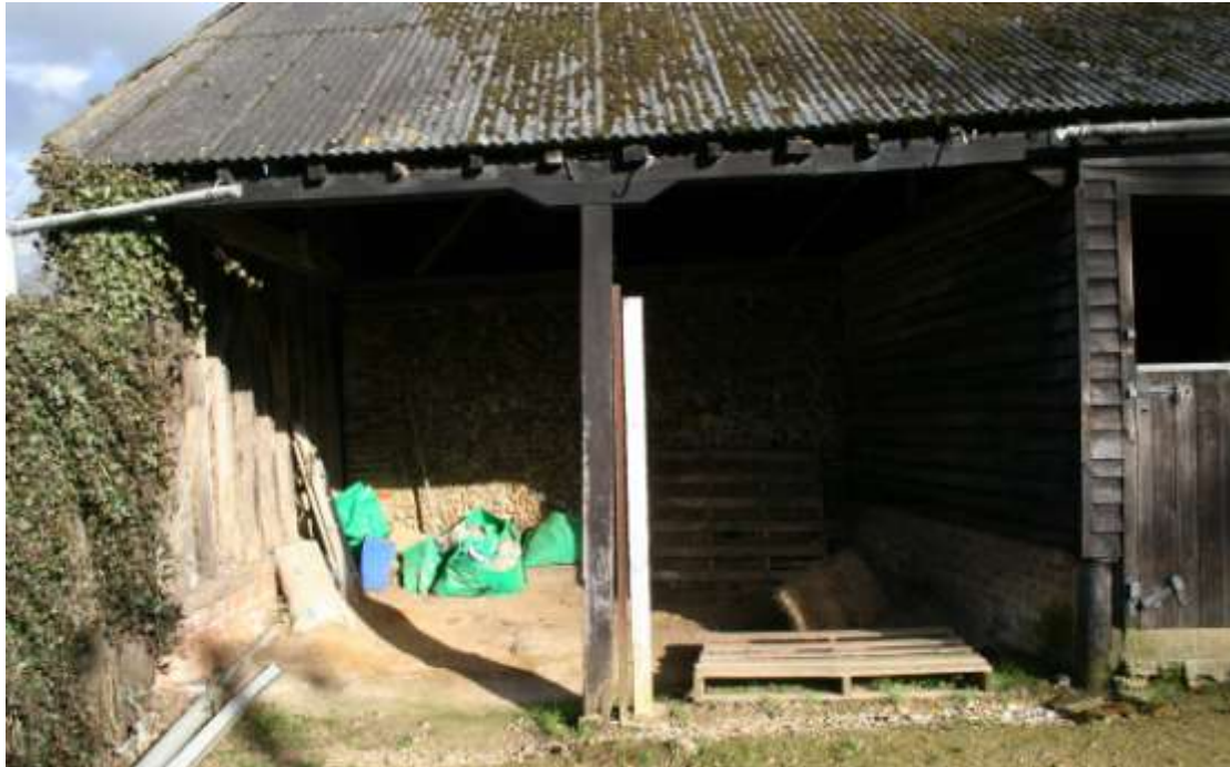
The open bays at the northern end. The axial brick wall can be seen to divide the building.
