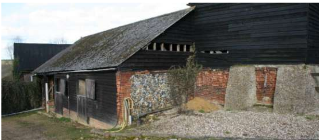
The southern elevation has a brick and flint wall.
