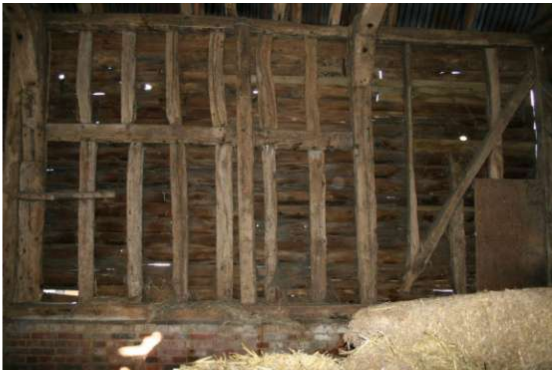
South wall, Bays 4 and 5. Studwork from an earlier house and Georgian nailed bracing.
