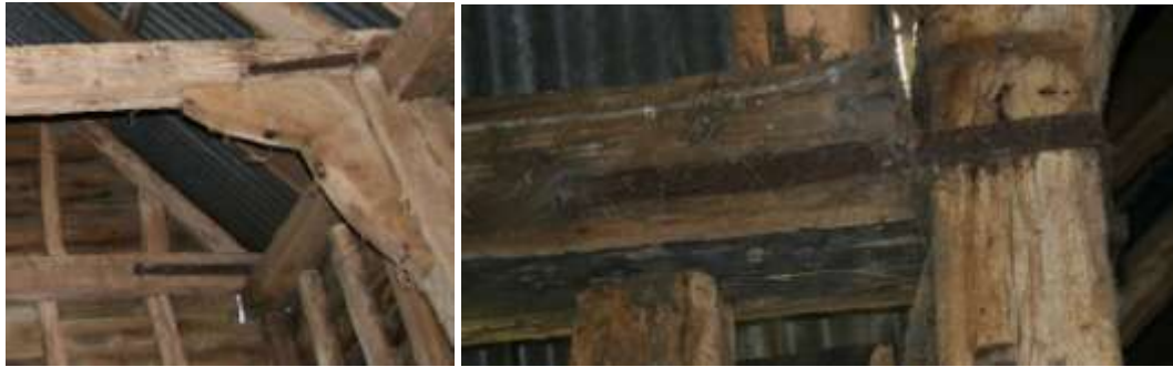
L-ties on the tie-beams with bolts through the hanging knees. Mild steel L-tie on midstrey.
