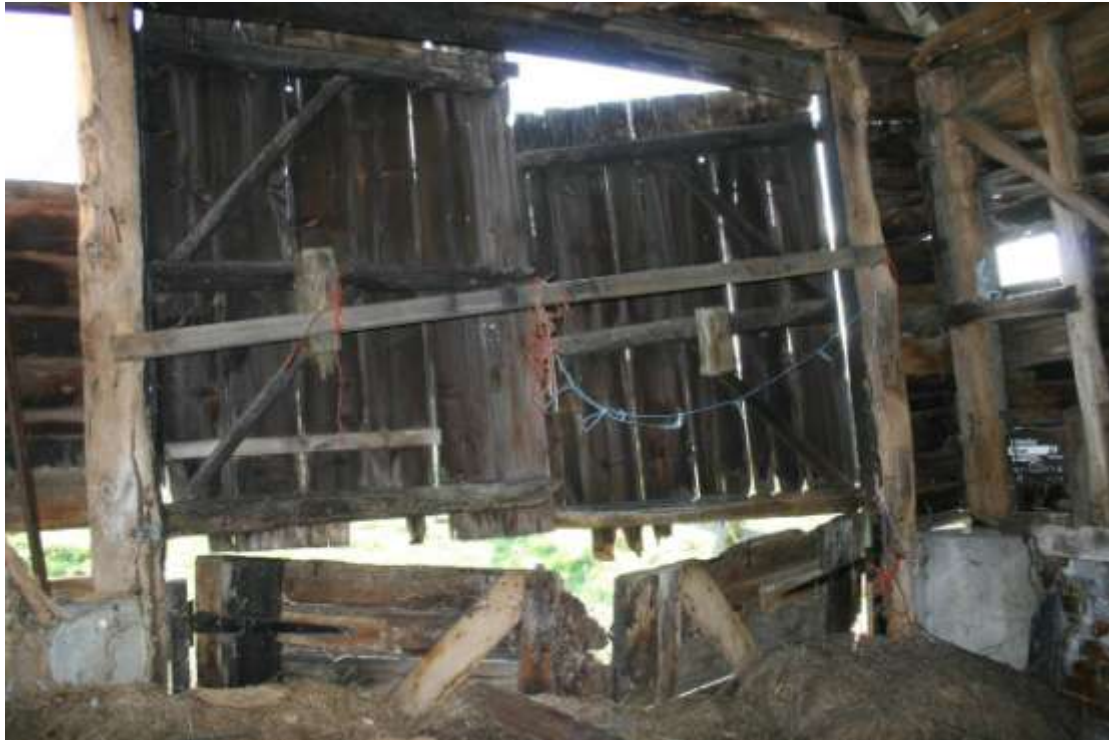
South doors in the midstrey porch. The upper doors may be original, the lower home-made.
