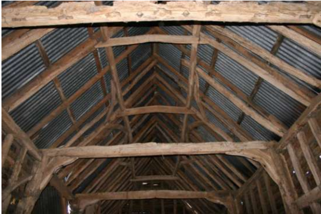
The roof structure looking east. Note curved windbraces and diamond mortices in tie-beam.
