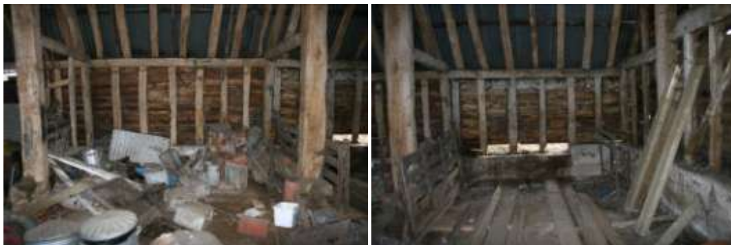
Comparing Bays 4 and 5 on the eastern side. Note awkward disposition of studs in Bay 5.
