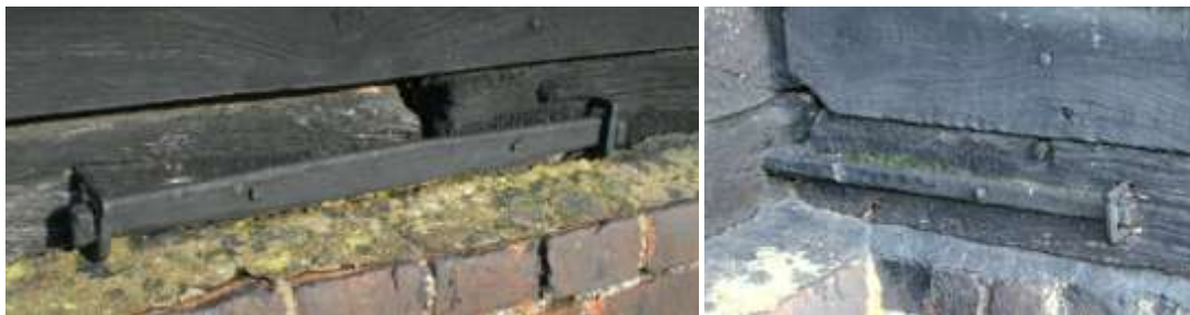
A wrought iron flat strap and a pin-tie both held with nails and square staples.
