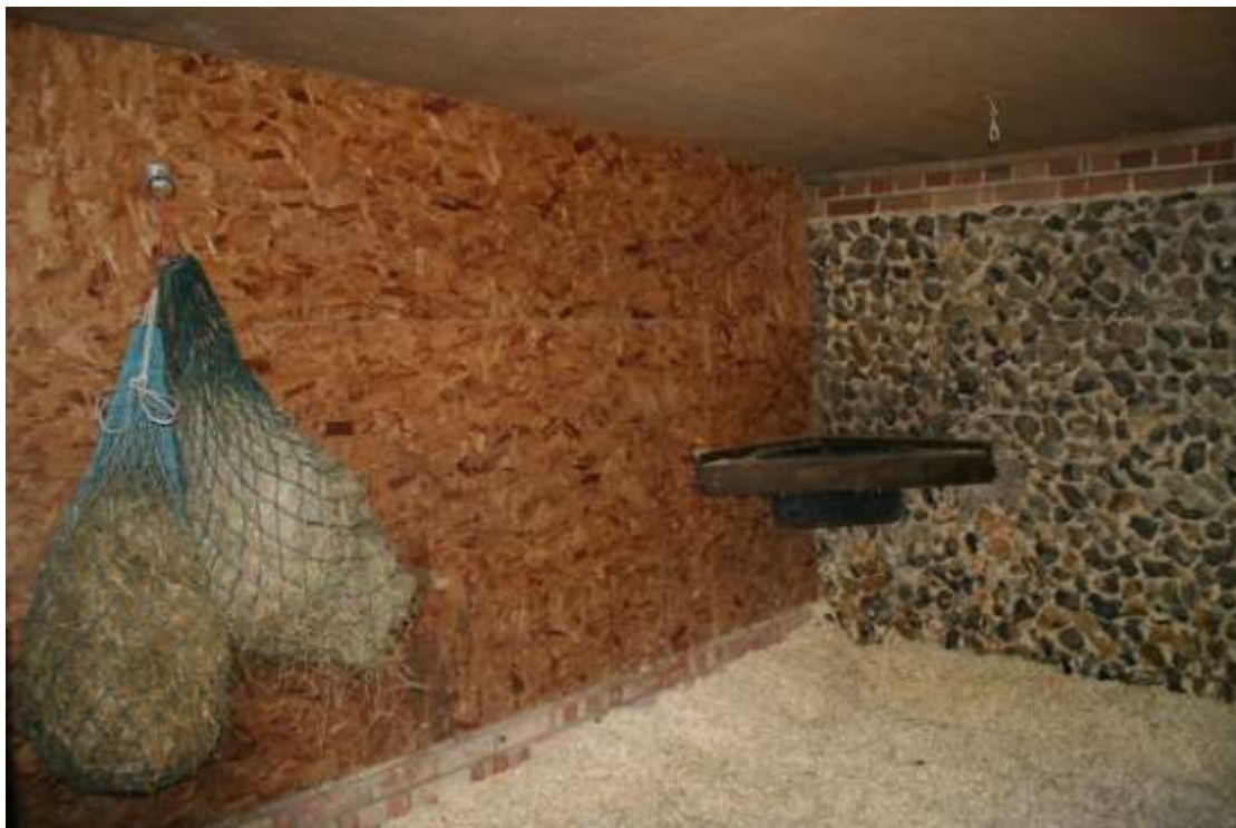
Stalls on the east side have C20th plastic corner bowl and hay nets. Walls are clad with OSB.
