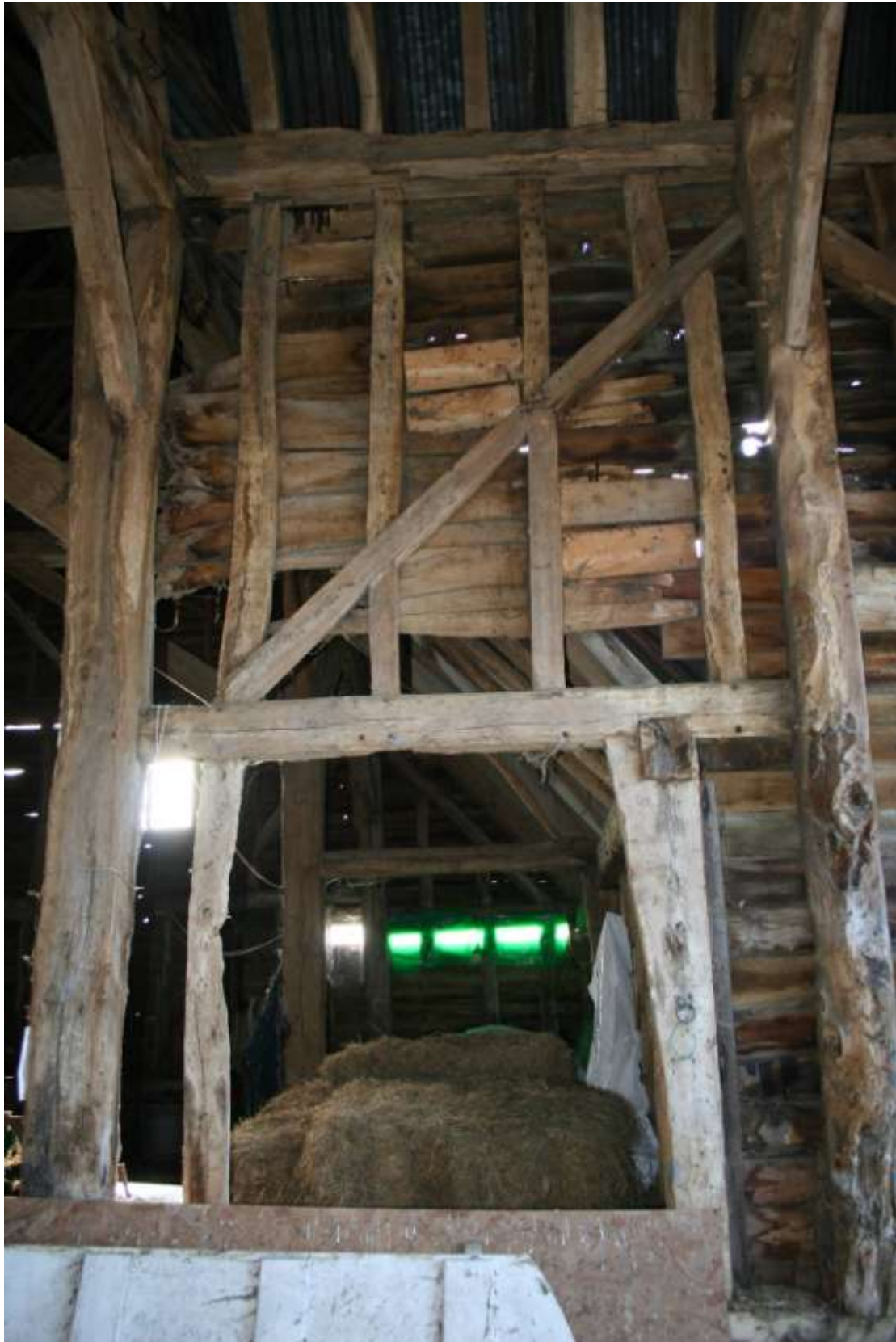
The southern side of the midstrey porch. Note scarf joint at top, interrupted studwork and unusual wall post. The midstrey post to the right is not oak. Initials WN are carved by the lashing ring.
