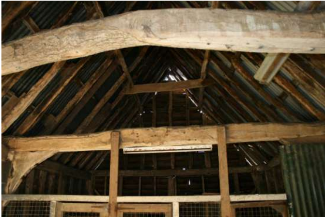
Main tie-beams are re-used oak. Central tie-beam is bark covered elm.
