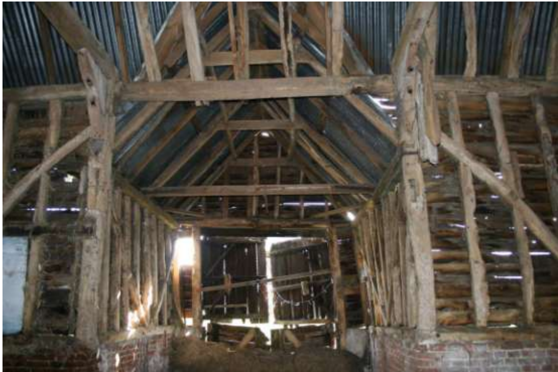
Looking south into the midstrey porch. Note interrupted studwork and reused timber.
