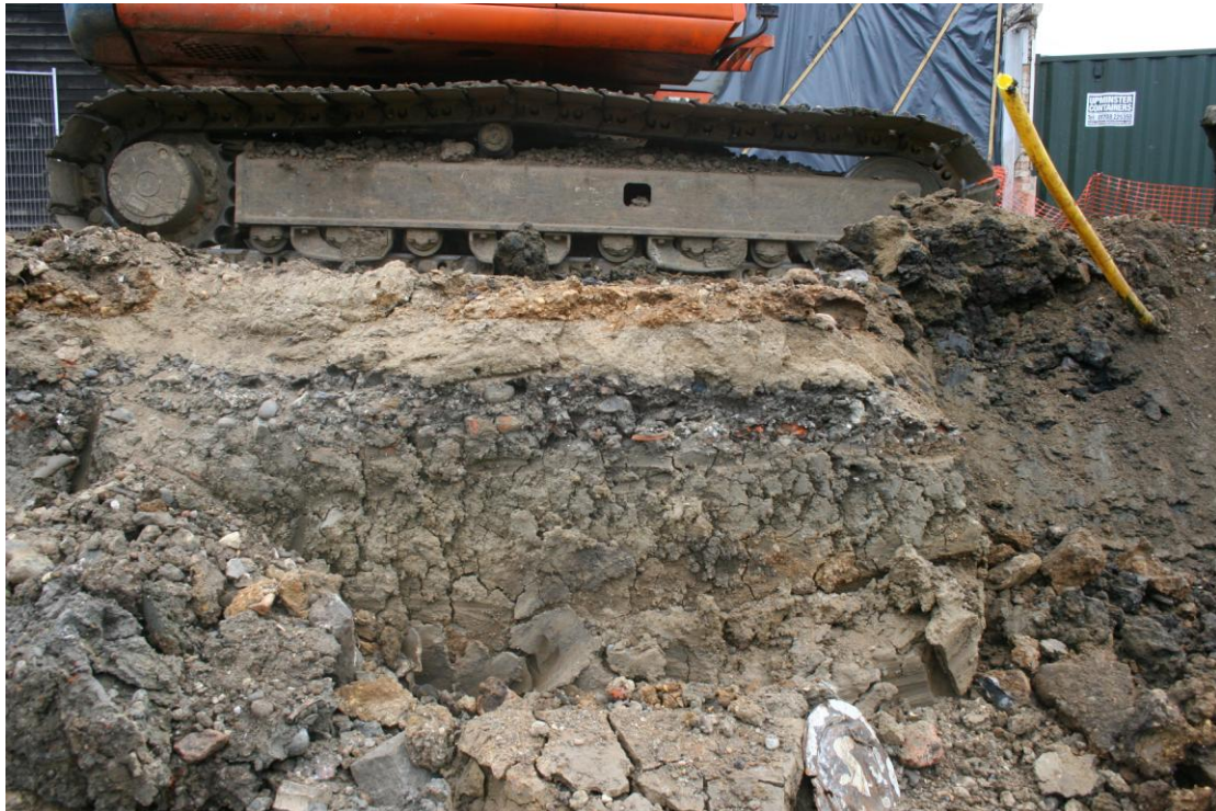
Layers of road make up adjacent to the Maintenance Workshop. Looking E.
