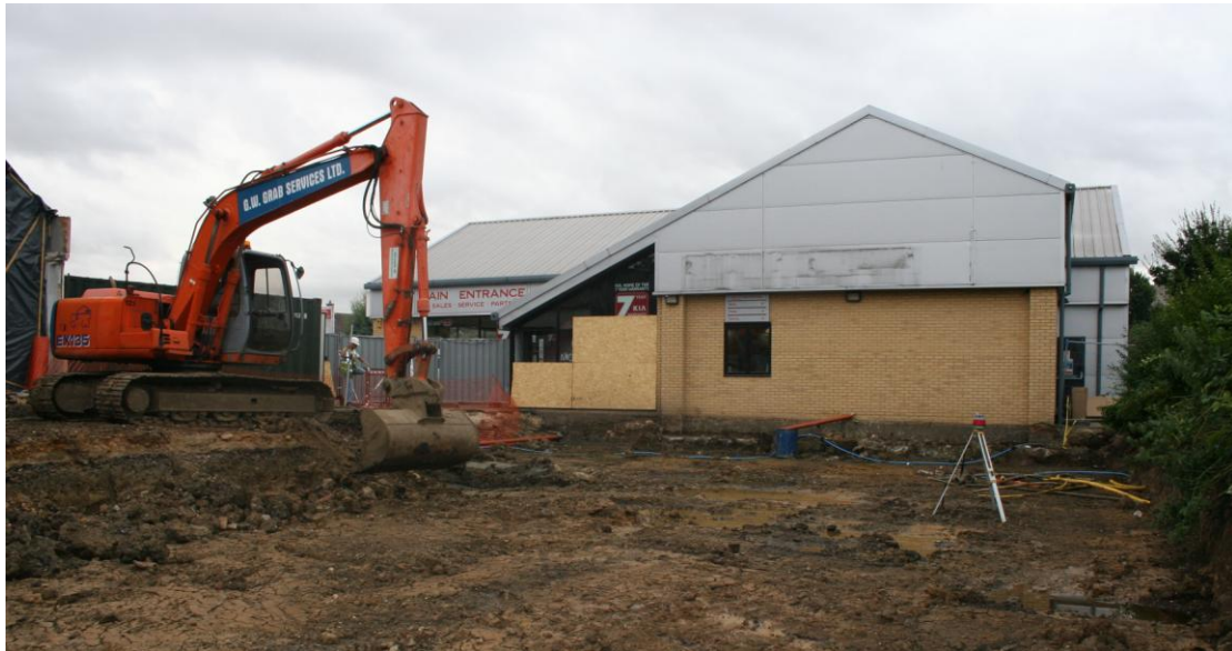
Excavator with ditching bucket. Looking S.
