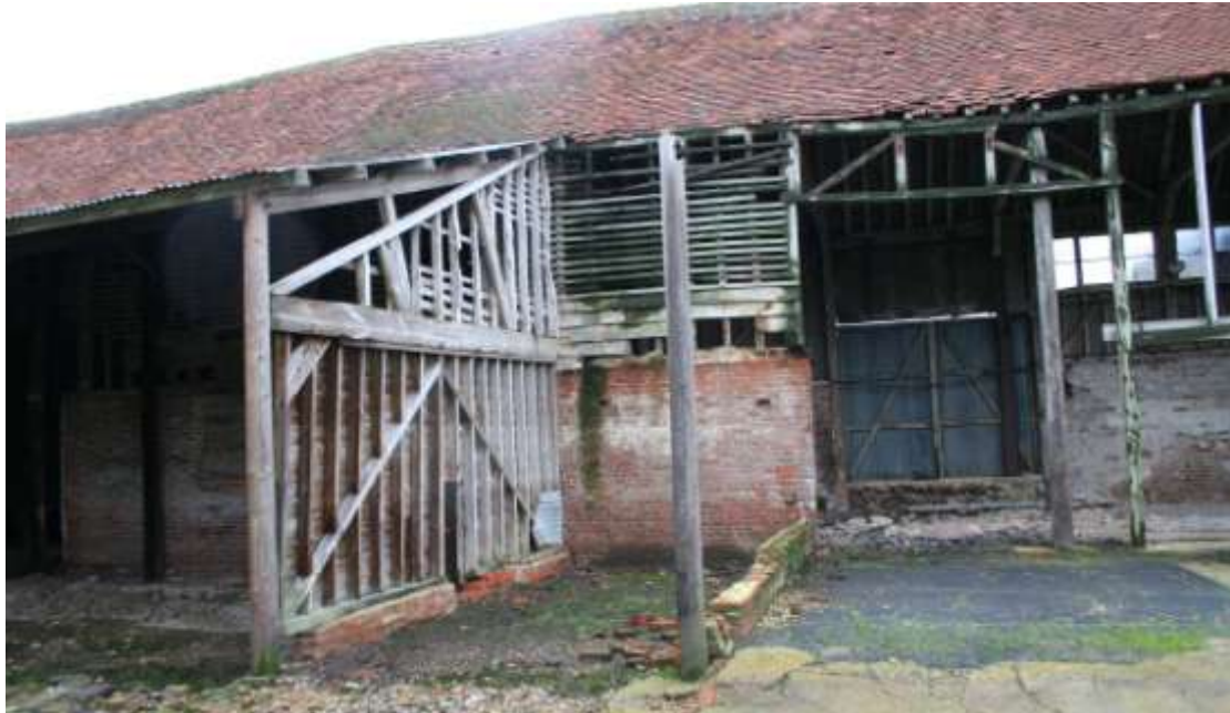
The partition wall ending Bay 7 is a LC20th rebuild.
