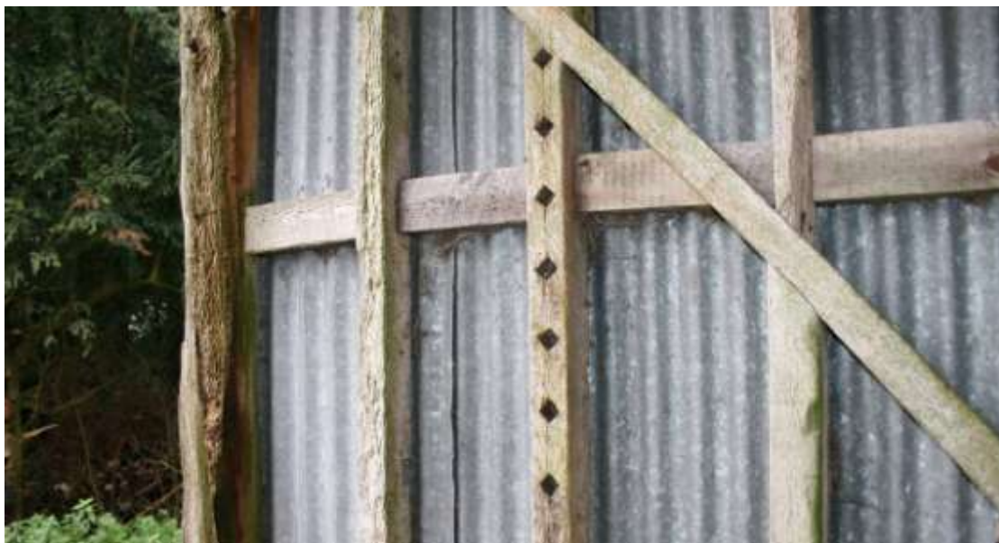
Detail of the repaired scantling frame.
