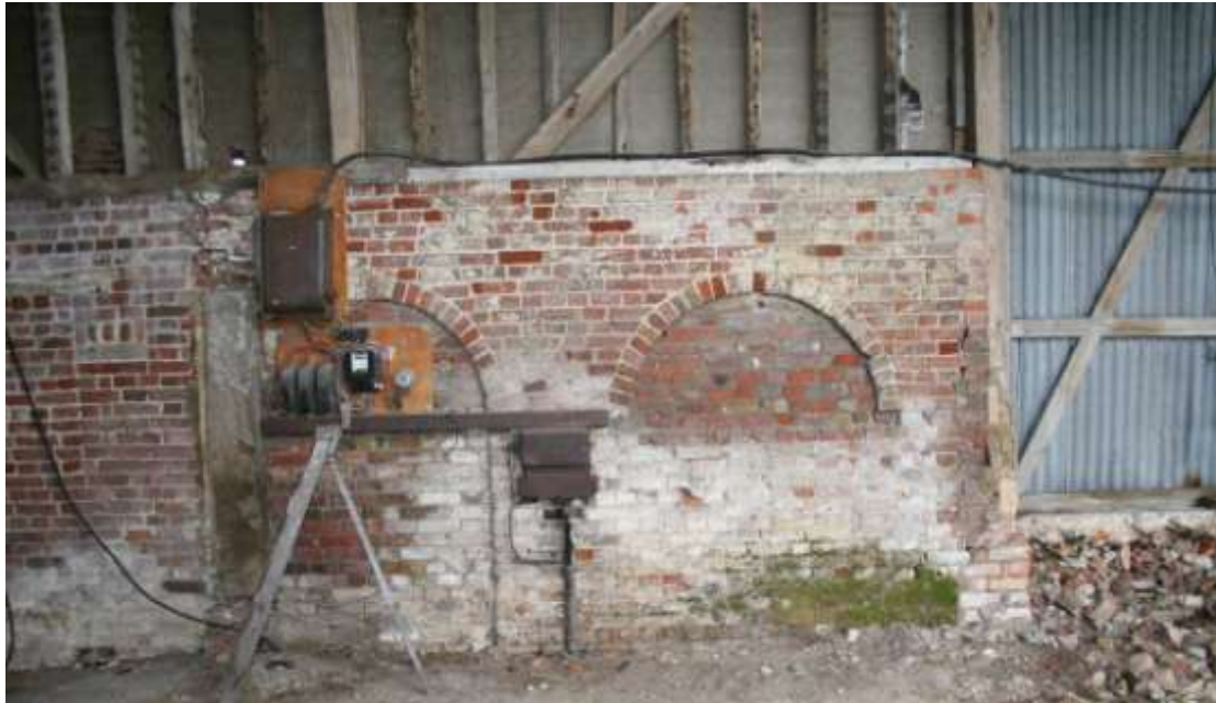
Blocked arch headed openings in Bays 9 and 10.
