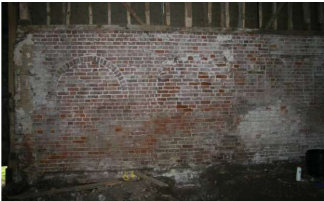
North wall Bays 4-5. The arch headed doorway and window have been blocked.
