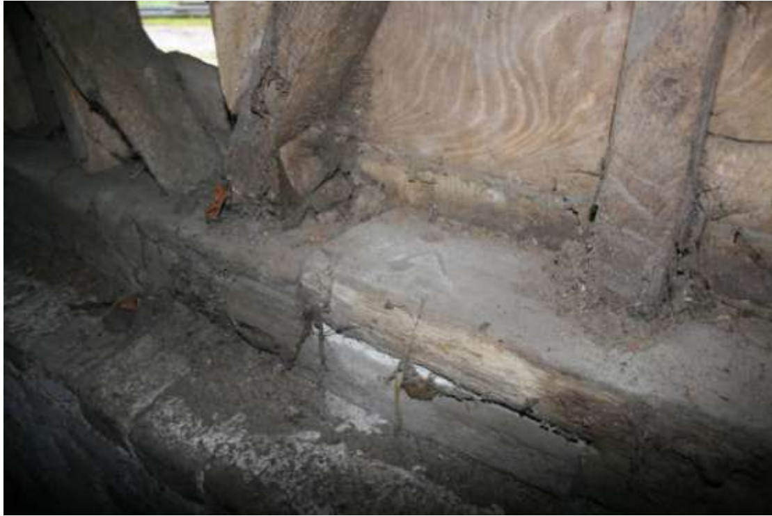
Carpenter's mark on the scarf on the south wall under Truss 4.
