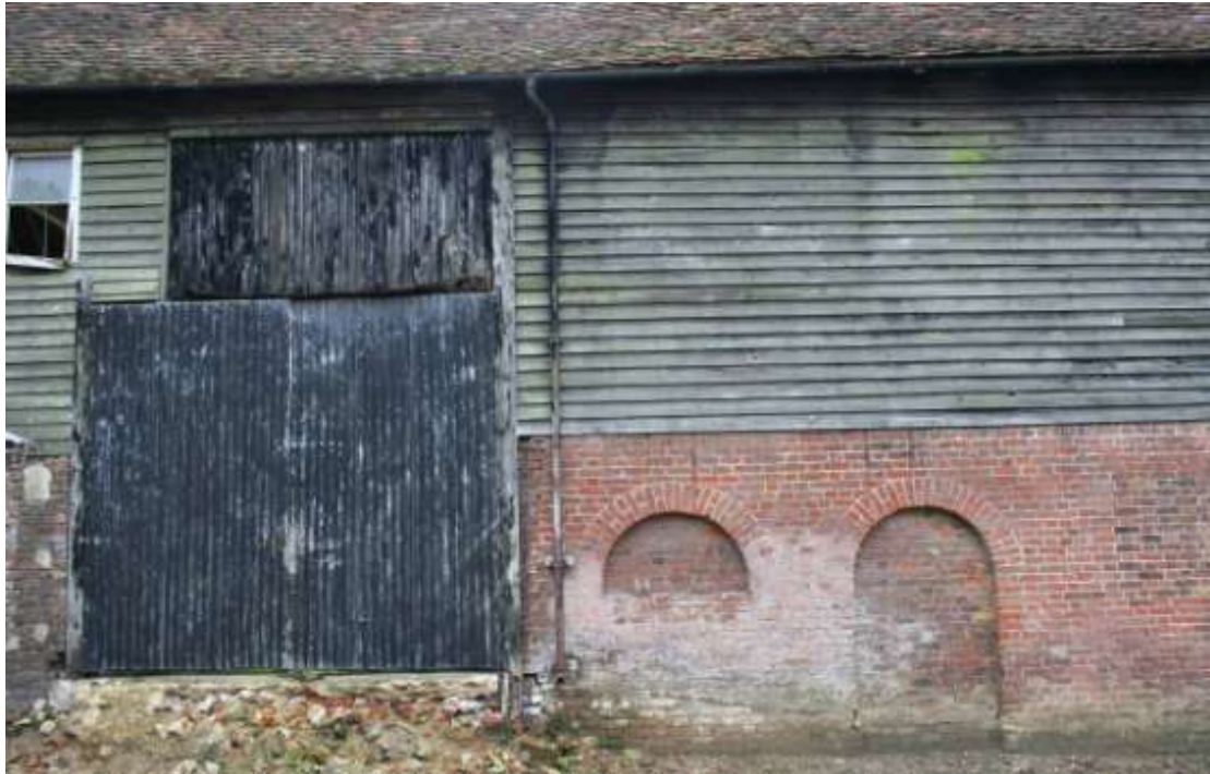
Enlarged full height doors and blocked arch headed window and doorway.
