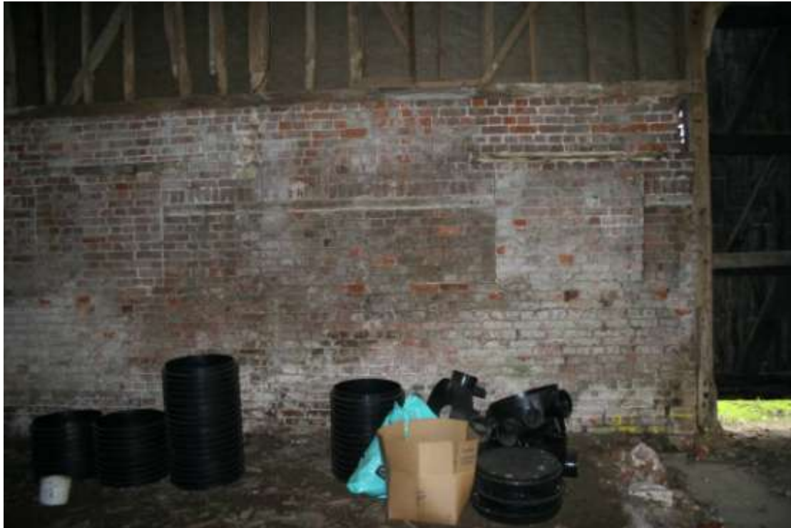
Two blocked windows in Bays 5 and 6.
