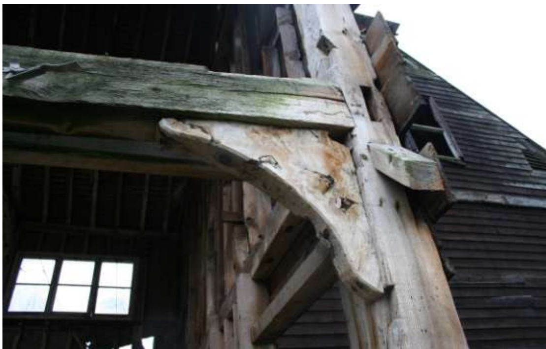
Junction of the corner post and mid-rail.
