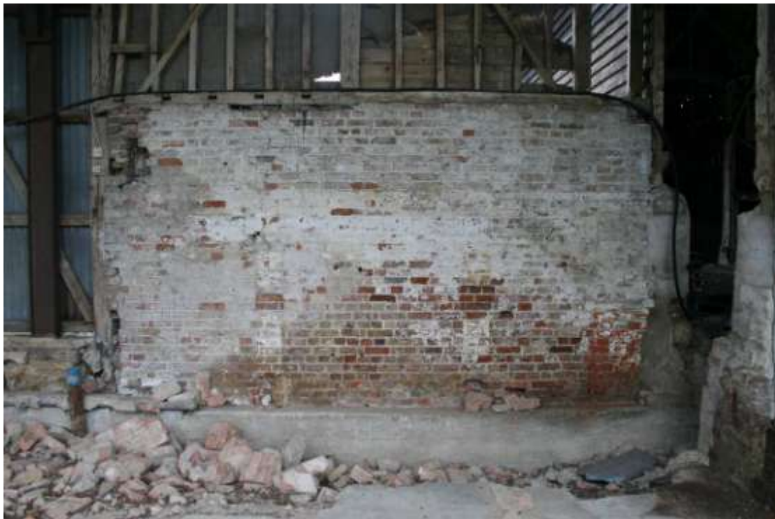
Bay 12 and 13. Later Stock brickwork wall.
