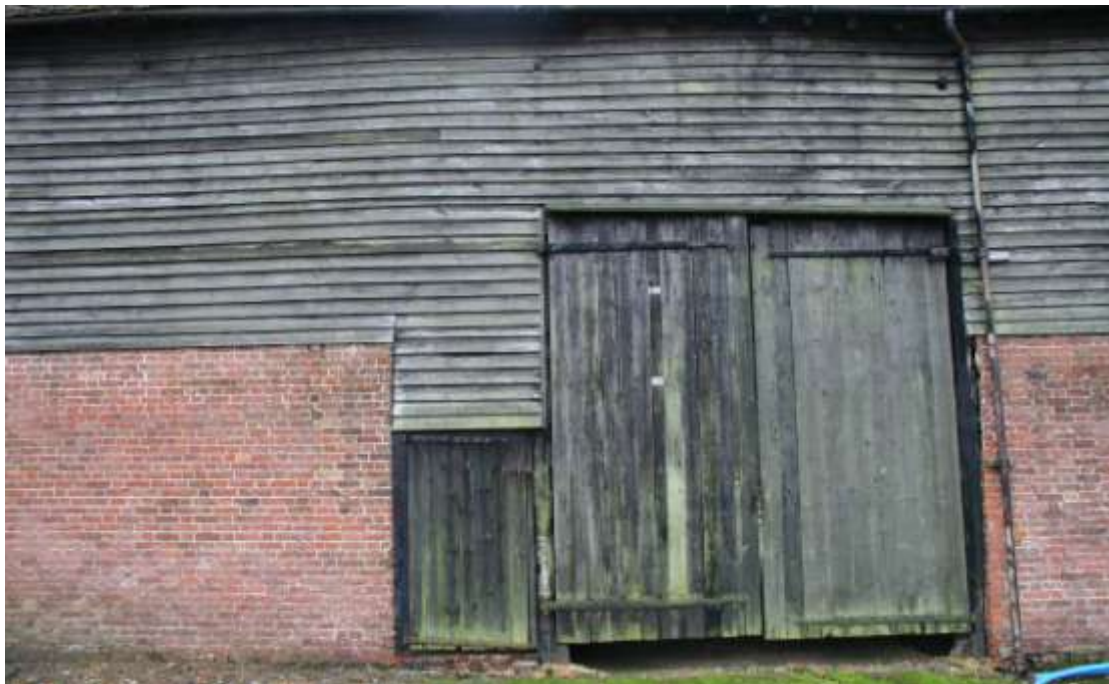
The central doors with pedestrian door. Note the 'leap' sockets on the door jambs.
