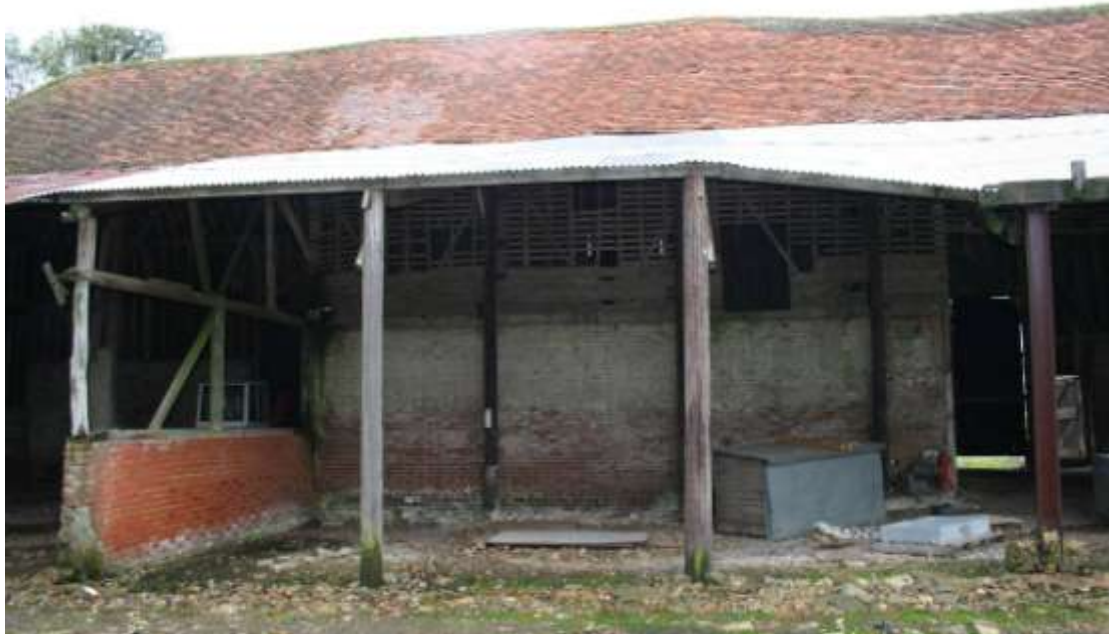
Southern elevation. Bays 4-6. Note the added brick plinth.
