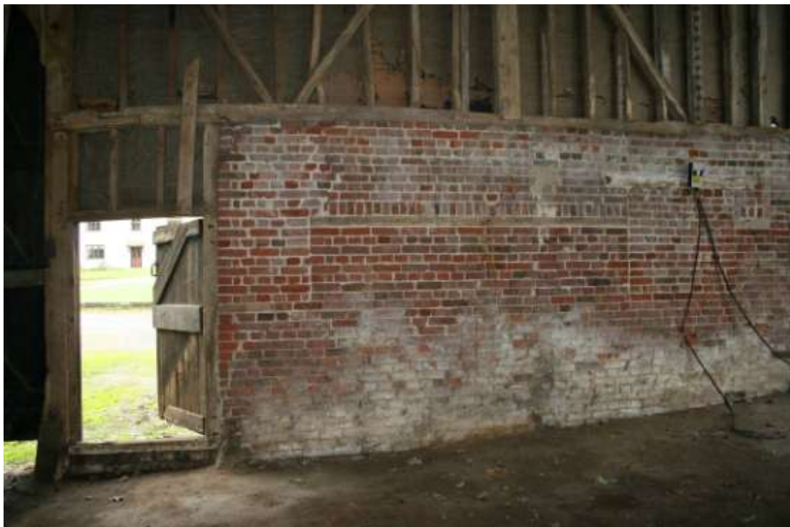
Two blocked openings in Bays 7 and 8. The LHS one has been altered for the doorway.
