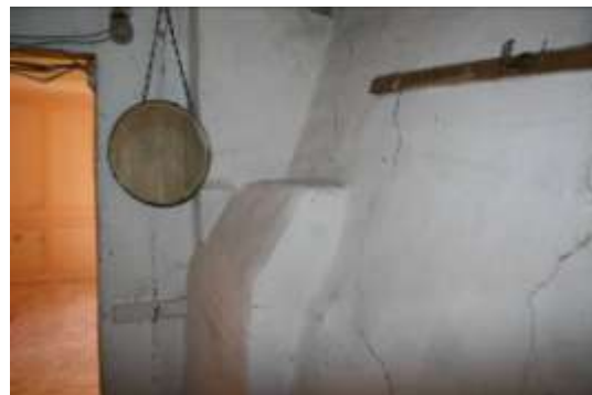
The closet to the side of the fireplace shows the plastered firestack.
