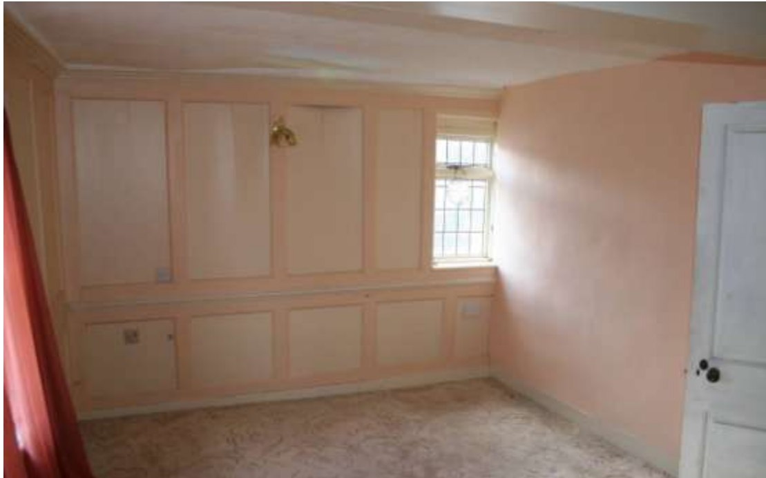
Looking SW in Bedroom 2. Note the window bisected by the inserted wall.
