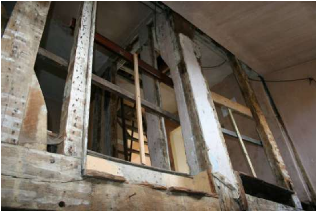
Looking upwards towards the Landing. Note the two doorways for previous staircases.
