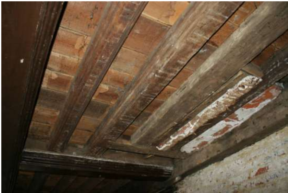
The timber-framed floor above the fireplace. Looking NNW.
