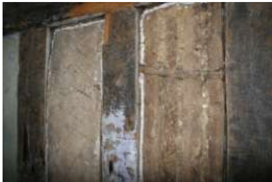
Detail of the wattle and daub panels in the northern wall.
