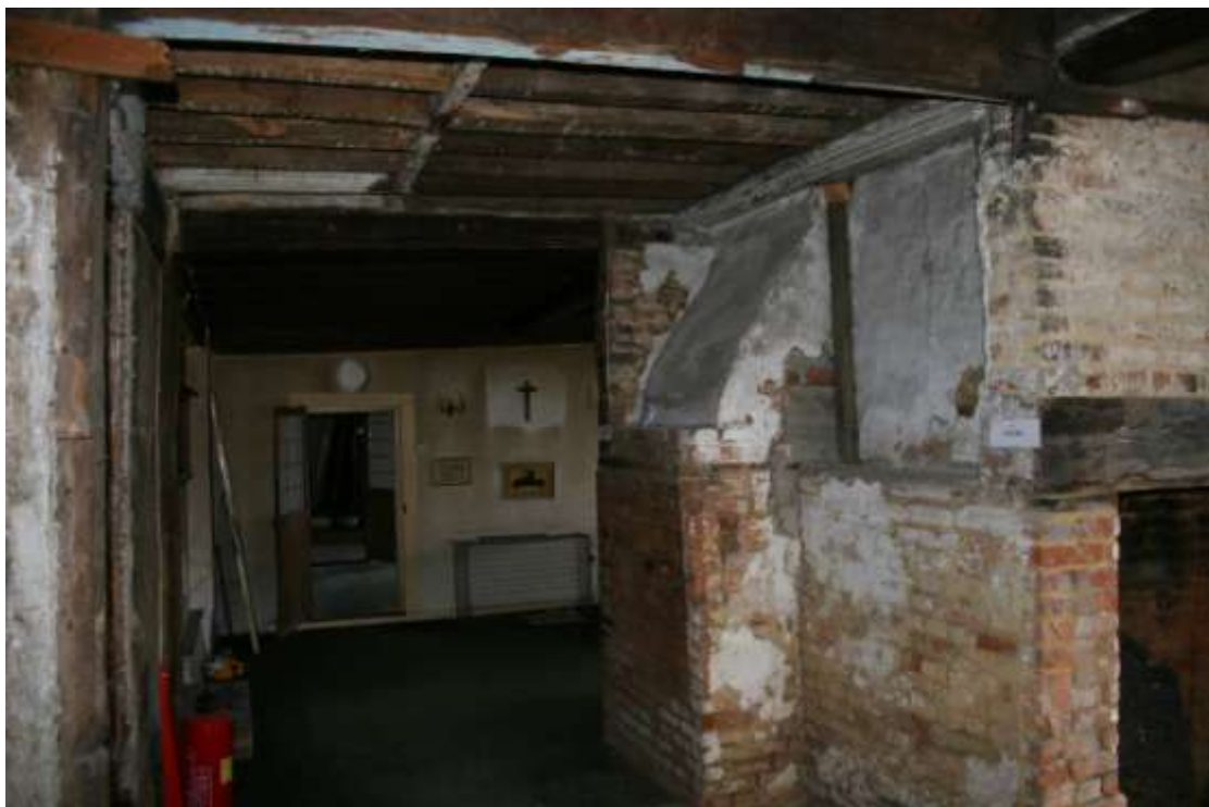
The area besides the two firestacks has a stair-trap later filled in.
