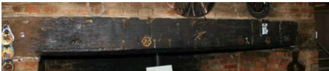
The bressummer has apotropaic marks and taper burns.
