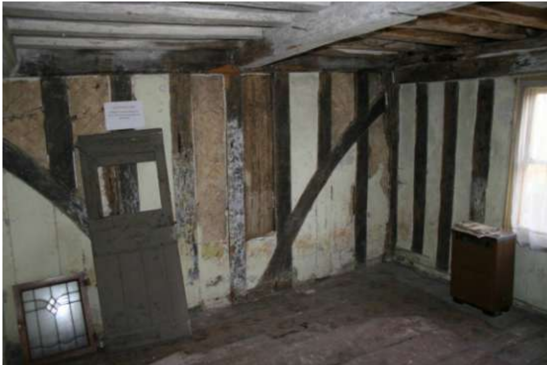
Looking NE in Bedroom 3. The walls retain their wattle and daub.
