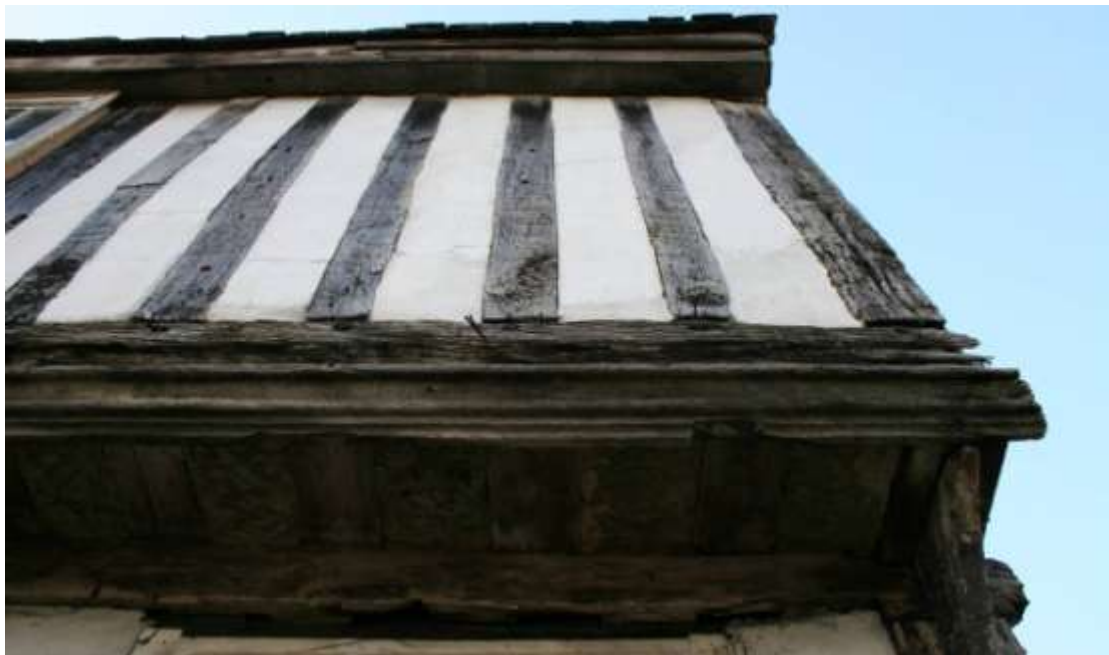
Looking at the underside of the jetty. Note the scratch coated lime render.
