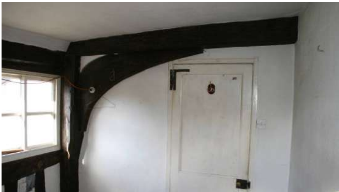
The frame and two panel door in Bedroom 1.
