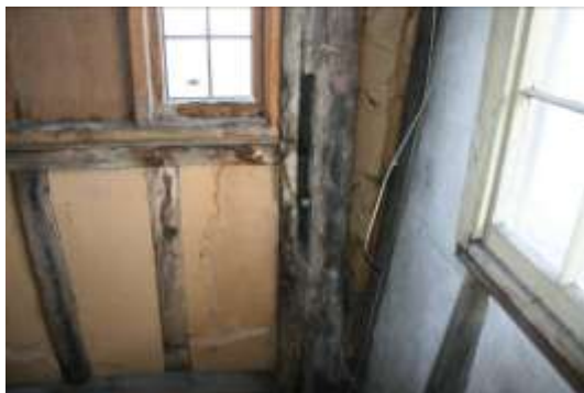
The mortice for the corner brace.
