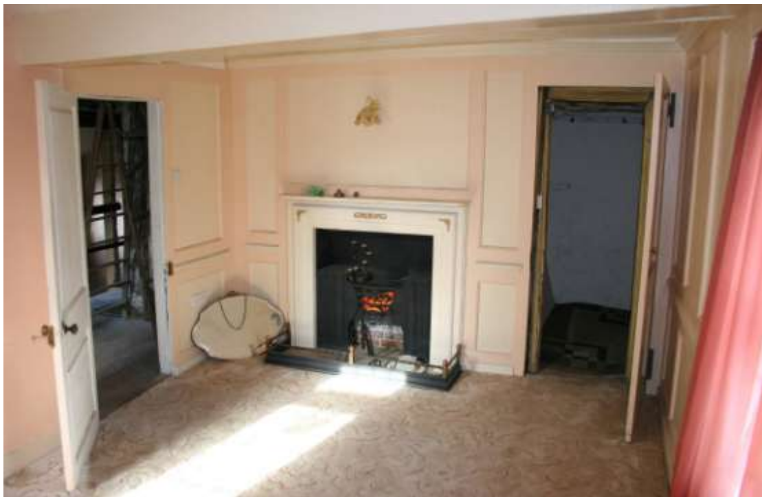
Looking N in Bedroom 2. The hobgrate appears genuine. Note the racked ceiling.
