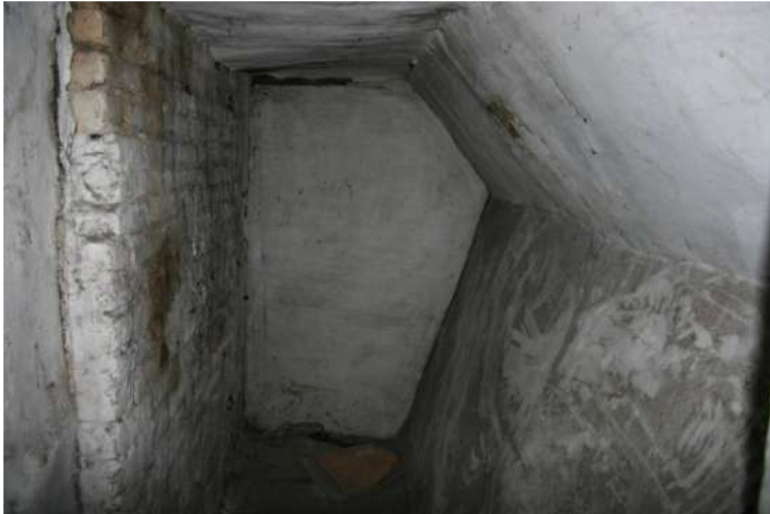
Looking S at the blocked doorway into the South Attic. The brickwork is the firestack.
