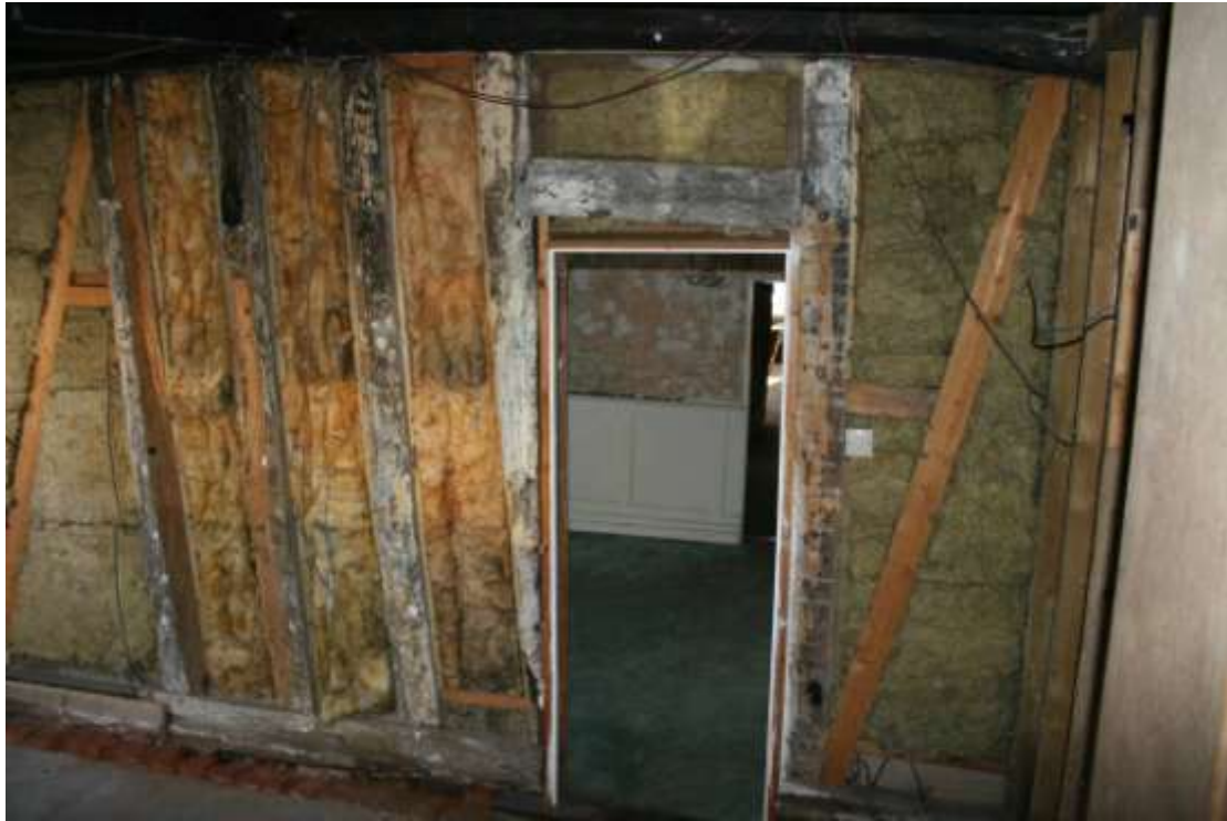
The pegged doorway looking into Room 3. Note the tapered door jamb.
