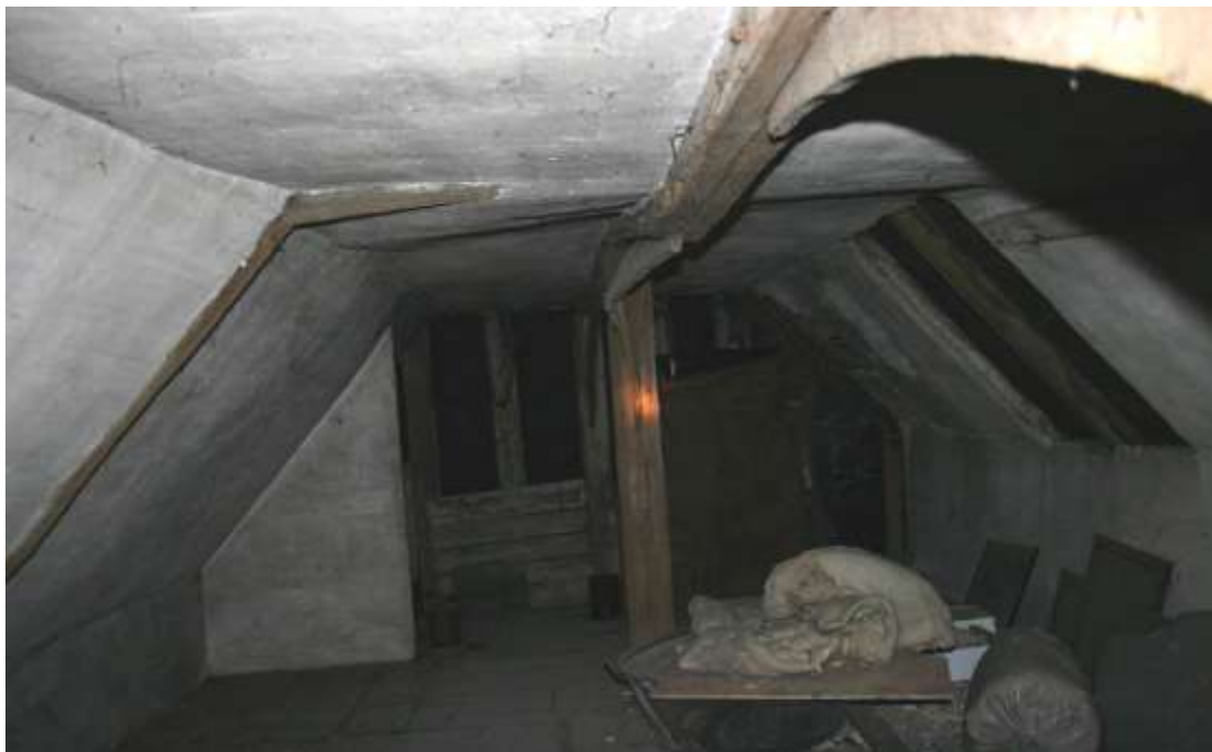
Looking N in the North Attic. Note the framing for a dormer window.
