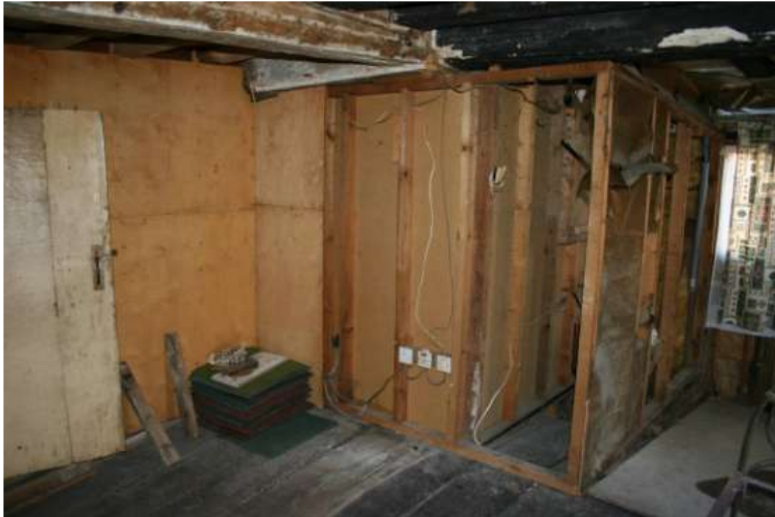
The axial beam and floorboards have mortices for earlier partition wall.
