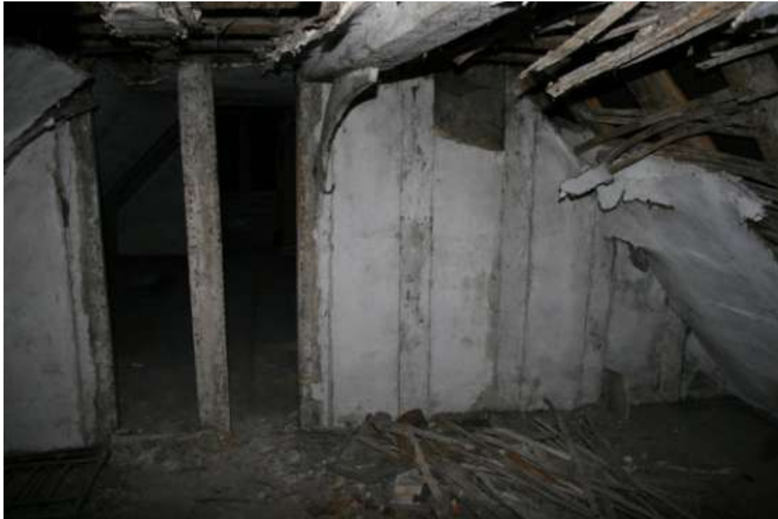
Looking N in the Central Attic. The lath and plaster has failed due to rusty nails.
