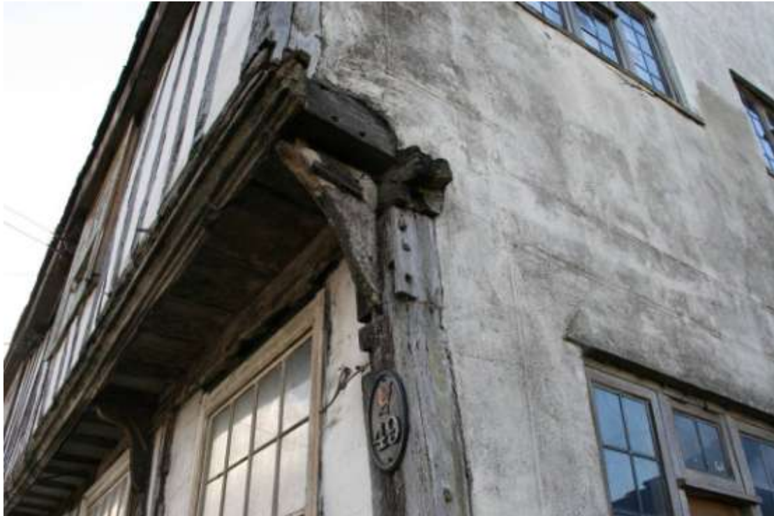
Detail of the bressummer and jetty brackets on the NE corner.
