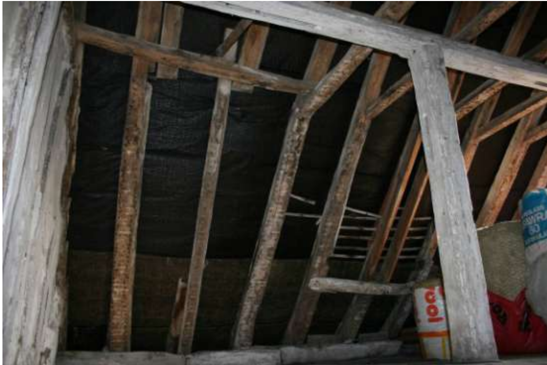
Looking SE at the roof structure in the South Attic. Note the trimmer beam for a window.
