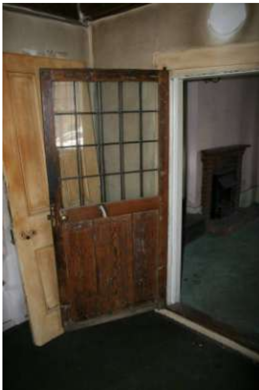
Pine doors altered in the LC20th and screwed in place. Room 2/3 and then Room 3/4.
