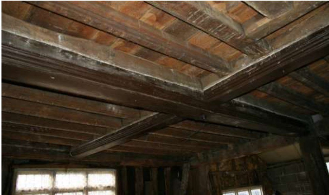
Looking S from the firestack at the sumptuously moulded ceiling.
