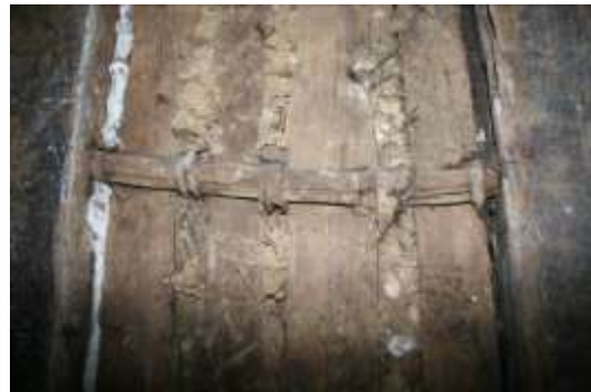
Looking NE in Bedroom 3. The walls retain their wattle and daub.
