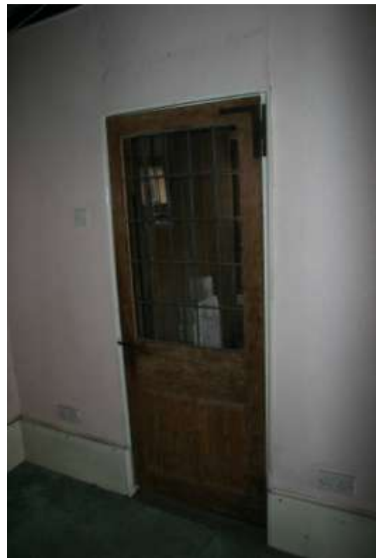
Pine doors altered in the LC20th and screwed in place. Room 2/3 and then Room 3/4.
