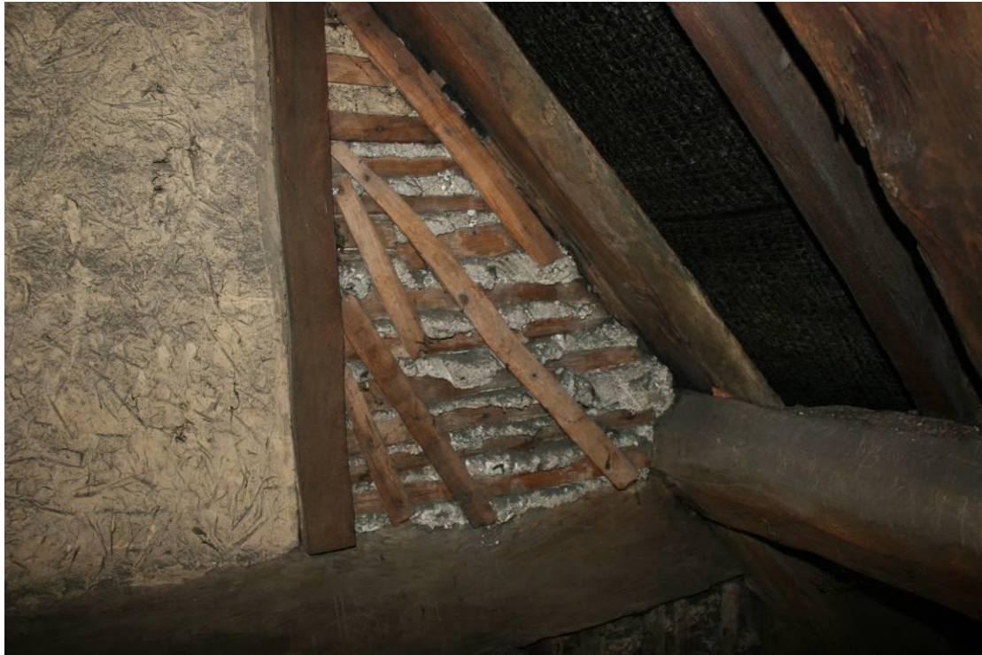
Detail of the lath and daub partitions.
