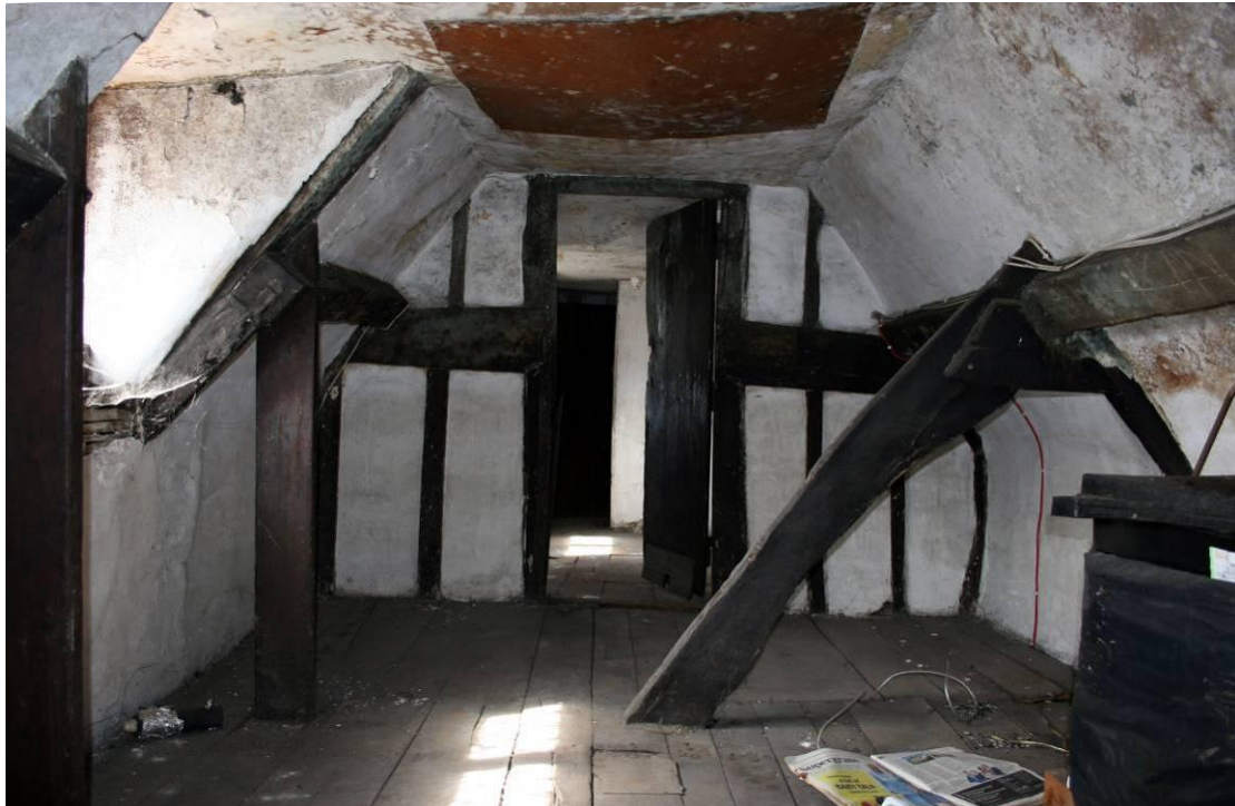
Looking W in Attic Room 2. The collar has been dropped and reused.
