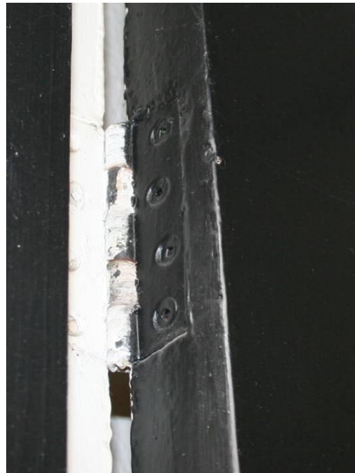
The Victorian door into the Dining Room. The hinges have Robertson screws.
