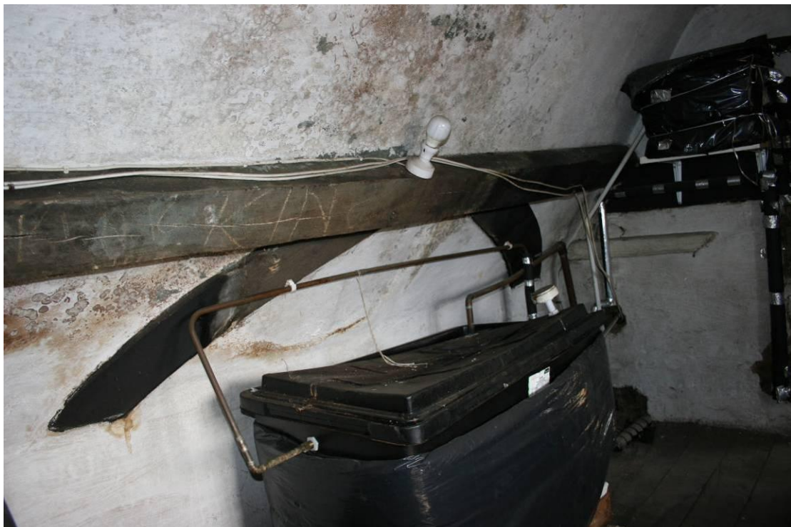
Curved windbraces on the northern side of the frame.
