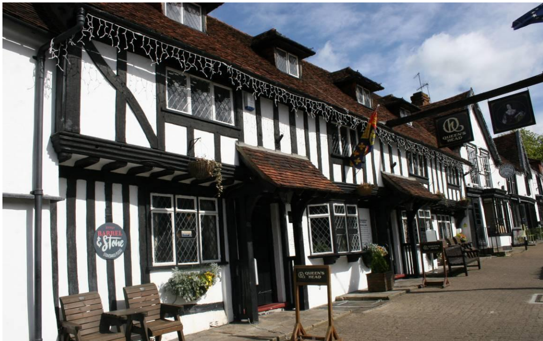
The oblique view shows the long wall jetty construction.
