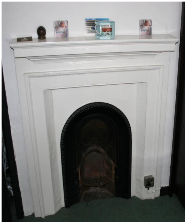
The timber fire surround and detail of the register grate.
