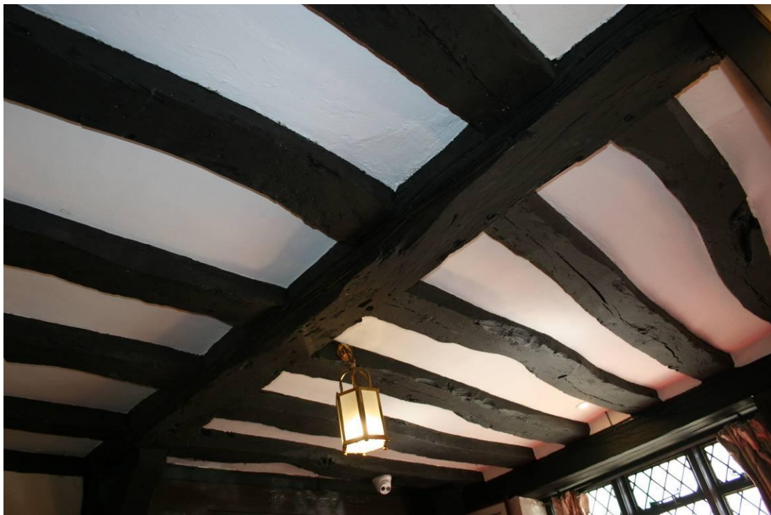
Detail of the wane flat joists in the Bay 4.
