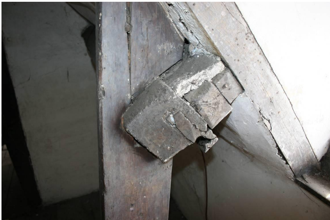
Detail of the sawn through side purlin. The vertical plate was the collar.
