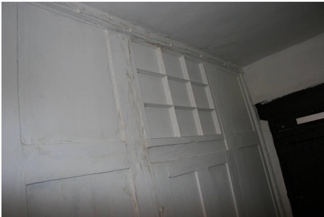
Detail of the reused casement window used to borrow light for the corridor.
