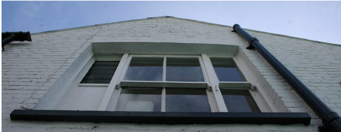
MC19th horned sash windows in the Brick Range.
