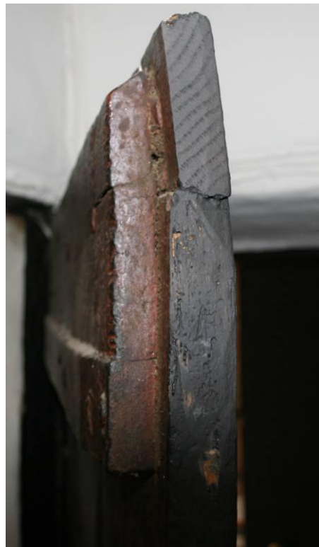
Extension pieces nailed to the door.
