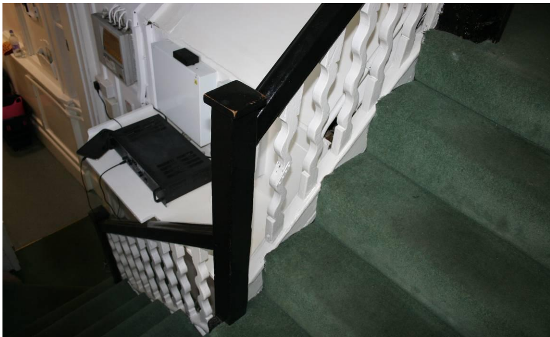
Detail of the splat balusters.
