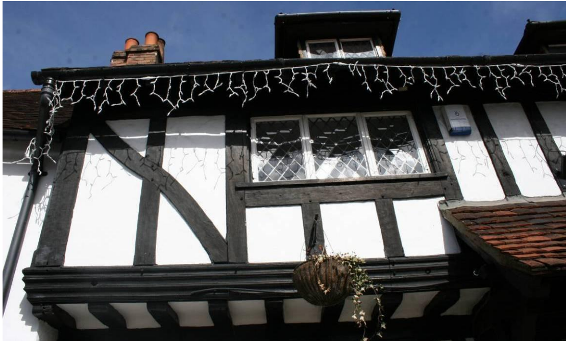
Detail of the jetty. The joists are original but have undergone rebuilding.
