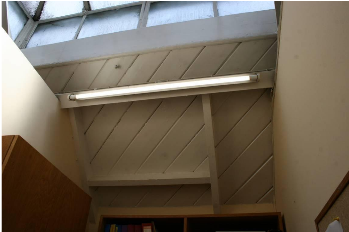
Detail of the boarded roof and skylight.
