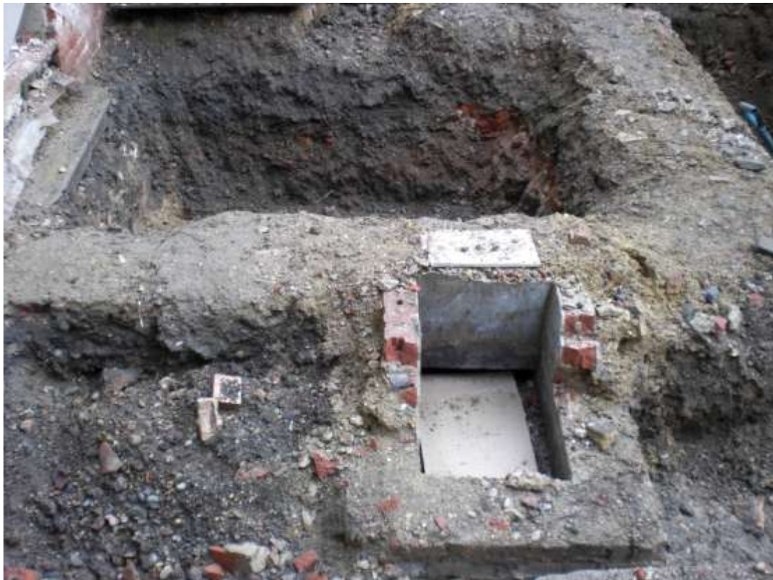
Brick and concrete foul water inspection chamber shown partly demolished.
