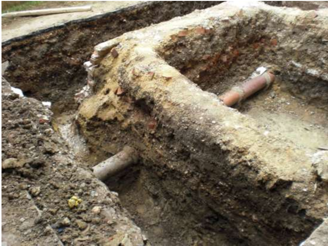
Foundation trenches revealed disturbed drainage trench with ceramic pipe.
