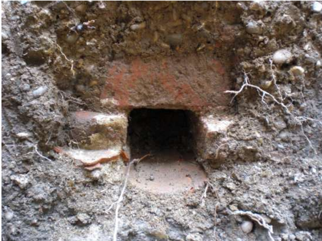
Victorian brick drain discovered in the western section of the excavation.
