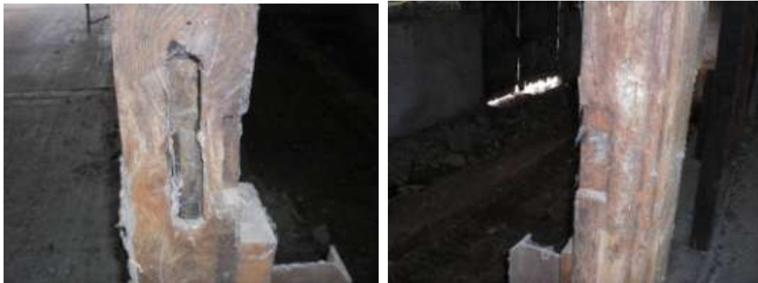
C19th bottle trapped inside the empty mortice (left) and the housing for a door bolt.
