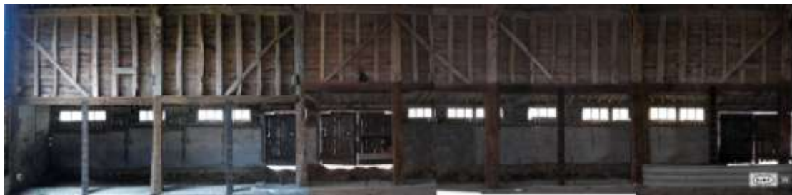
Composite photograph of the south side showing the raised midrails in darker coloured timber.
