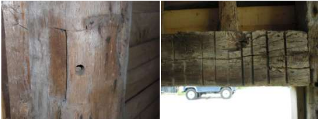
Storey post with pegged birdsmouth and oak beam reduced in section by sawing down.
