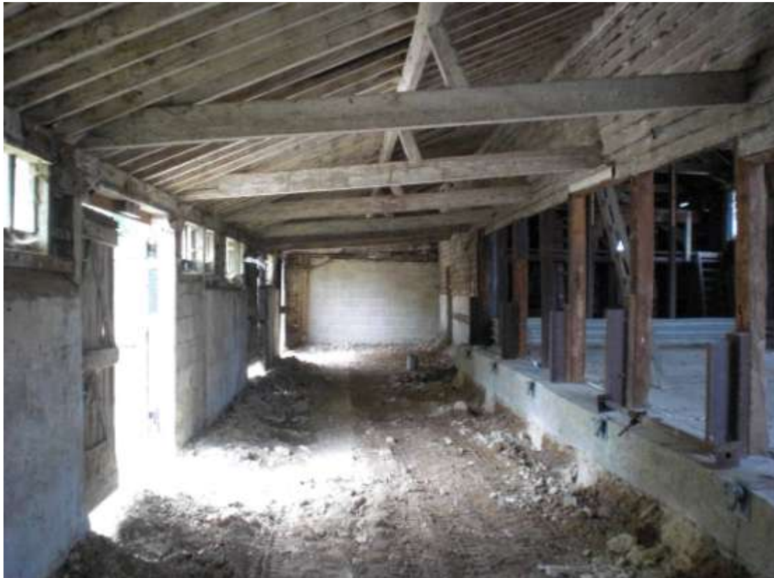
Roof structure of the Outshot looking west. Tie-beams support the simple purlin roof.
