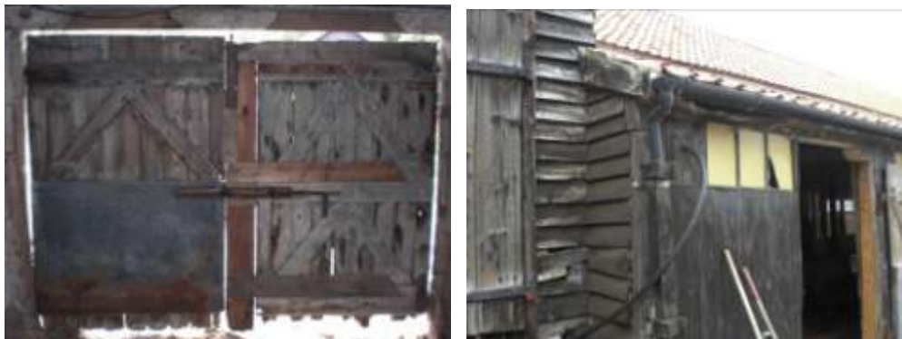
Reused doors and plastic C20th guttering with square downpipes on the SW corner of the Outshot.
