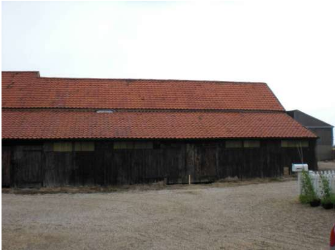
The southern elevation comprises an Outshot with vertically panelled walls.
