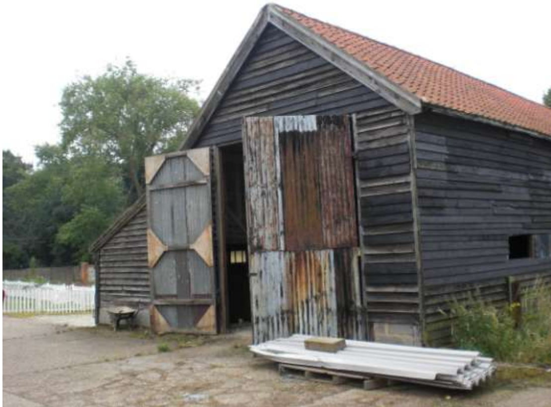
Eastern elevation showing the C20th homemade doors. The cladding on the pallet lined the interior.
