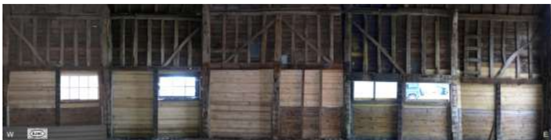
Composite photograph of the north side showing the raised midrail in the midstrete (Bay 3).
