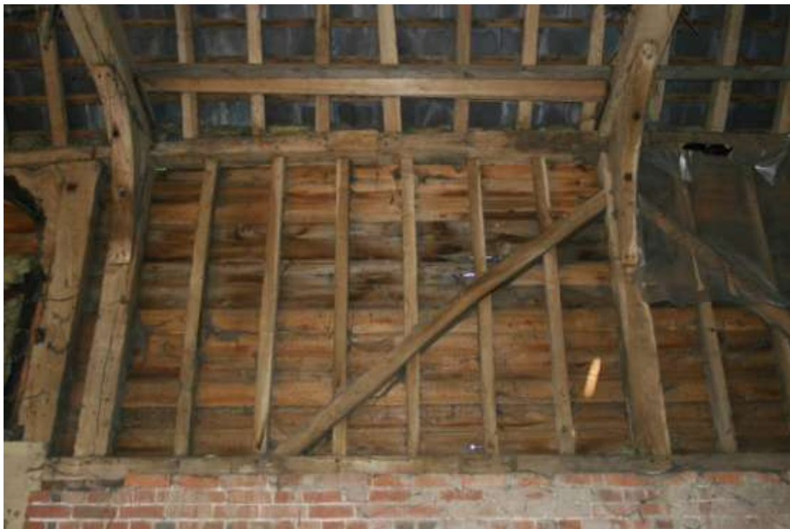
The wall panel in Bay 5 (north side) typifies the construction of the timber frame.
