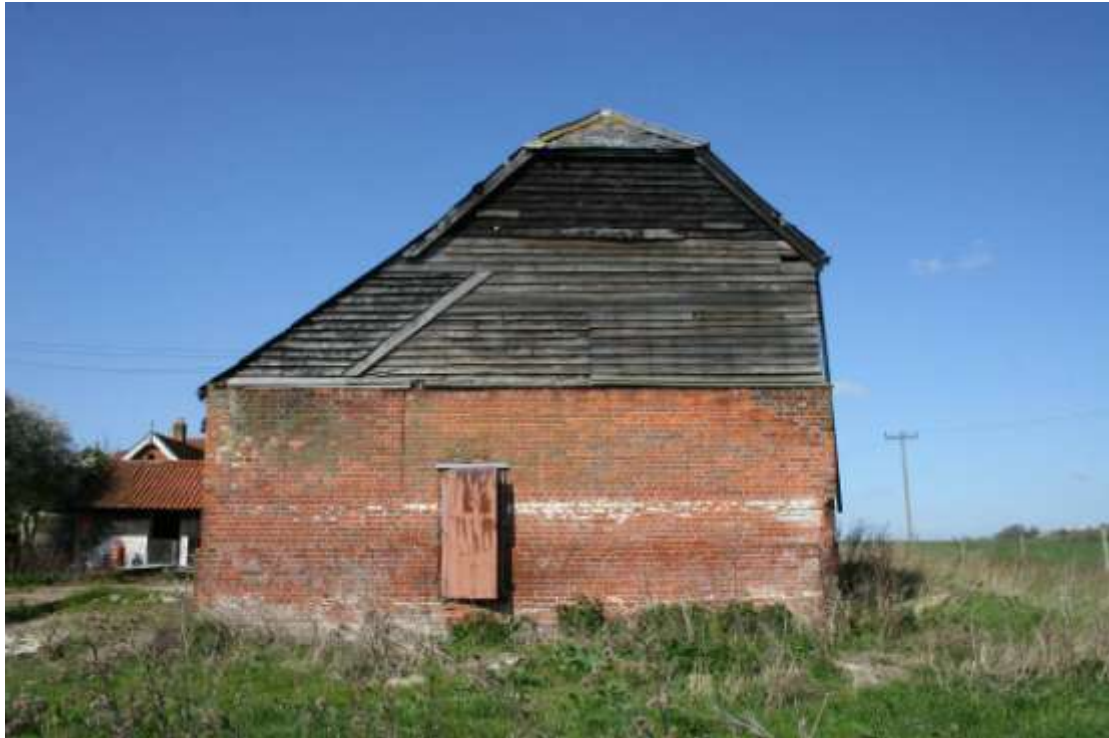
The eastern elevation shows several episodes of weatherboarding.
