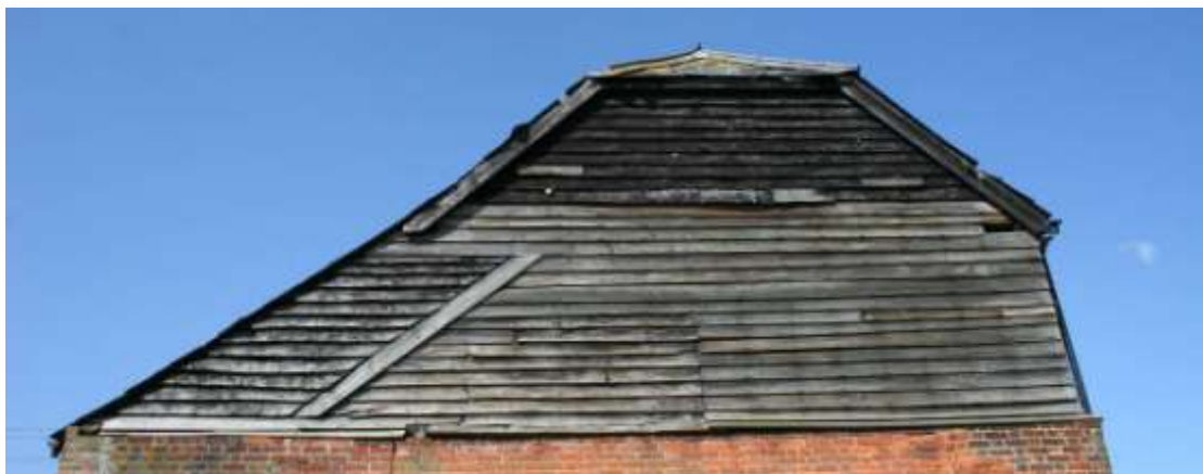
The weatherboarding is in three distinct sections with local repairs.
