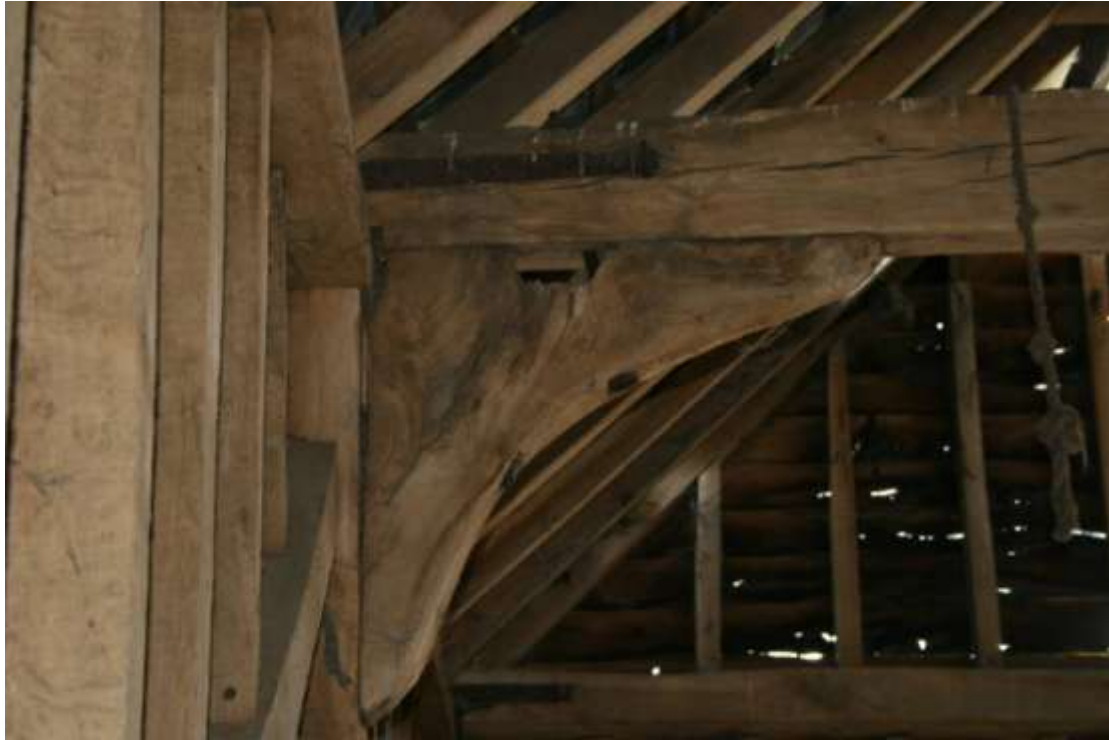
Hanging knee fastened with screw-threaded bolts.
