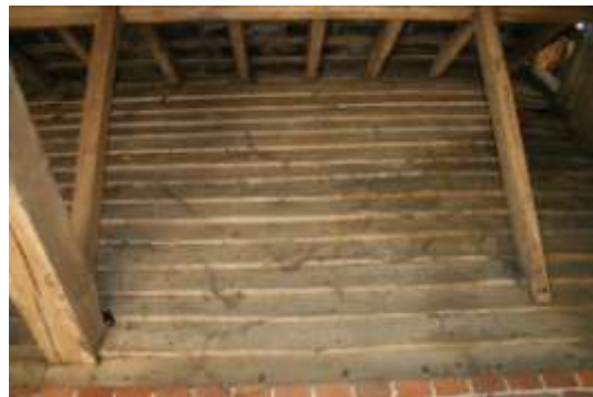
The weatherboarding above the Western Outshut is clean and untarred.
