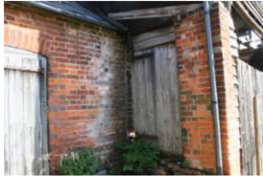
Failing eastern flank of the porch and (right) the side entrance to the porch.
