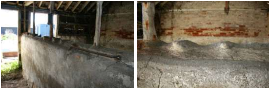
Worn down timber rail in Pen 3. There is a sliding tether rail near the middle.
