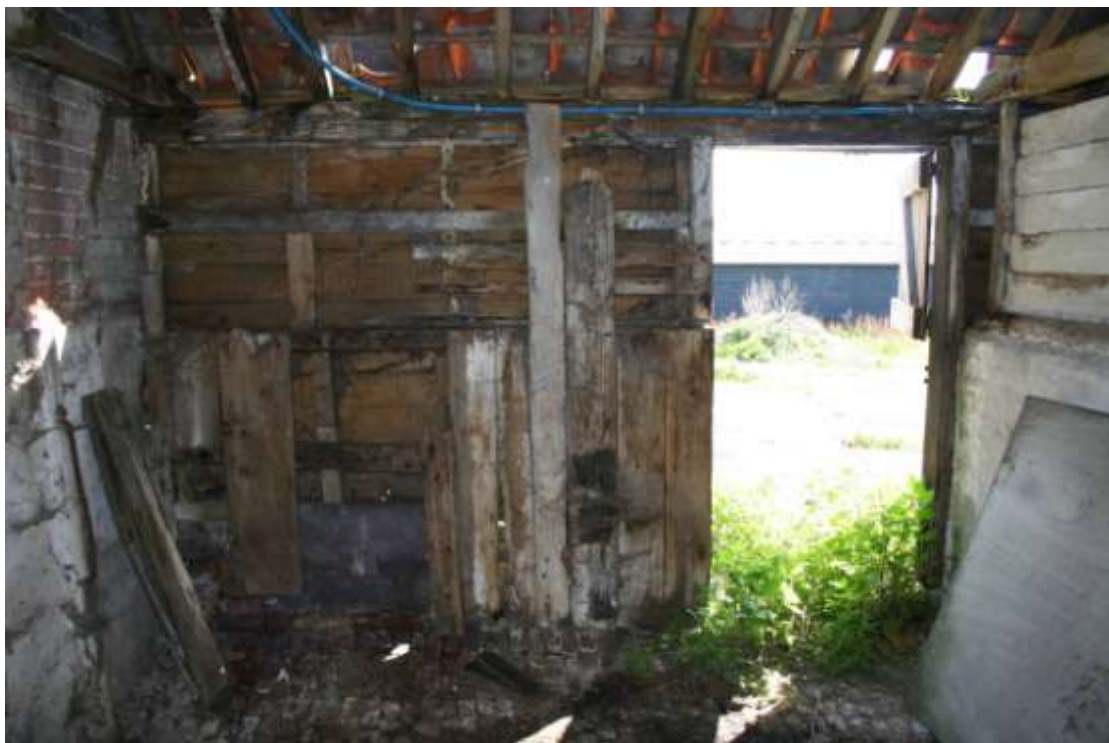
Interior of Pen 1. Vertical boards and thick slate tiles. Note sliding tether bar to left.
