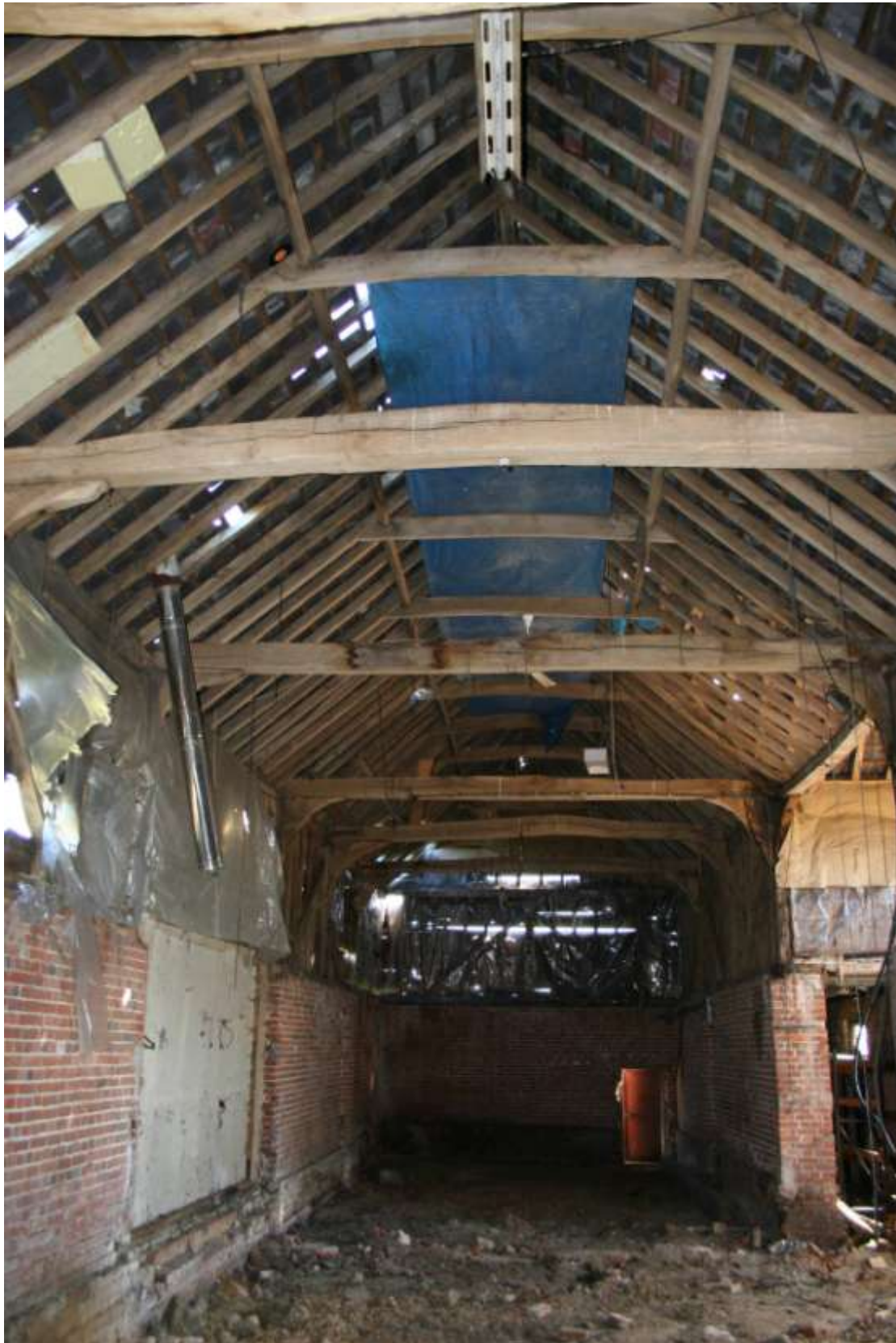
Simple clasped side purlin roof. See also the architect's section drawing.
