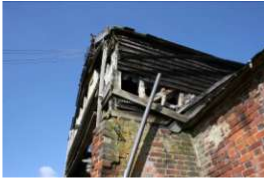
Failing eastern flank of the porch and (right) the side entrance to the porch.
