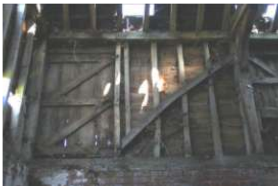
Inserted door in the NW corner of Bay 1.
