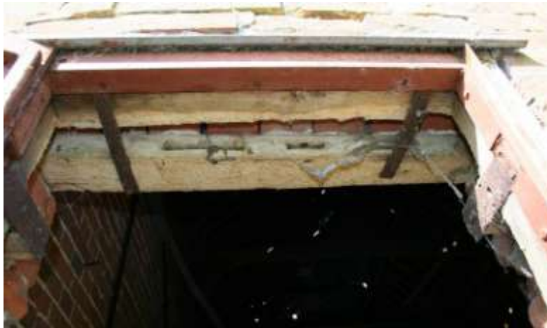
Detail of the inserted door into the eastern elevation.
