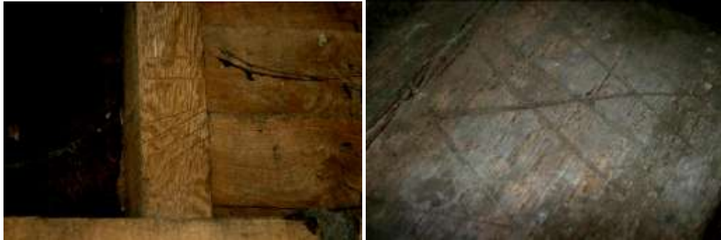
Carpentry marks on the stud (left) and on the sill plate. Contrast boosted for clarity.
