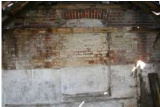
Bricked in doorway visible in the Stables. Mortar is markedly different.
