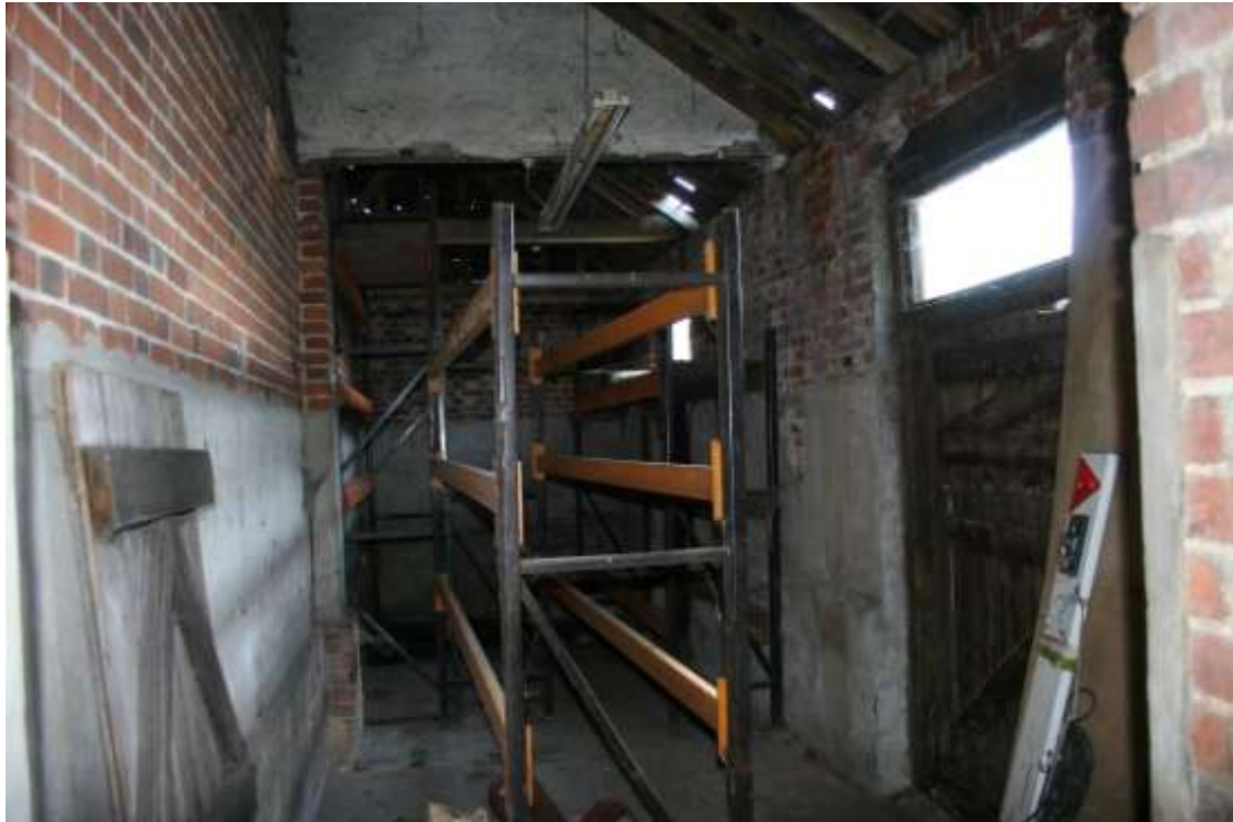
Looking into the Eastern Outshut. Lath and plaster division still in-situ above.
