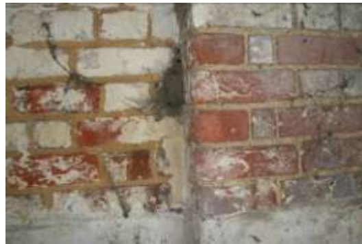
Bricked in doorway visible in the Stables. Mortar is markedly different.
