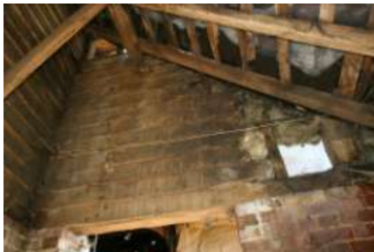
The weatherboarding above the Western Outshut is clean and untarred.
