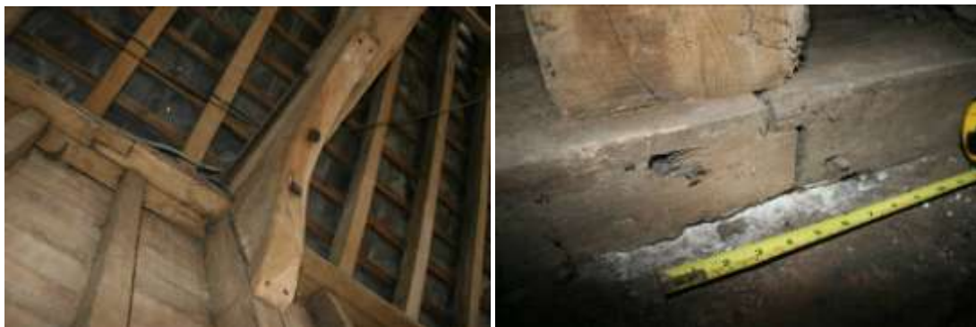
Scarf joints in the top-plate (left) and the sole plate.
