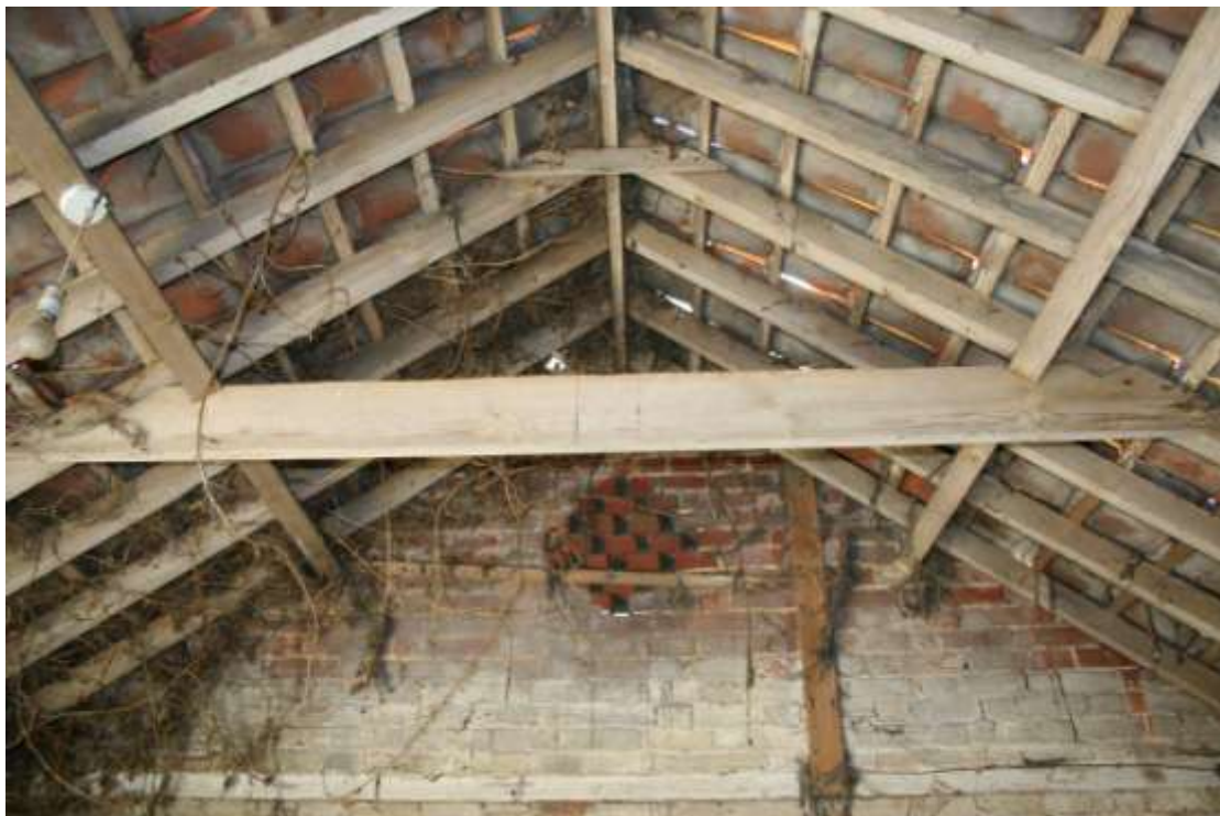
The roof is made of machine sawn softwood.
