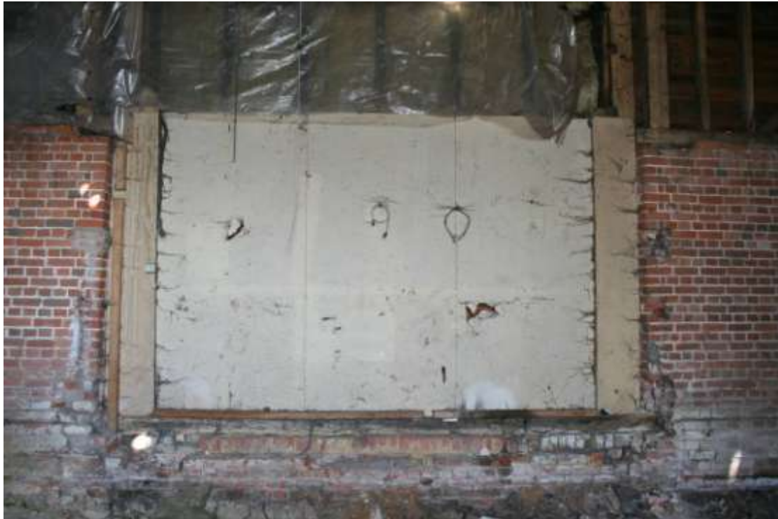
Walls scars in the door jambs show where two dividing walls crossed the barn.
