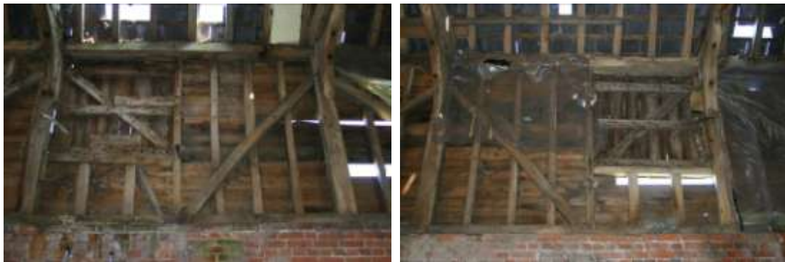
The two loft doors are fully framed and original to the build.
