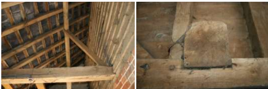
Roof structure of the Western Outshut and the end of a tie-beam visible inside the Barn
