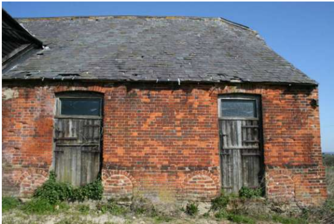
Southern elevation of the Eastern Outshut. Note semi-circular tunnels.
