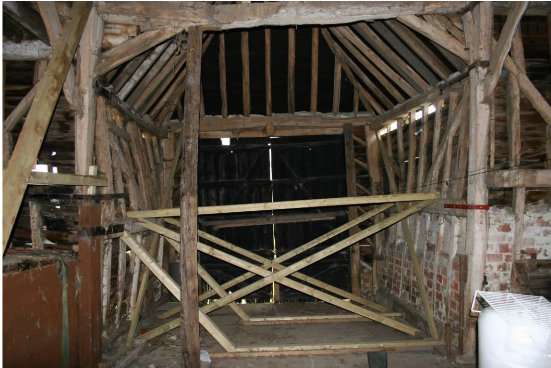
Internal struts and props to stabilise the raked midstrey.
