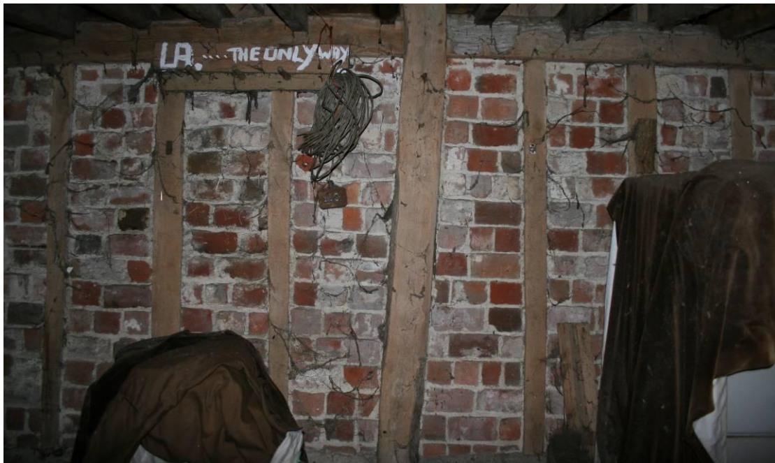
Brick noggin still in-situ in the SE wall.
