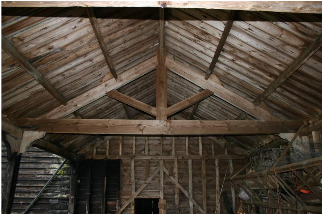
Pre-fabricated machined truss with central king strut. Looking west.
