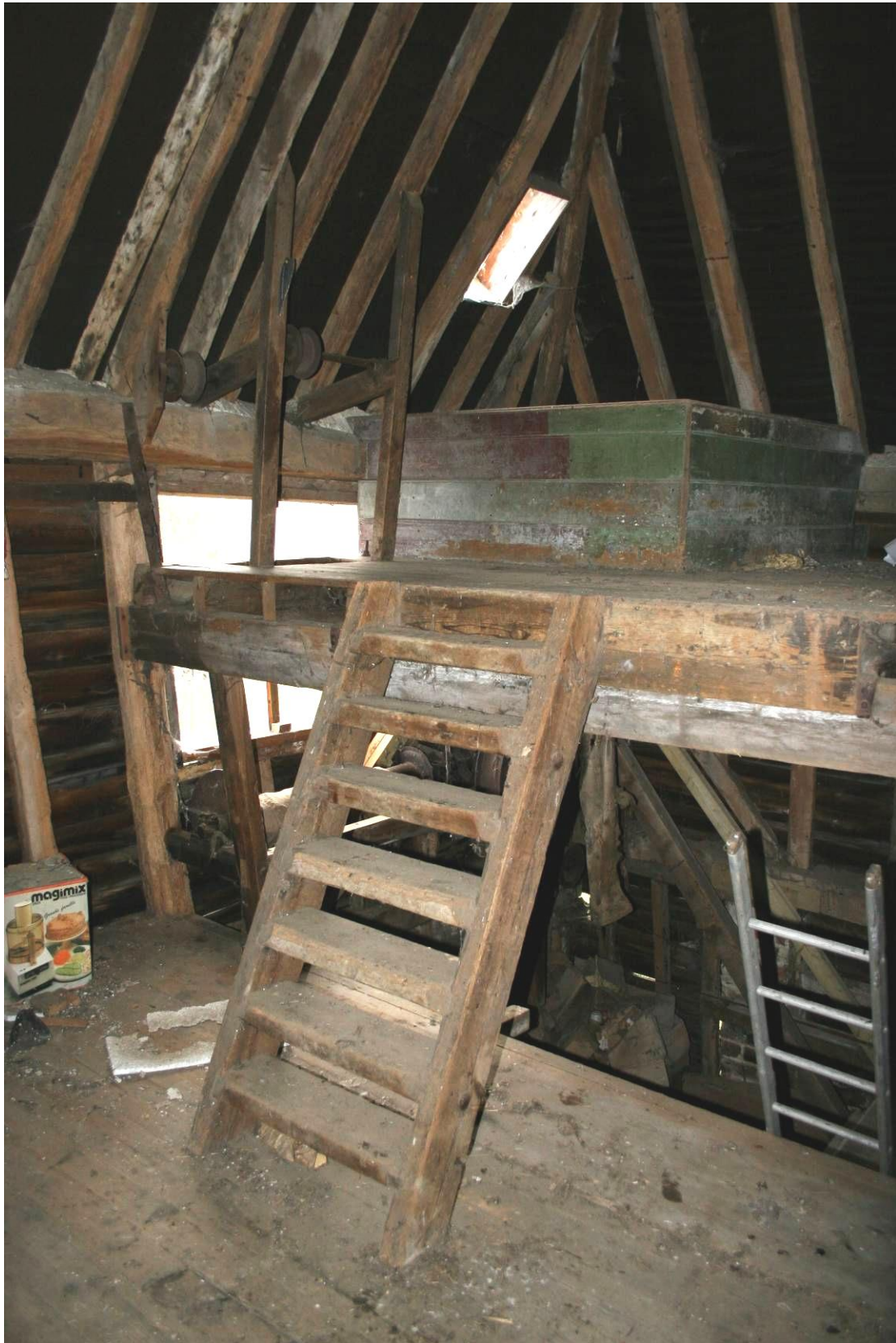
Grain hopper on the top floor. Connecting ladder between the two floors. Machinery behind. Looking SW.
