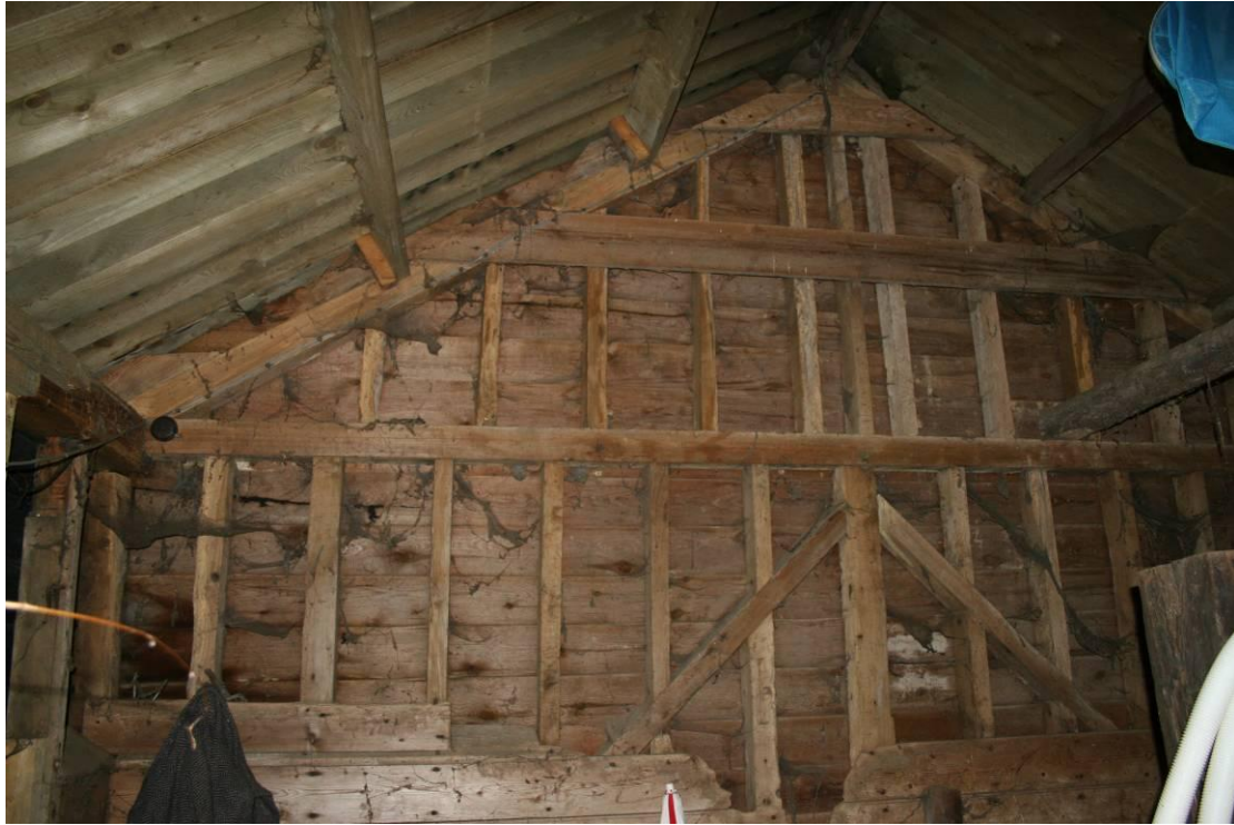
Western wall with primary bracing and interrupted studwork.
