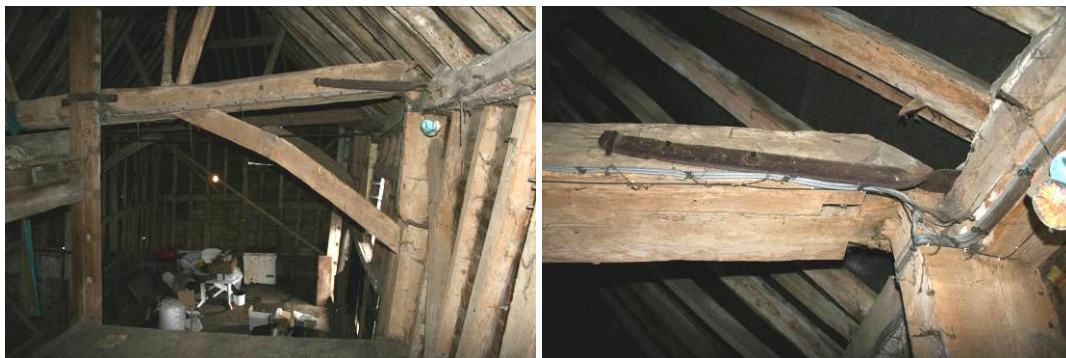
Eastern side of the southernmost truss. Underside shows misplaced teasel mortice.
