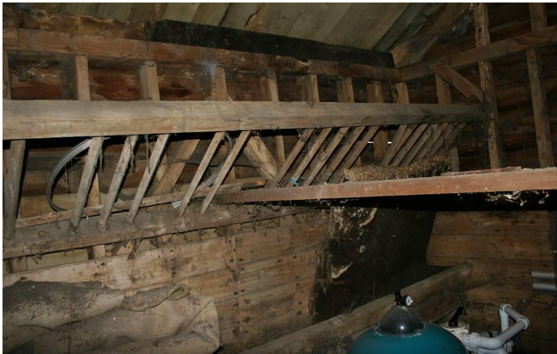
Hay rack and manger running along the north wall.
