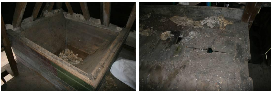
Grain hopper on the top floor and trap door for chain hoist run on pulleys above.
