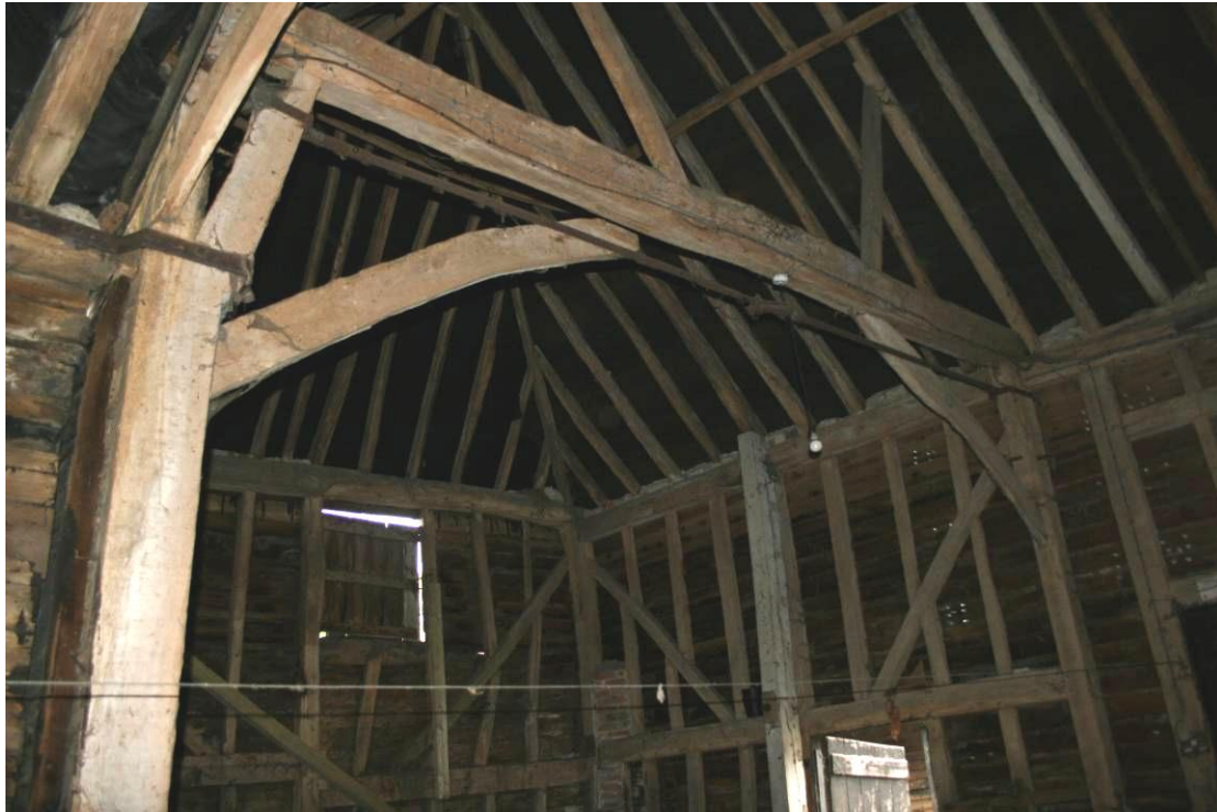
The northernmost truss has failed at both jowls and been reinforced with steel tie-rod.
