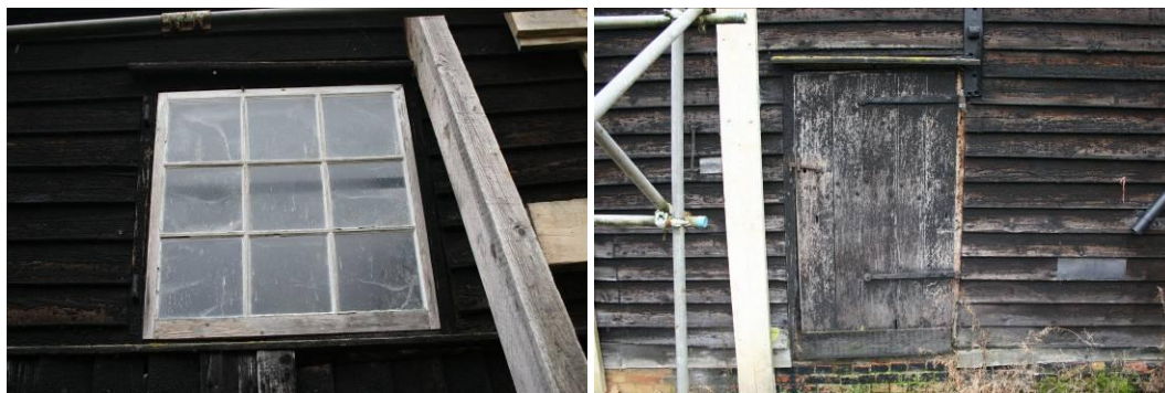
Re-used sash window above the central doors and pedestrian side door.
