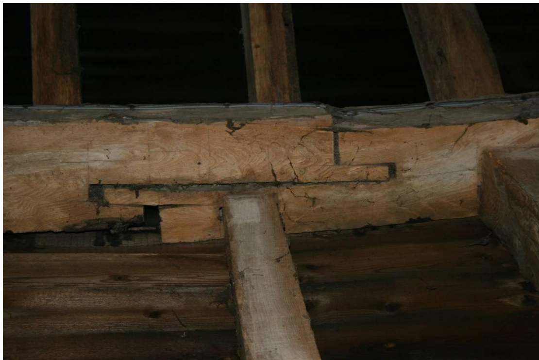
Scarf joint in the NW wall top-plate.
