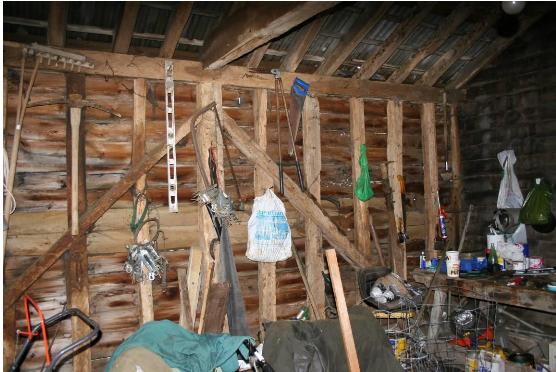
Northern wall of the workshop. Note tie-beam above.
