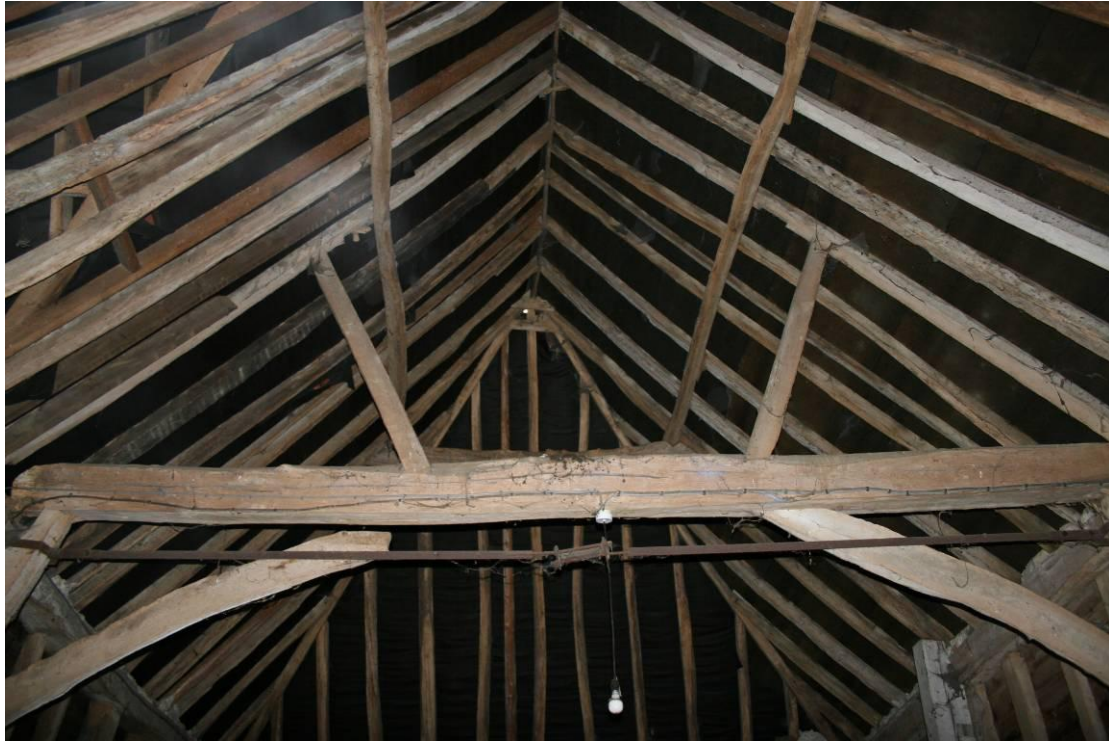
Collar side purlins and queen strut roof structure. Northern truss collar is missing. Looking N.
