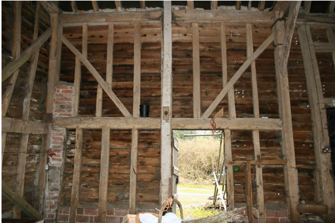
NE interior wall showing the offset studs and inserted pedestrian door.
