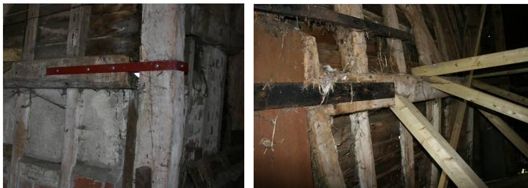
C21st repairs to the midstreys. North side (left) and south side (right).
