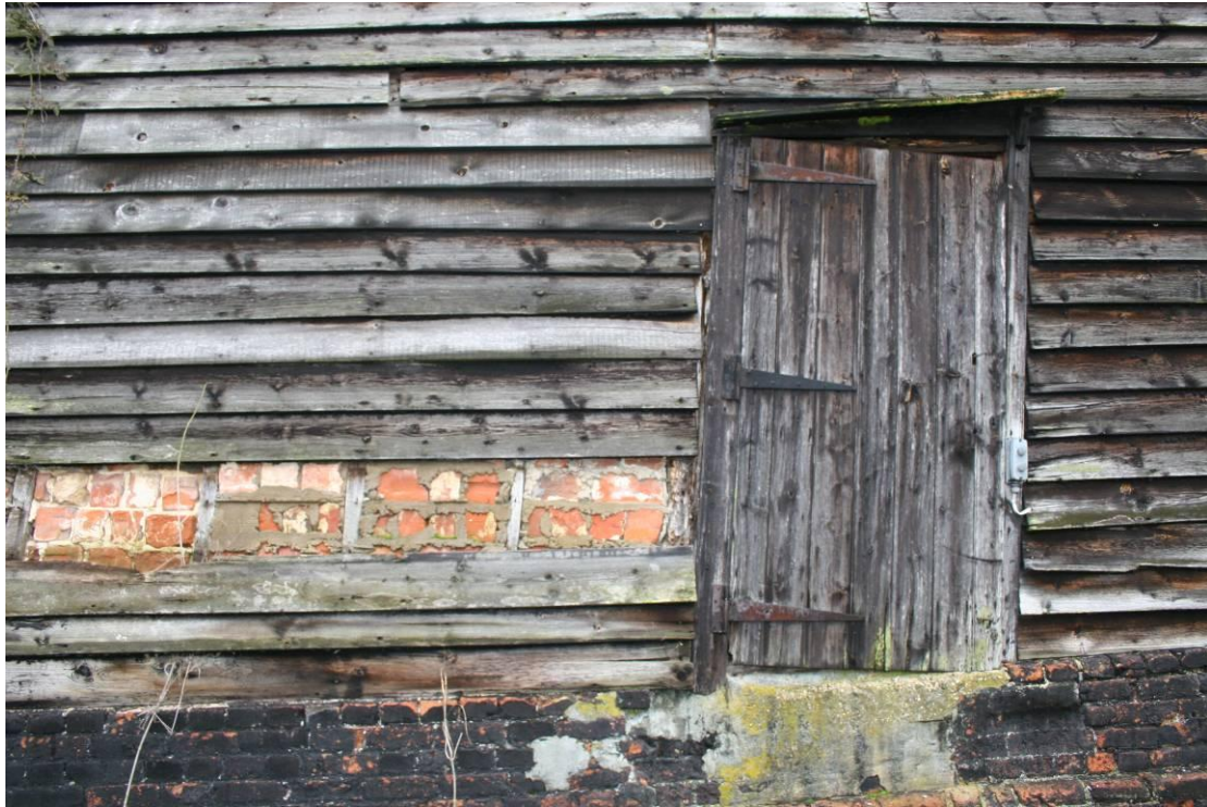
The inserted C20th door and the exposed brick noggin and plinth.
