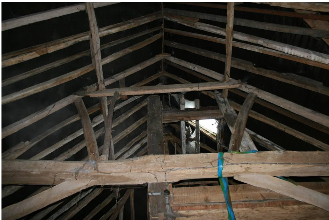
Southern truss with curved queen struts and collar in place. Looking south.
