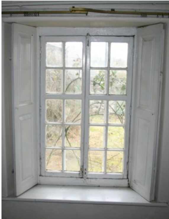
Plate 28. Early Side Hung Casement Window
