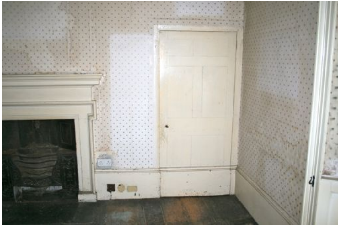
Plate 16. Dressing Room Door Showing Flush Arrangement and Skirting
