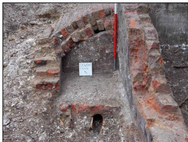
Plate 8: Vaulting and inlet pipe (0.5m scale)
