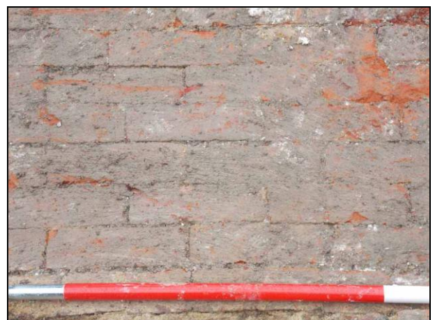
Plate 6: Vaulted roof brickwork (0.5m scale)
