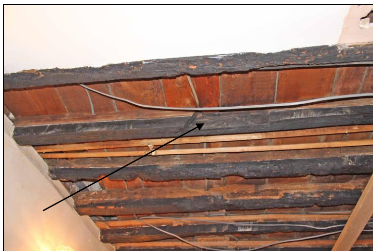
Plate 2: Joist 2 from the south with rafter seating arrowed
