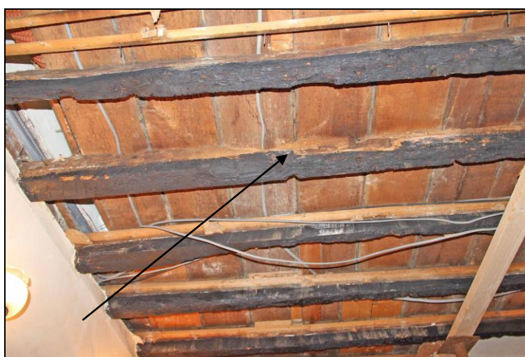
Plate 4: Western end of Joists 3 and 4 from the south. Through mortice on Joist 4 arrowed
