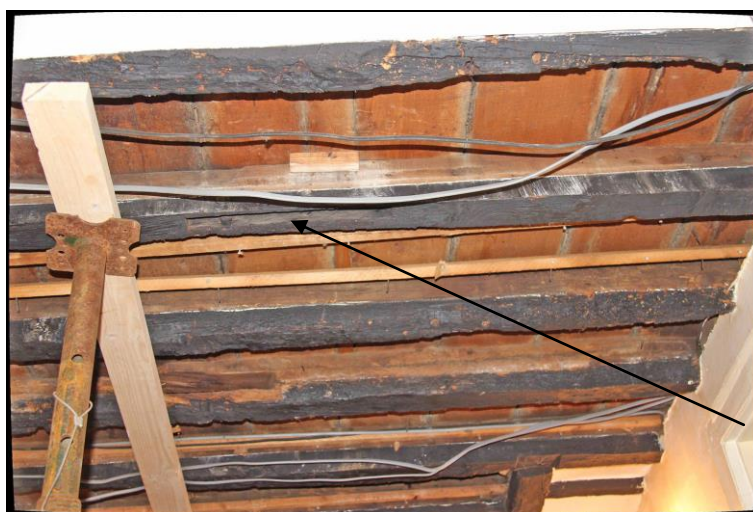
Plate 3: Joist 2 from the south with mortice arrowed
