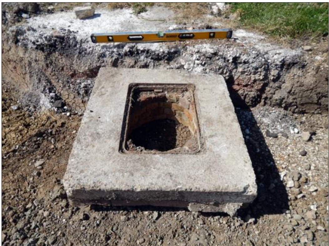
Plate 19: Cover for well, not in situ (1.2m scale)
