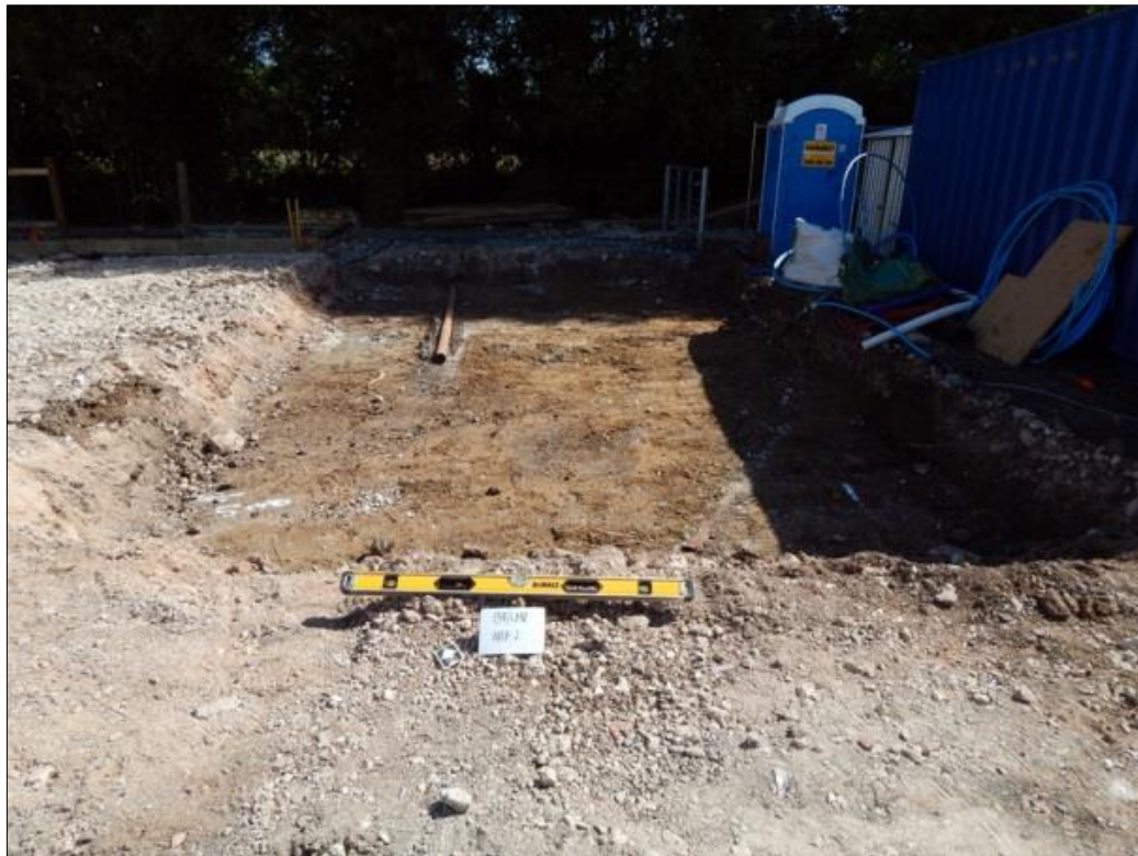
Plate 20: Area 2, facing northeast (1.2m scale)
