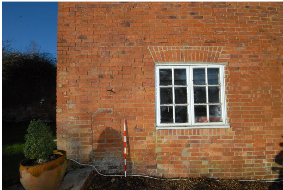
South-west range, detail showing blocked arch
