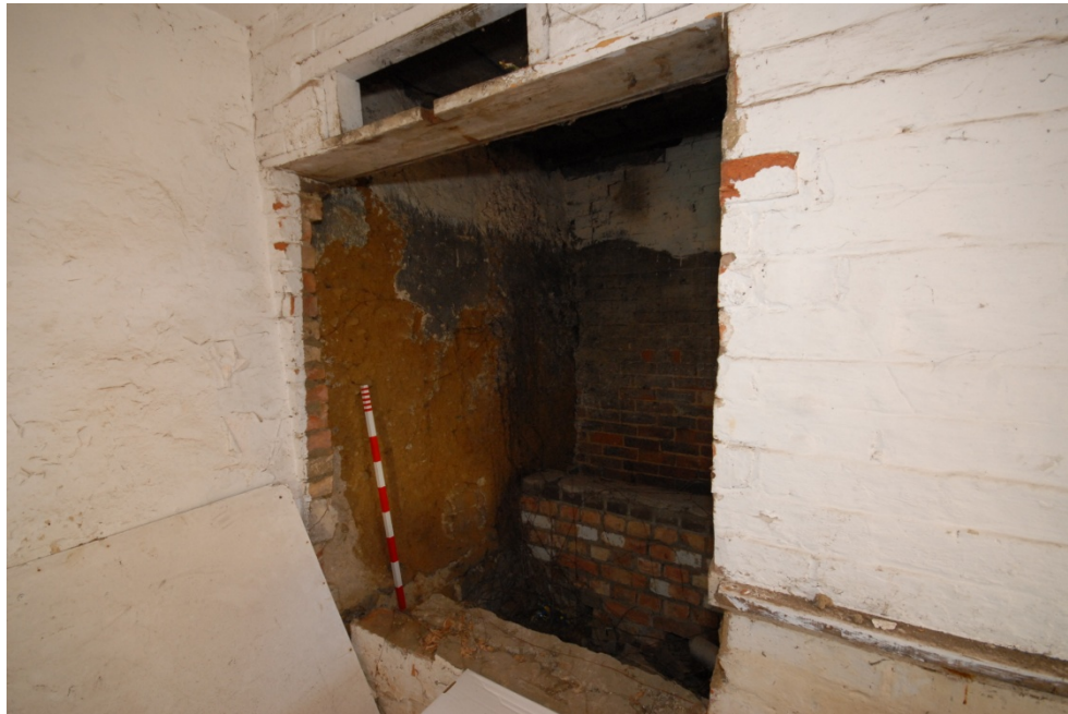
The opening from the former coach room to the possible former fuel store, with the exposed cob wall visible Fig 16
