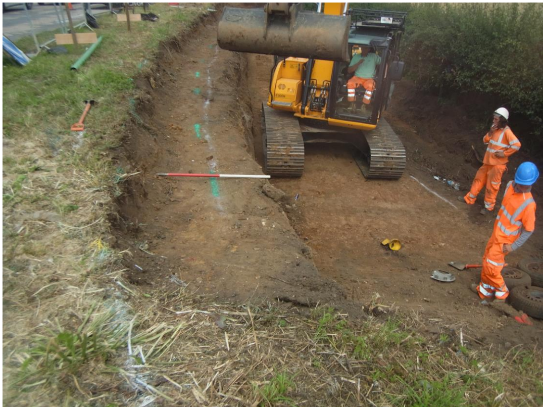
Excavation of the old highway ditch, looking north Fig 9
