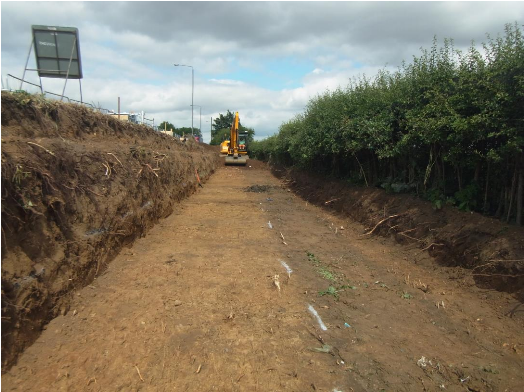
Excavation of the old highway ditch, looking north Fig 8
