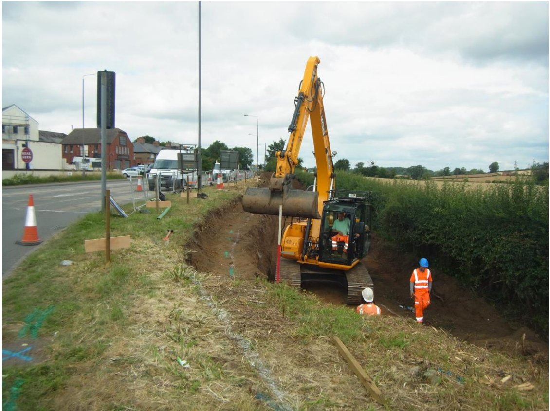
The groundworks in progress, looking north Fig 6
