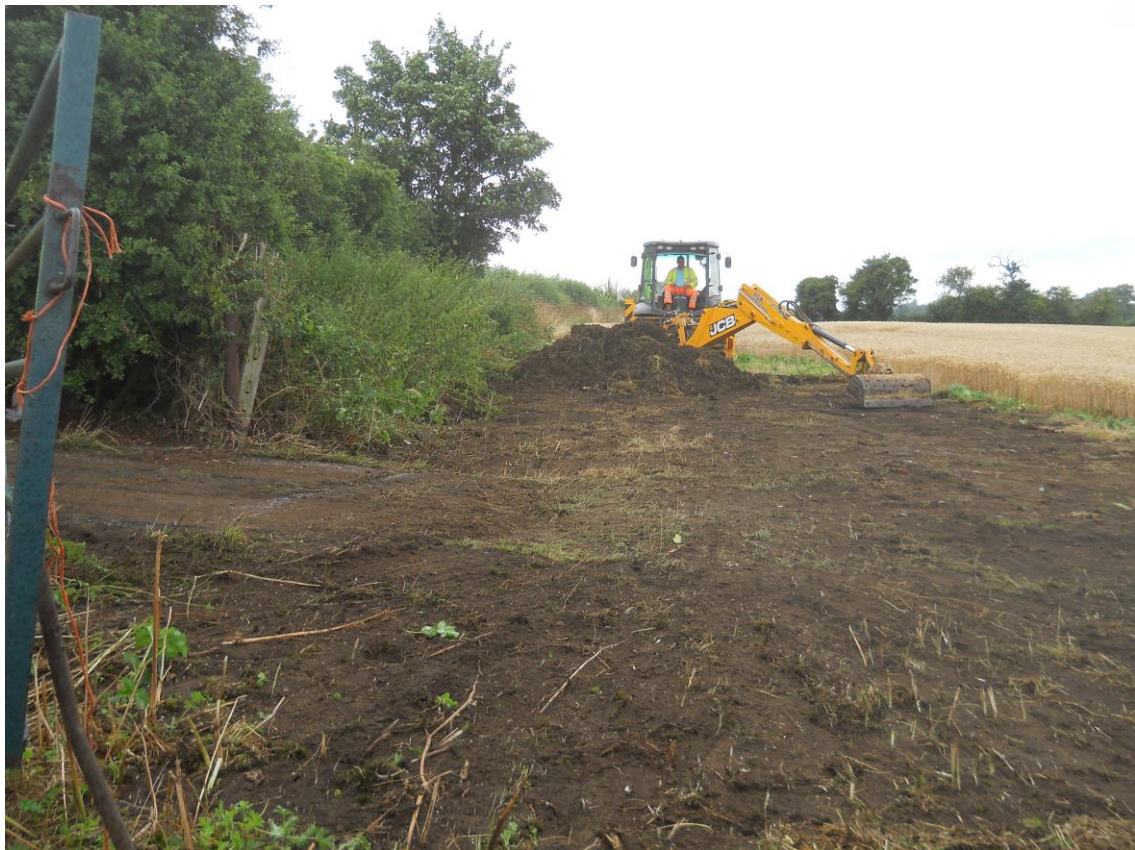
Stripping the area of the new compound, looking north Fig 7
