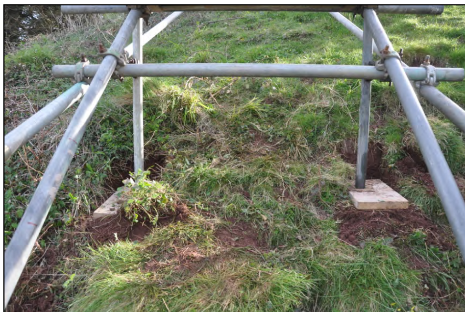
Detail of shallow excavations for the scaffold post pads Fig 16
