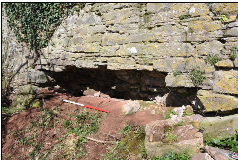
The south curtain wall prior to installation of props Fig 8
