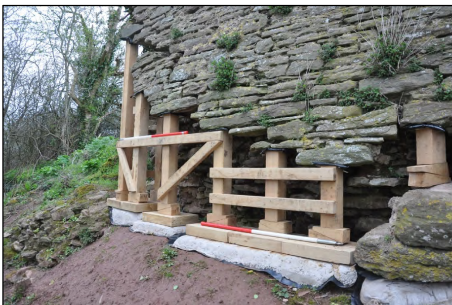
The west edge of the south curtain wall with props installed Fig 11
