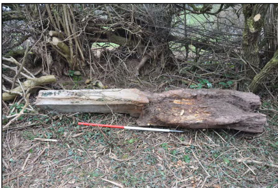
The hanger post, showing the shaped and unshaped portions of the timber Fig 5
