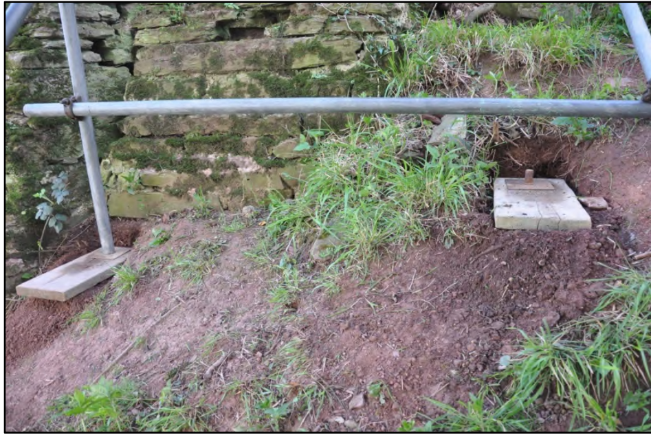
Detail of the scaffold post pads Fig 20
