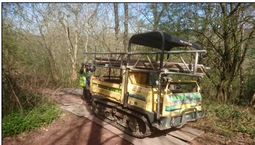
Protection of the access track by wooden boards Fig 7
