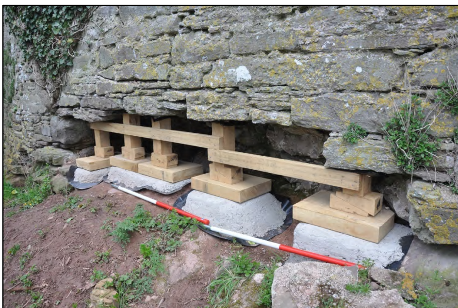
The south curtain wall with props installed Fig 9
