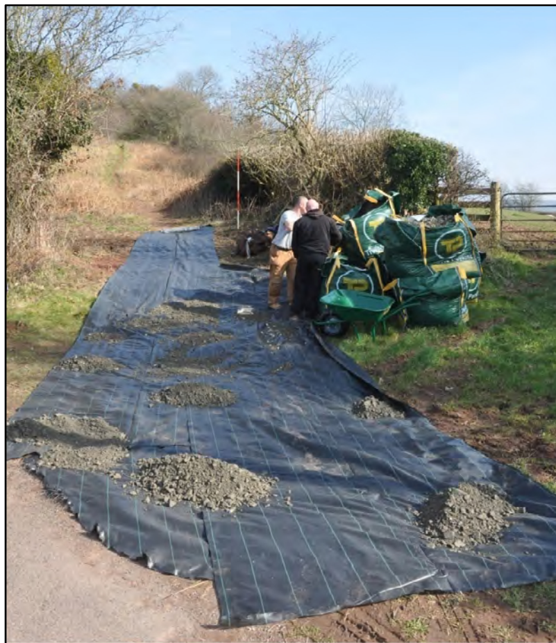
The compound access with protective membrane Fig 6
