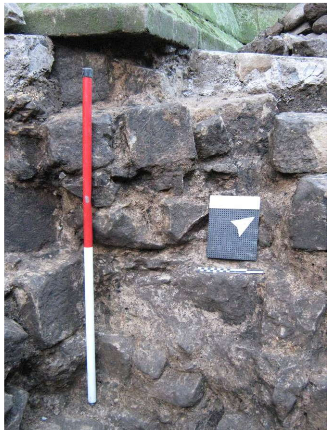
Plate 10. Another detail of the mid-13 th century foundation raft (5005), again showing the gap below the base chamfer where medieval foundation-work was been removed in the 1985 landscaping. Looking west. Scale 1m.
