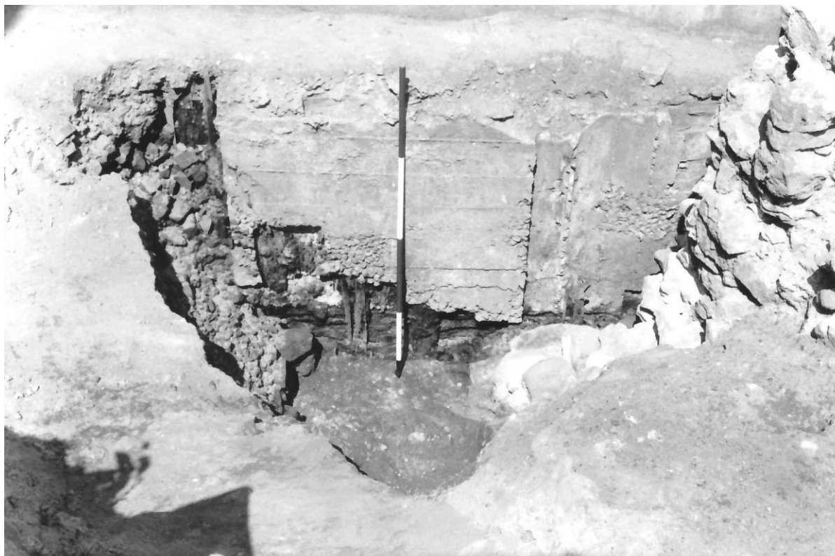
15. Rear wall and offset of the air-raid shelter after removal of part of the construction cut infill, showing offset and remains of shuttering. Wall (734/852) to the right. Scale 2m. (Film 1984/2/32)
