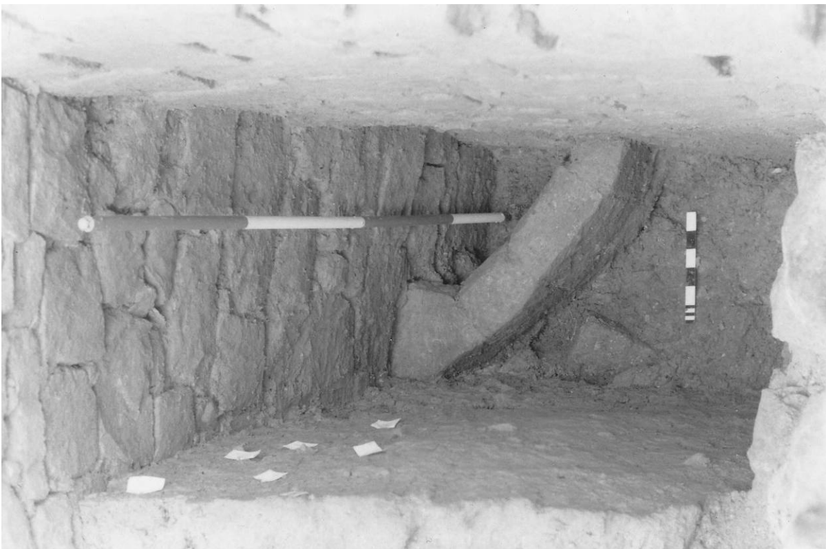
13. Left - Masonry arc (1843) in the south-west angle of 'cess-pit' (1823), looking south. Scales 2m and 0.5m. (Film 1984/5/20A)
