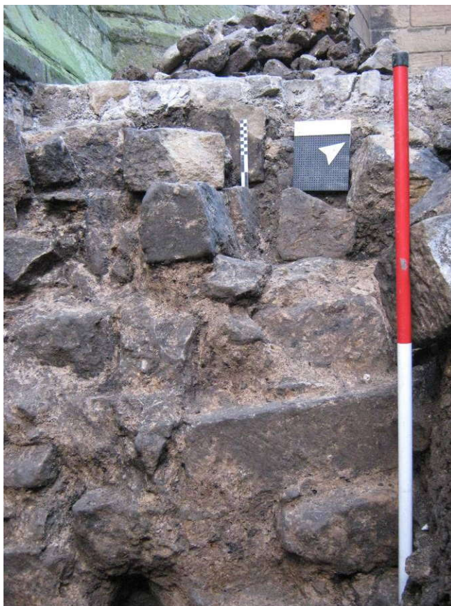
Plate 11. Another detail of the mid-12 th century foundation <5005> to the Black Gate, showing faced ashlars re-used as part of the rubble and mortar raft. Looking west. Scale 1m.
