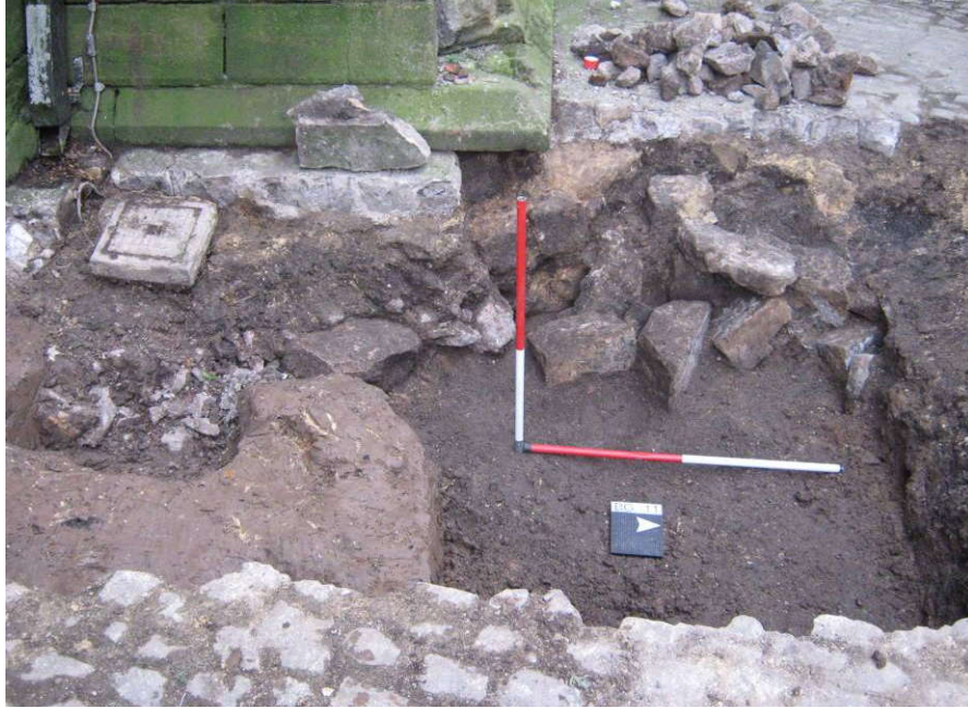
Plate 3. After removal of hard landscaped surface and sub-base, showing glacial till <5006>, lightning conductor <5007>, soil and rubble backfill and disturbed foundation stones from the Black Gate foundation raft. Looking west. Scales 1m.
