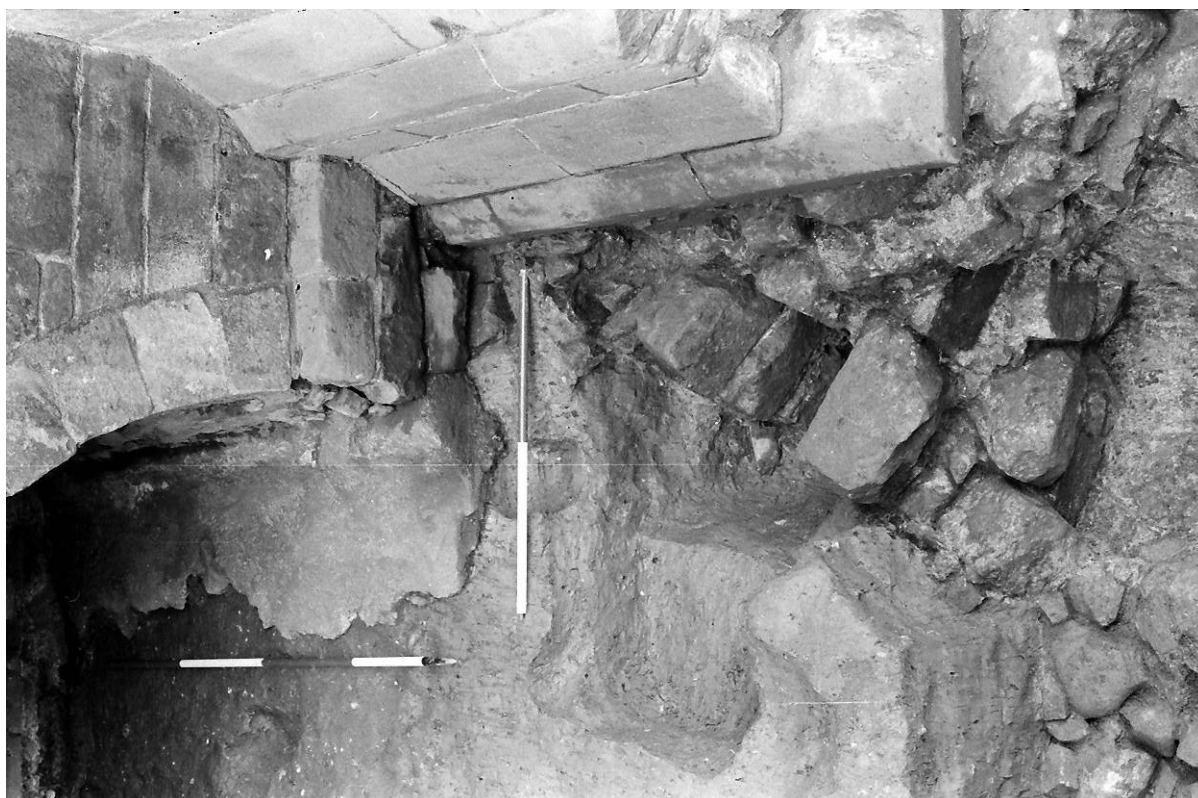
5. Left - Junction of wall (1825) and the Black Gate <5008> showing foundation raft of the latter <5005> (Film 1984/3/37)
