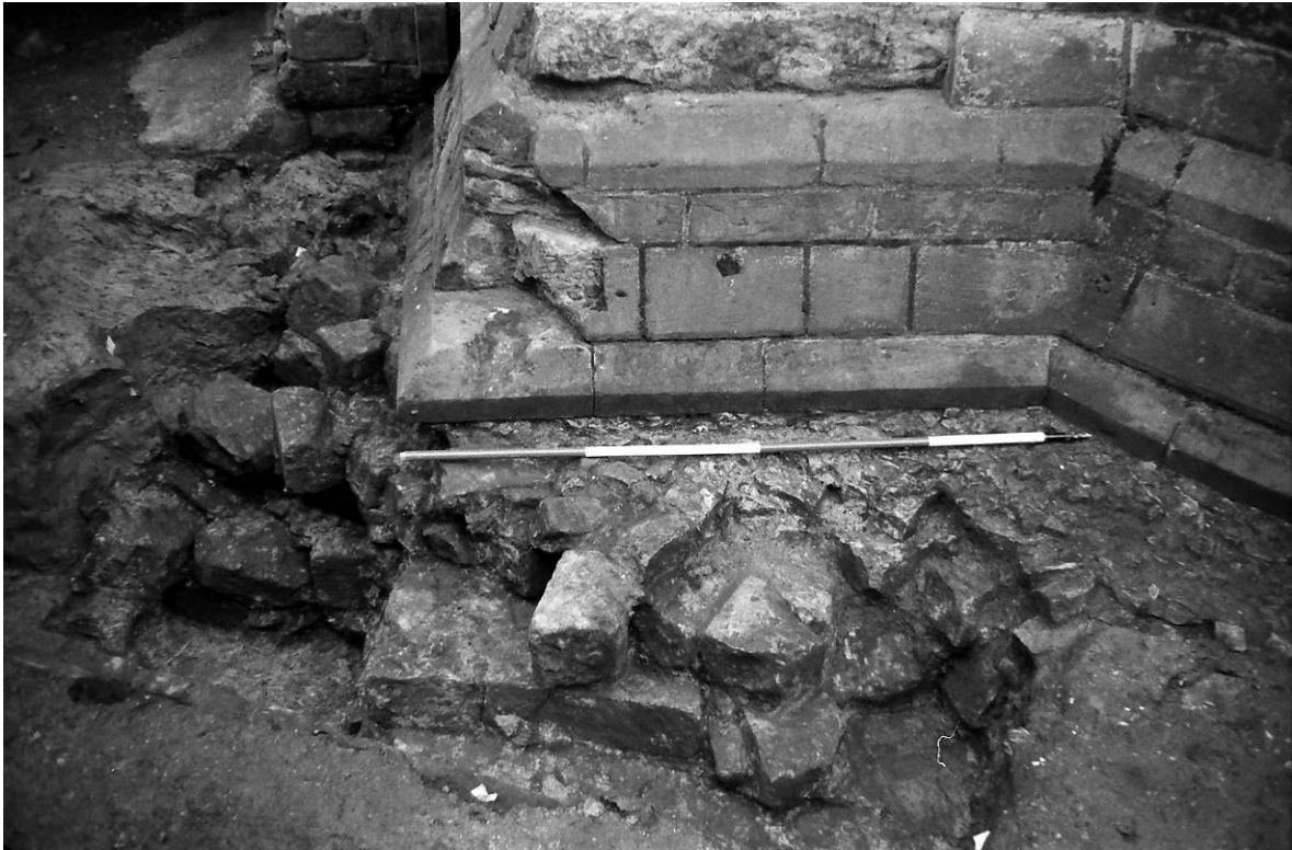
3. Foundation raft ,5005. for the Black Gate during excavation, looking south. This shows the small sandstone chippings and mortar levelling-up surface, removed during subsequent landscaping. Scale 2m. (Film 1984/4/32A)
