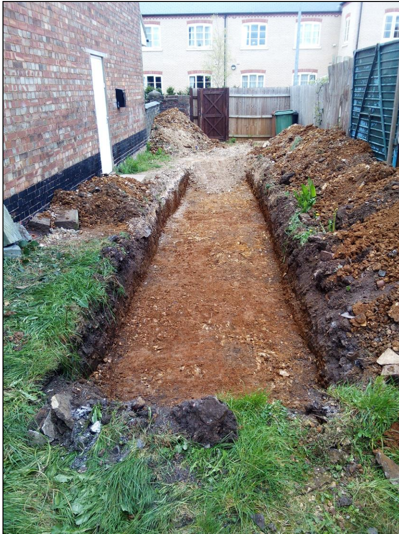
Figure 4. Trench 1. Overview. West facing photo.
