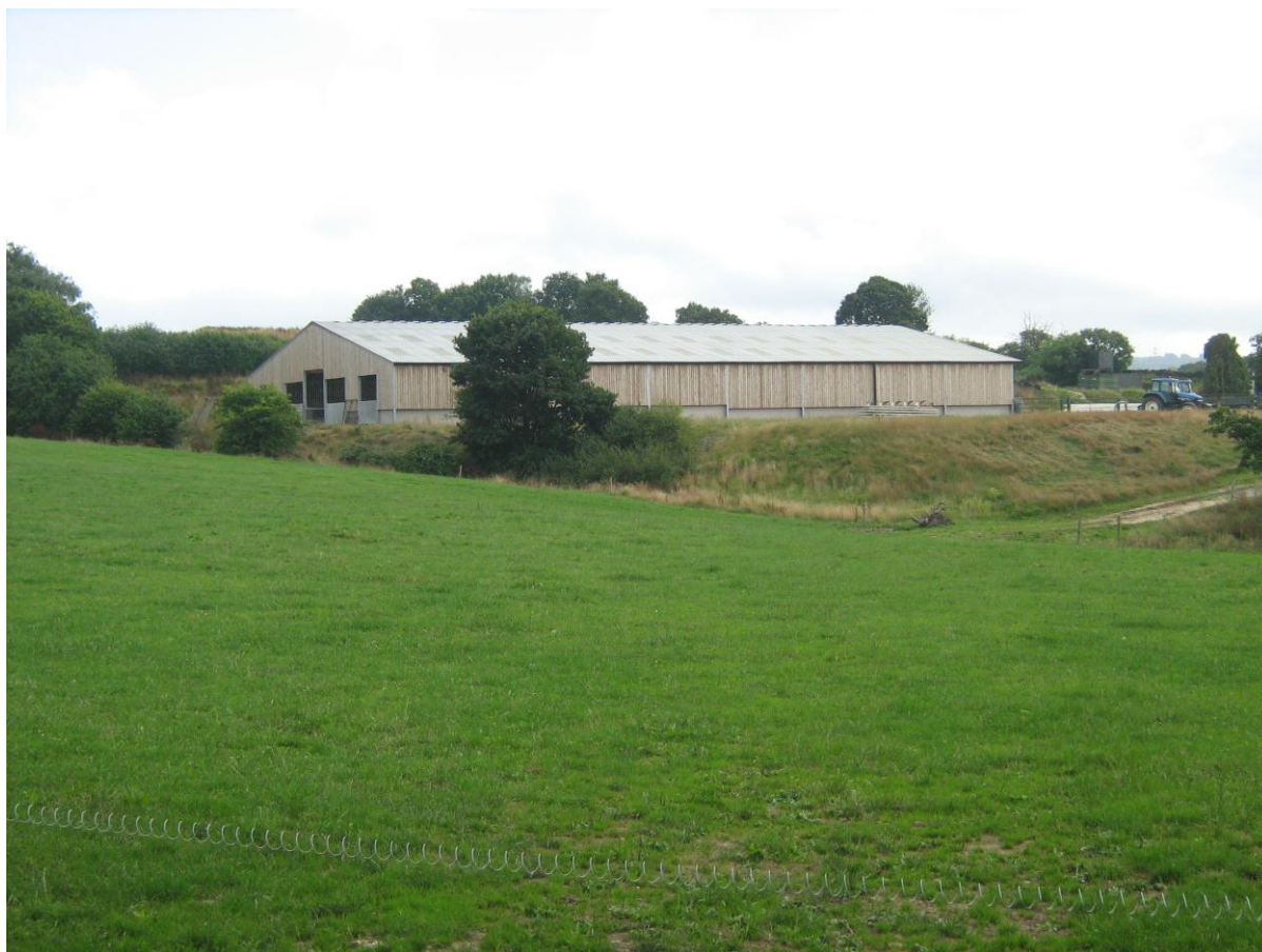
Fig. 3.4 View of the covered yard at Colston Fm which provided an exposure used in Campbell et al. (1998).
