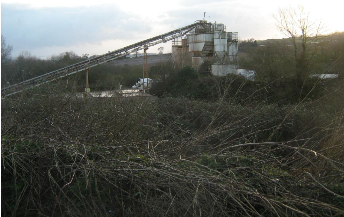
Figure 3.2. Kilmington South Quarry washing plant, March 2013.
