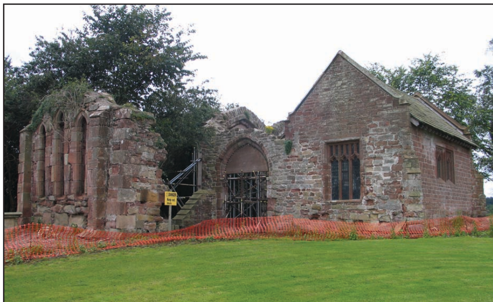
Figure 8. All Saints' Church viewed from the north east in 2007, showing the isolated west chancel wall, the preserved chancel arch and the restored Conyers Chapel
