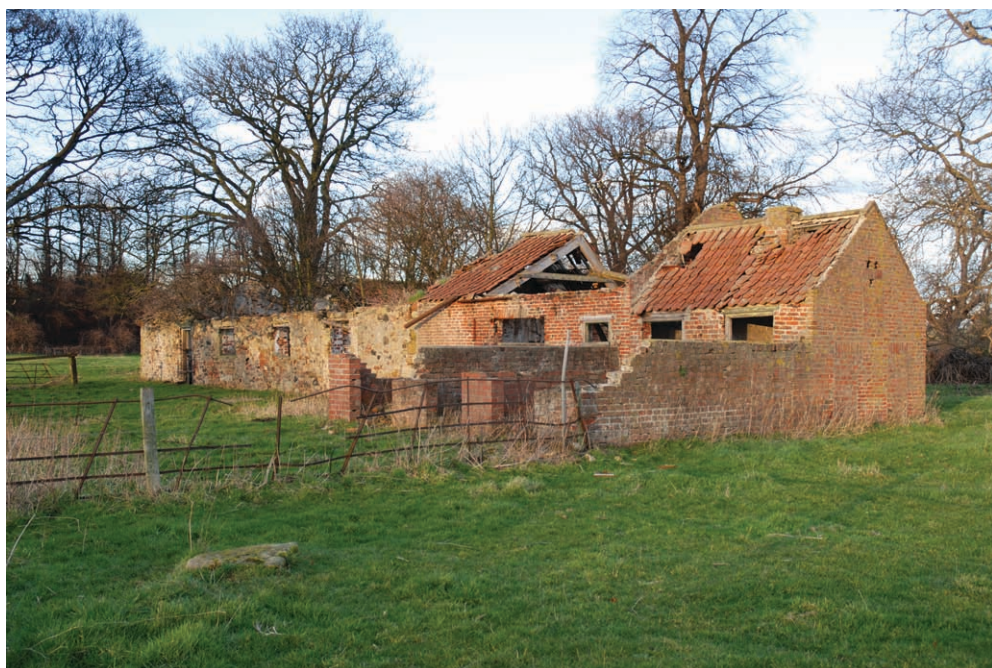
Figure 30. The brick-built extension, pigsties and 'poultiggery' at the southern end of the farm buildings © C J Dunn
