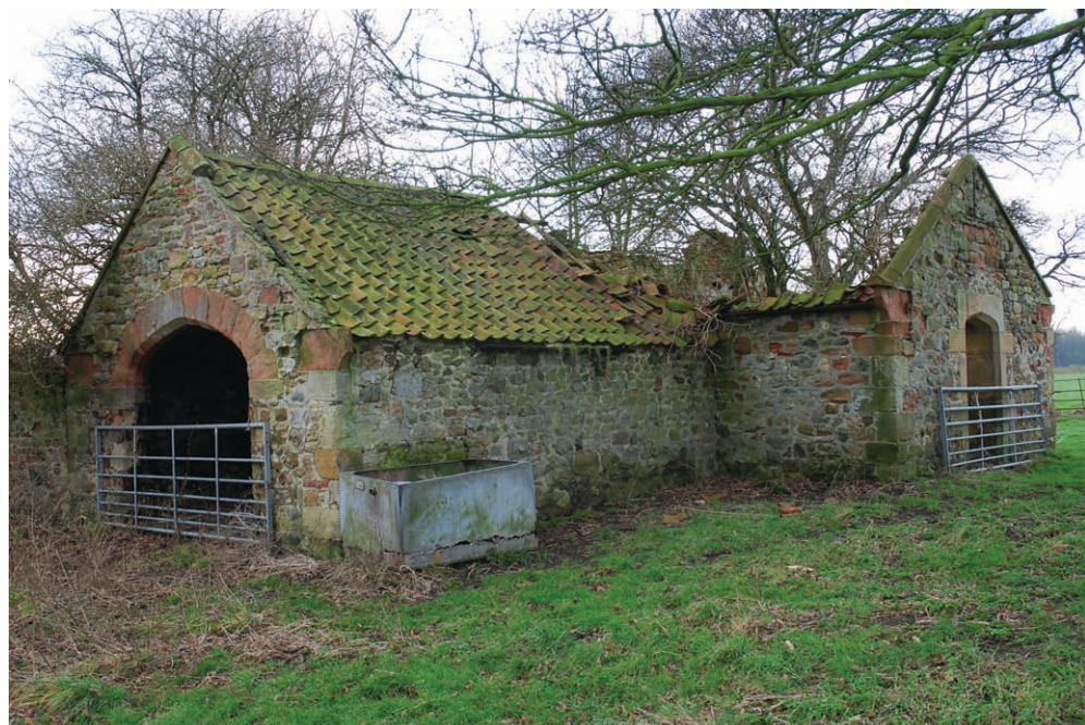
Figure 29. The agricultural buildings viewed from the north east showing the ornate doorways facing north (narrow) and east (wide). (© C J Dunn)
