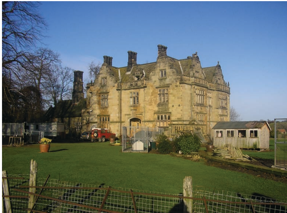
Figure 14. Sockburn Hall viewed from the south west
