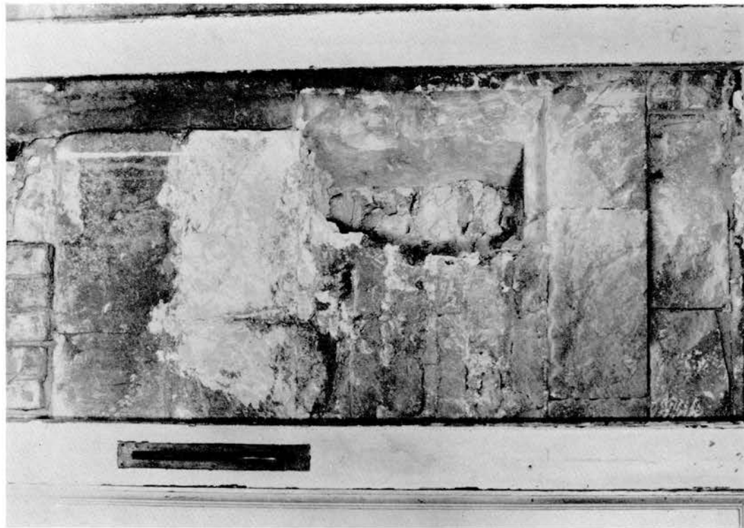
(a) Window A: bottom right-hand corner, showing medieval sill and splay, and later in-filling.
