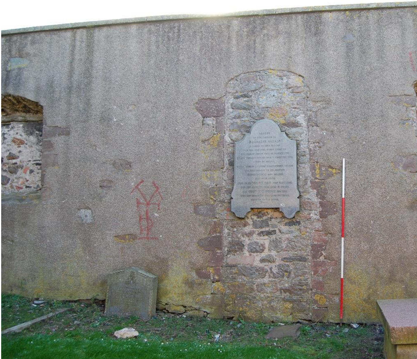
Illus 48 South wall interior: (l-r) W8, D5, W2, W1,D1, W7
