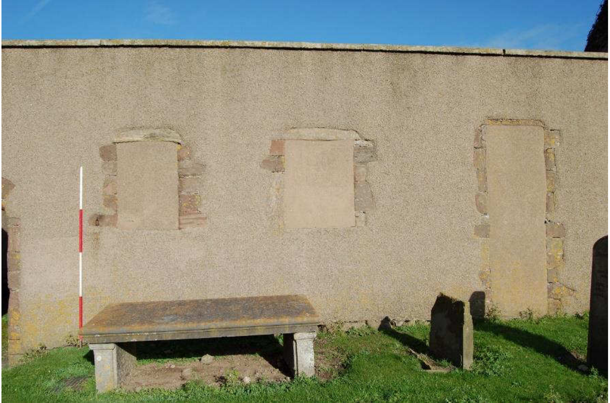
Illus 49 South wall exterior: (l-r) Door 1, window 1, window 2, door 5
