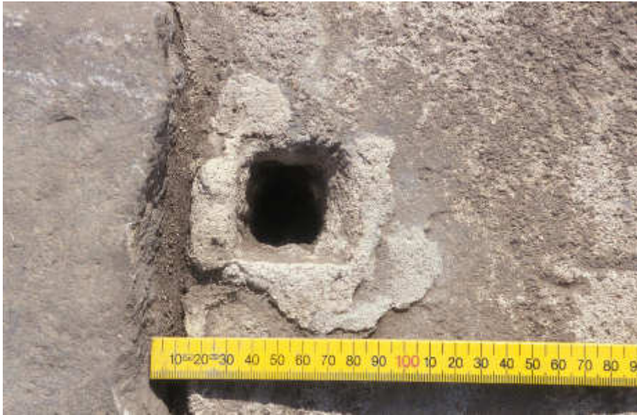
Illus 32 Building 2, Looking south down steps AG showing hole for railing AY
