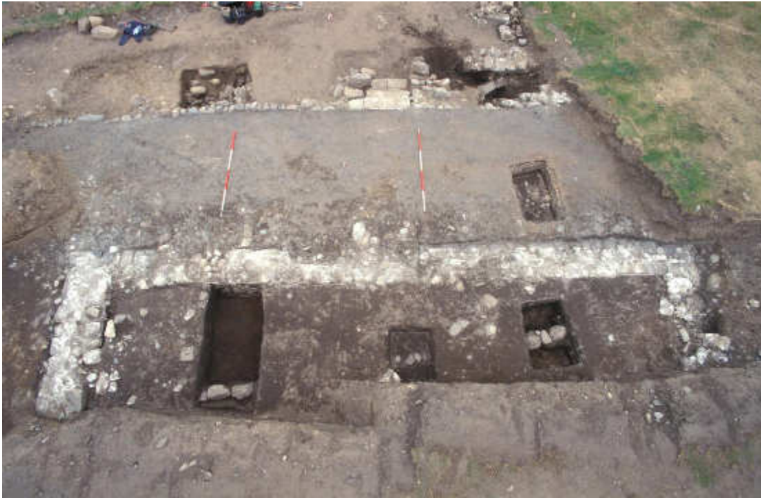
Illus 29 Foundations of manse building (Building 2) foreground, driveway (with 2m scales) and garden (top); facing south
