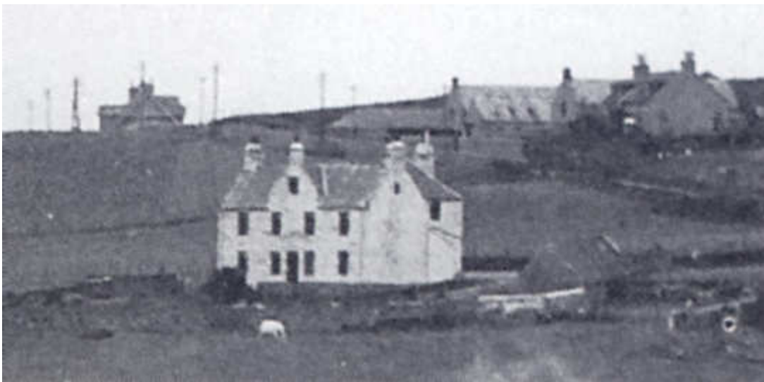
Illus 30 Building 2, manse (foreground) showing Kirkhill Farm (background right) prior to the development of Balnagask (copyright Aberdeen Journals)
