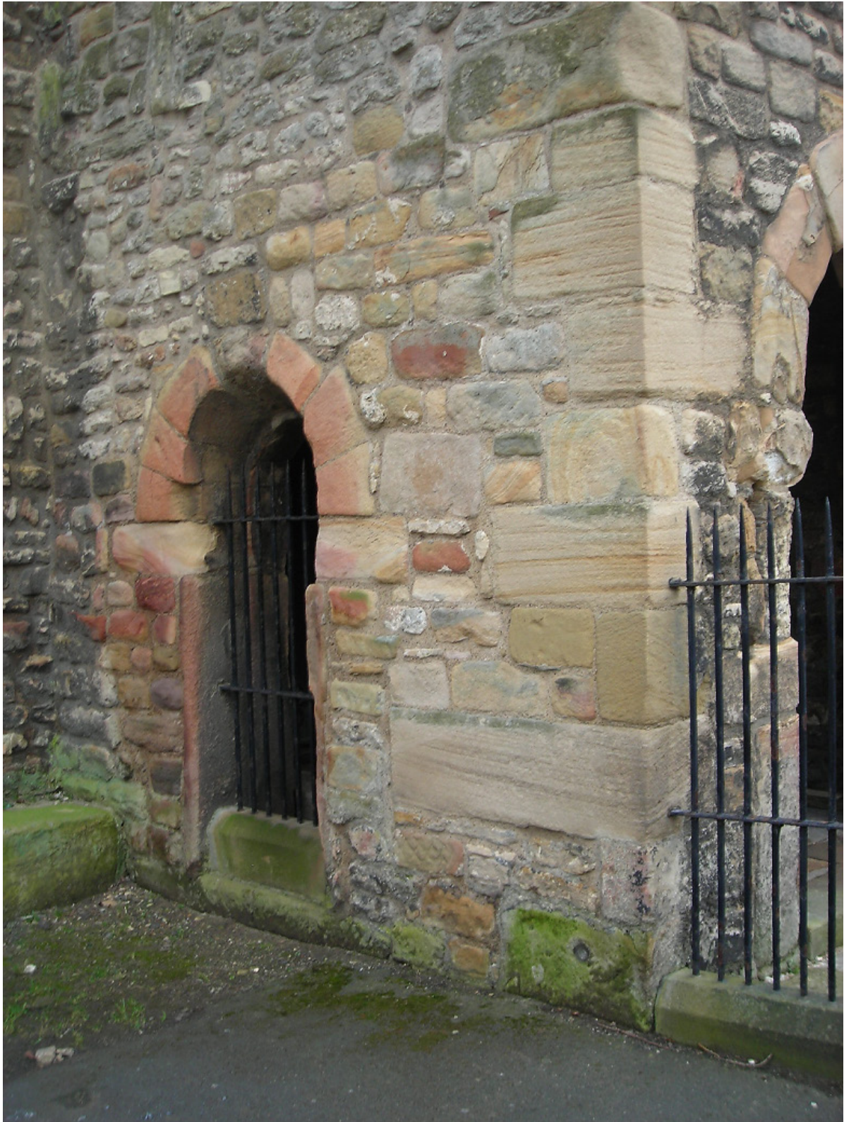
Figure 3a: Entrance on north side of the porch, St. Peter's, Wearmouth. Shows burned ashlar in situ.
