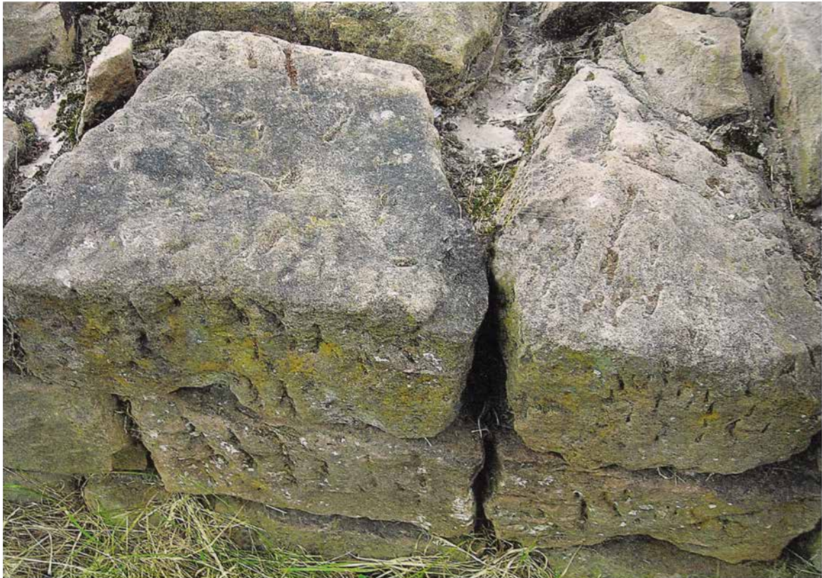
Figure 18: Arbeia: example of squared rubble blocks executed in Wrekenton Sandstone with a c. 25 cm lift height and tapered backs.
