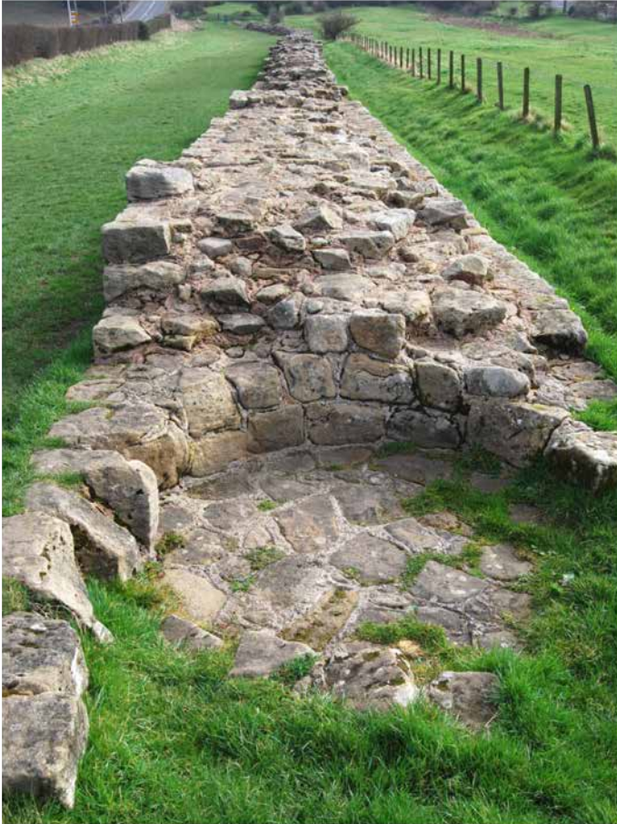
Figure 23: Roman Wall section at Heddon-on-the-Wall, constructed with local Millstone Grit ('Third Grit' Lower Carboniferous; NZ 130668).
