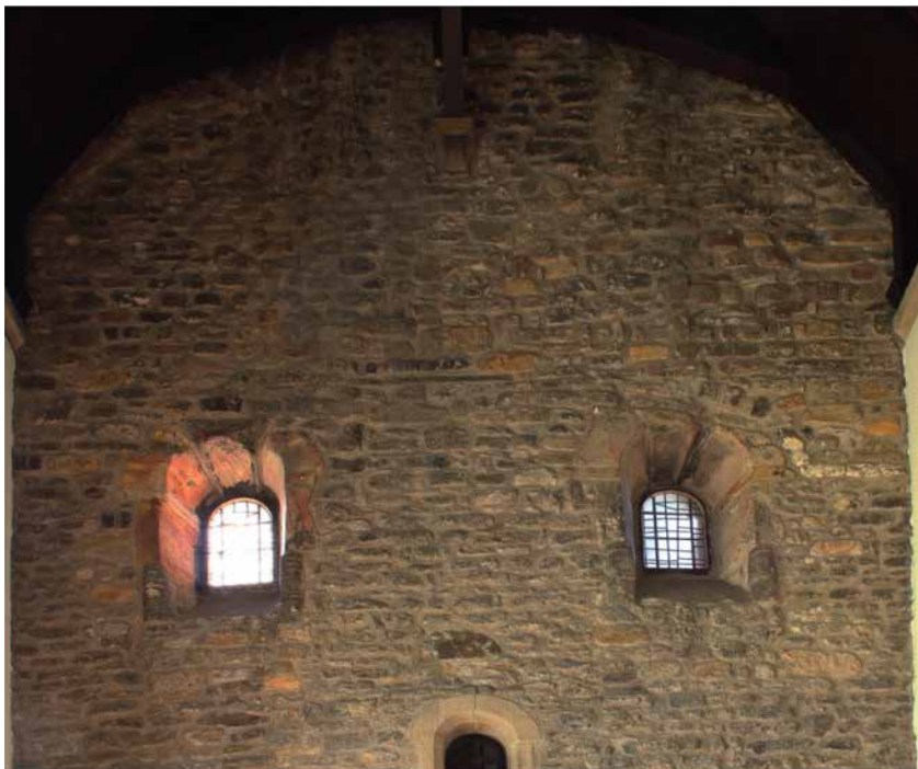
Figure 41a: interior stone work at the western end of the nave at St Peter's, Wearmouth, showing the burnt areas around the upper windows.
