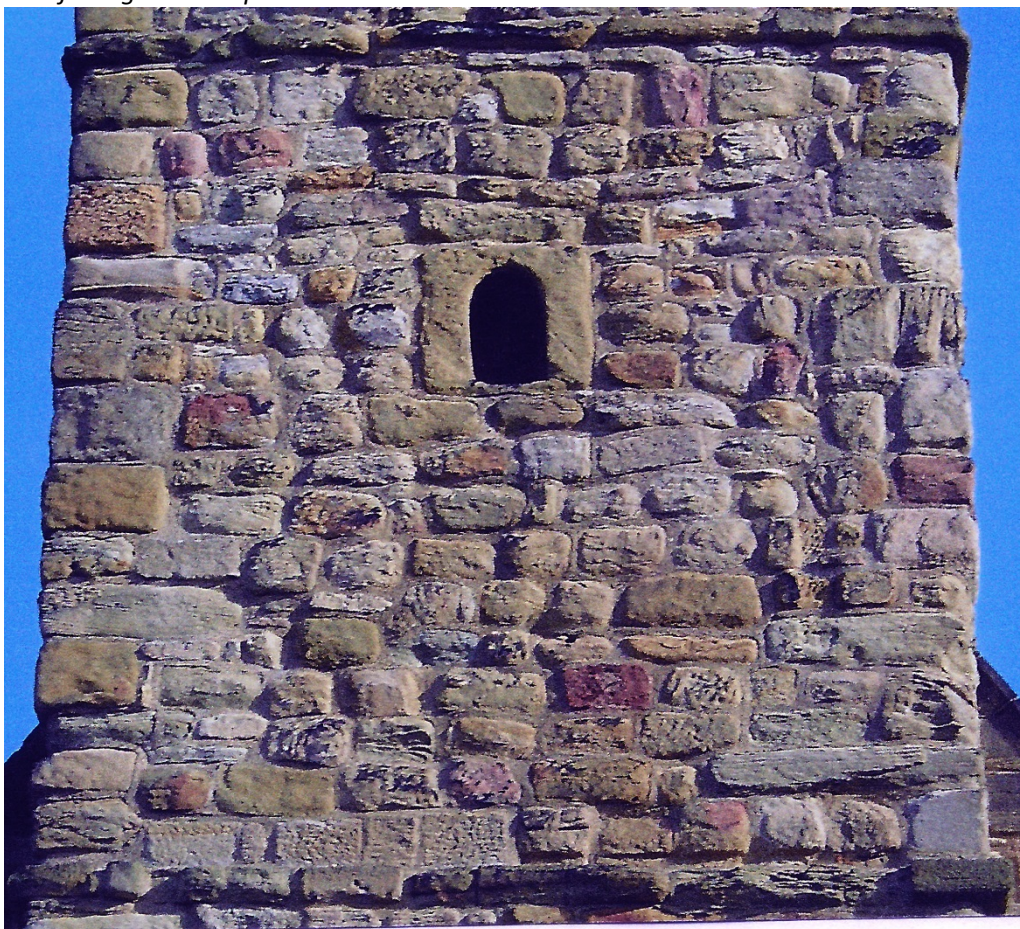
Figure 18: Arbeia: example of squared rubble blocks executed in Wrekenton Sandstone with a c. 25 cm lift height and tapered backs.
