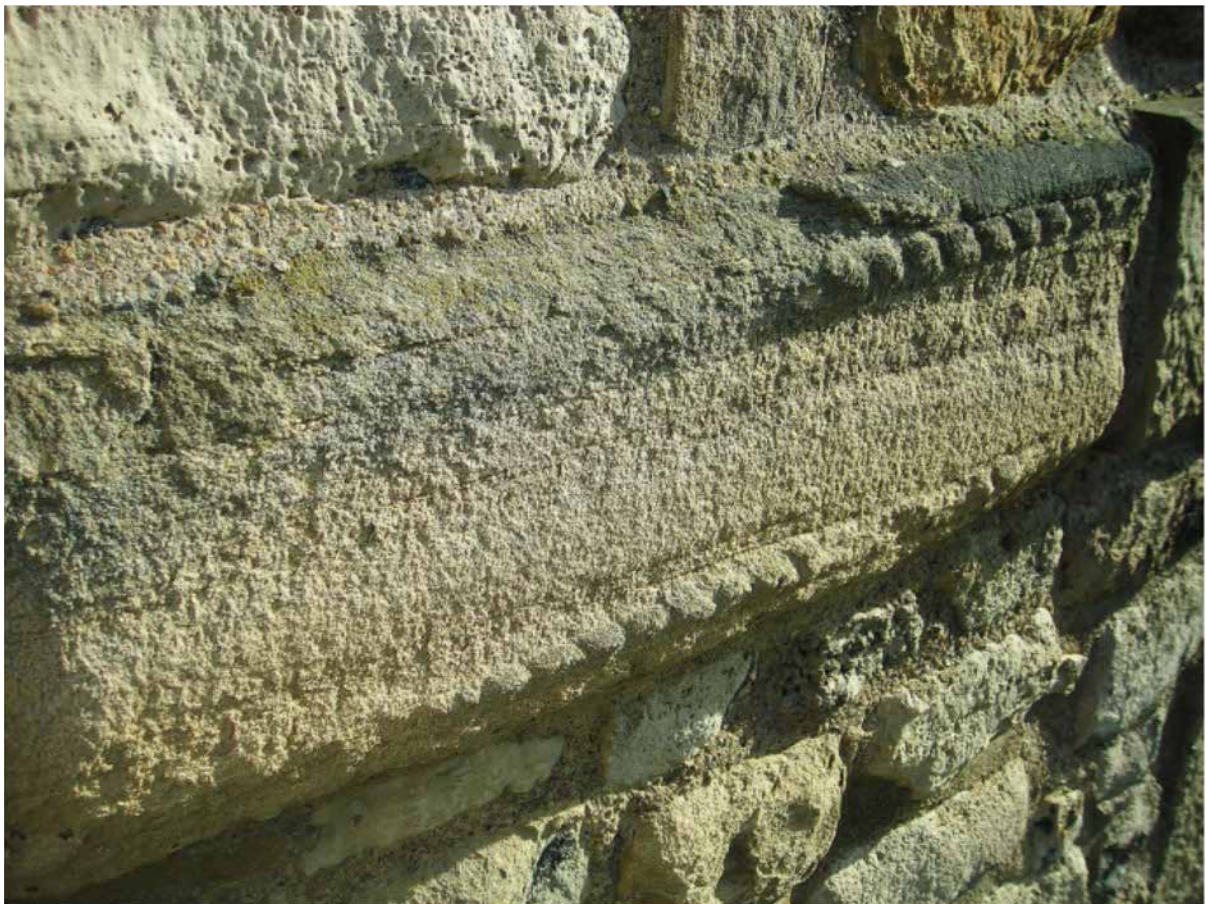
Figure 12b: Roman frieze: strong coursing, west face of porch at St. Peter's, Wearmouth.
