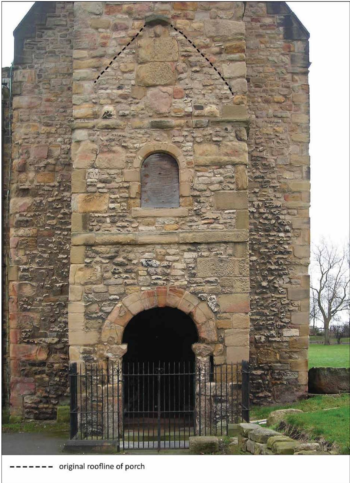
Figure 2: Western porch entrance, St. Peter's, Wearmouth. Showing original roof line.
