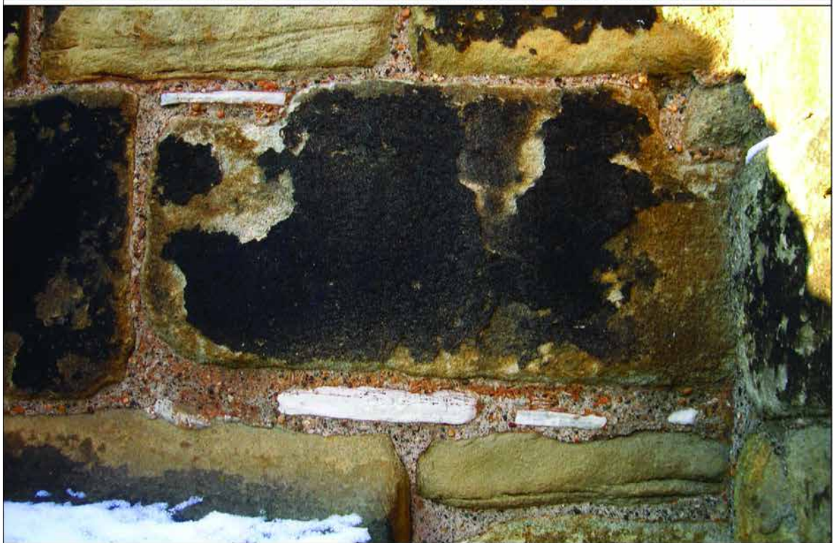
Figure 33: Use of Magnesian Limestone in an Anglo-Saxon context at St. Paul's, Jarrow: a) as packing in the frame of the North Doorway; b) As packing at the east end of the church (south-east corner). 26
