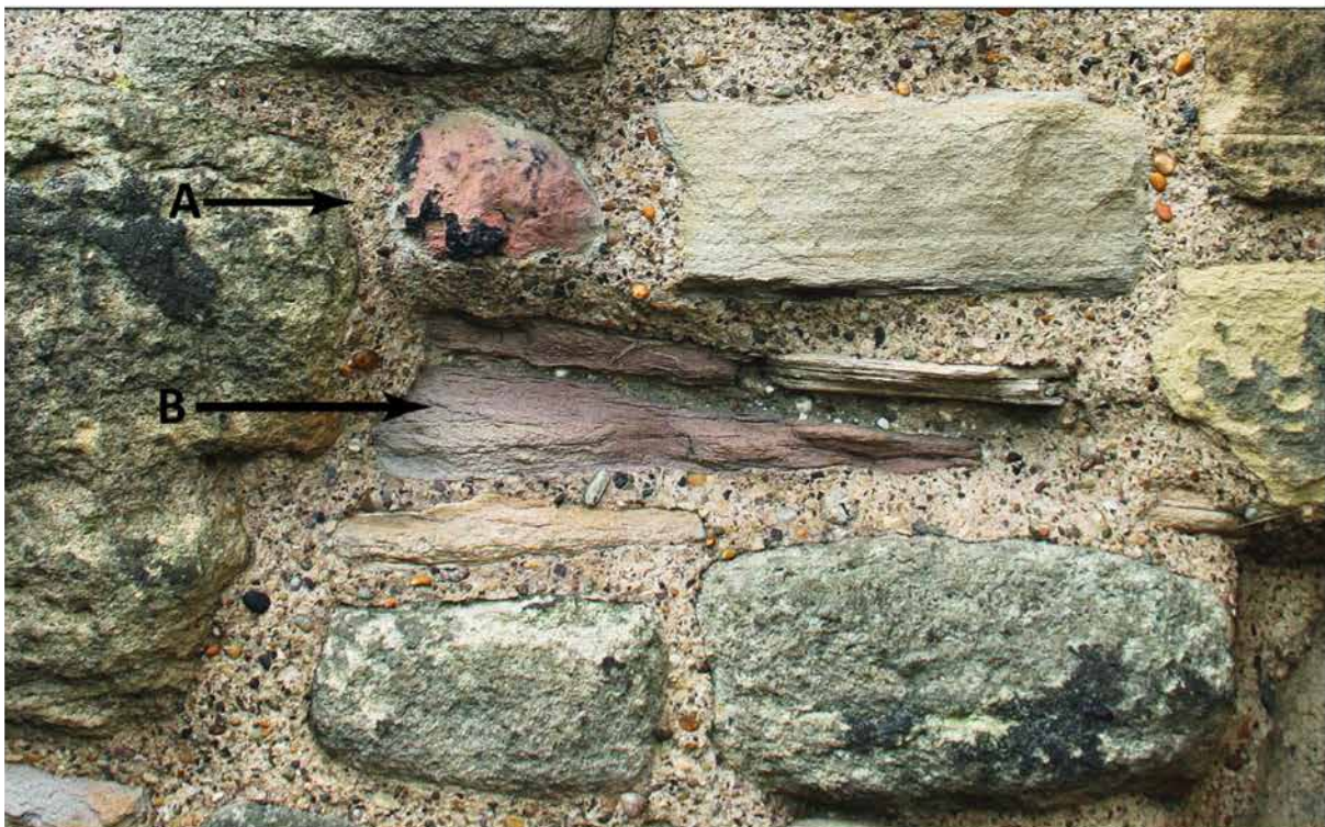
Figure 25: Top: Naturally reddened sandstone from Dean Quarry and Roman stone cut from pale oolitic dolomite. St. Peter's, Wearmouth. Bottom: Reddened sandstone fragment in the Anglo-Saxon fabric of St. Paul's, Jarrow(B) , located in the south-east part of the external east wall. Sitting below a fragment of reddened Roman brick (A).
