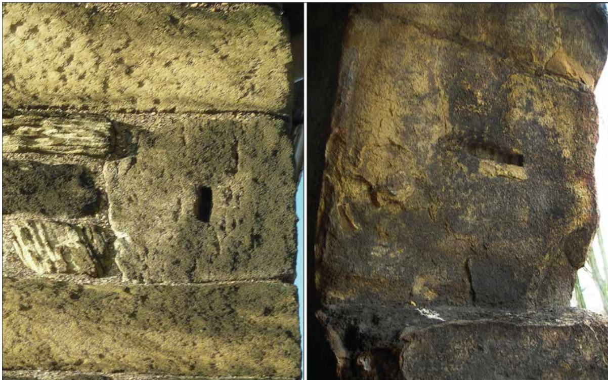
Figure 10: Left: Lewis lifting hole in reused Roman ashlar: quoin at south-east corner of the eastern chapel at Jarrow. Right: Lewis lifting hole in reused Roman ashlar: voussoir on southern side of the western porch entrance at Wearmouth.
