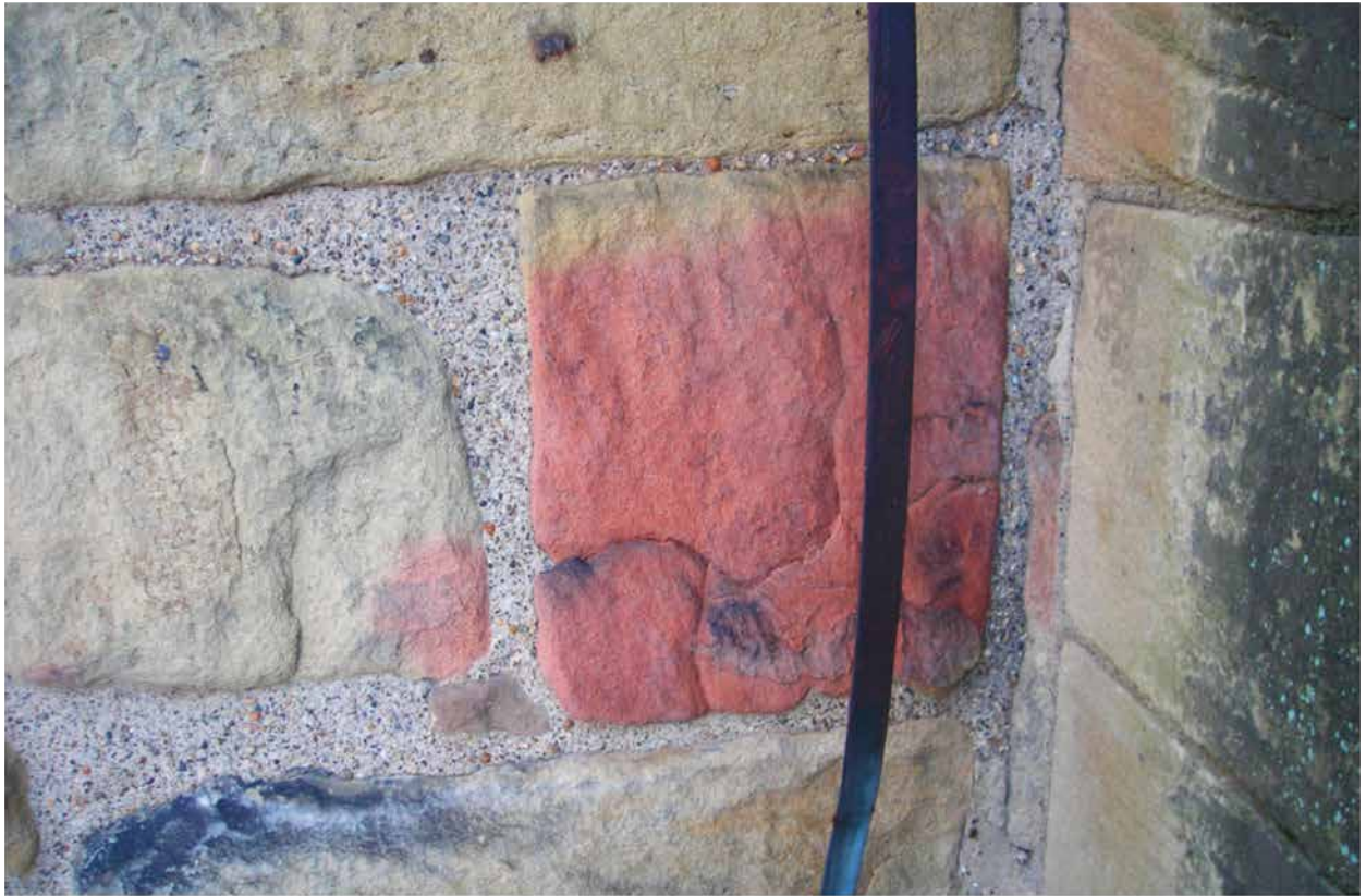
Figure 29: Roman cut stone blocks reused at Jarrow. Exterior, north-west corner of Eastern Church. Stones appear to have been burned prior to their use in the pre-Conquest structure.
