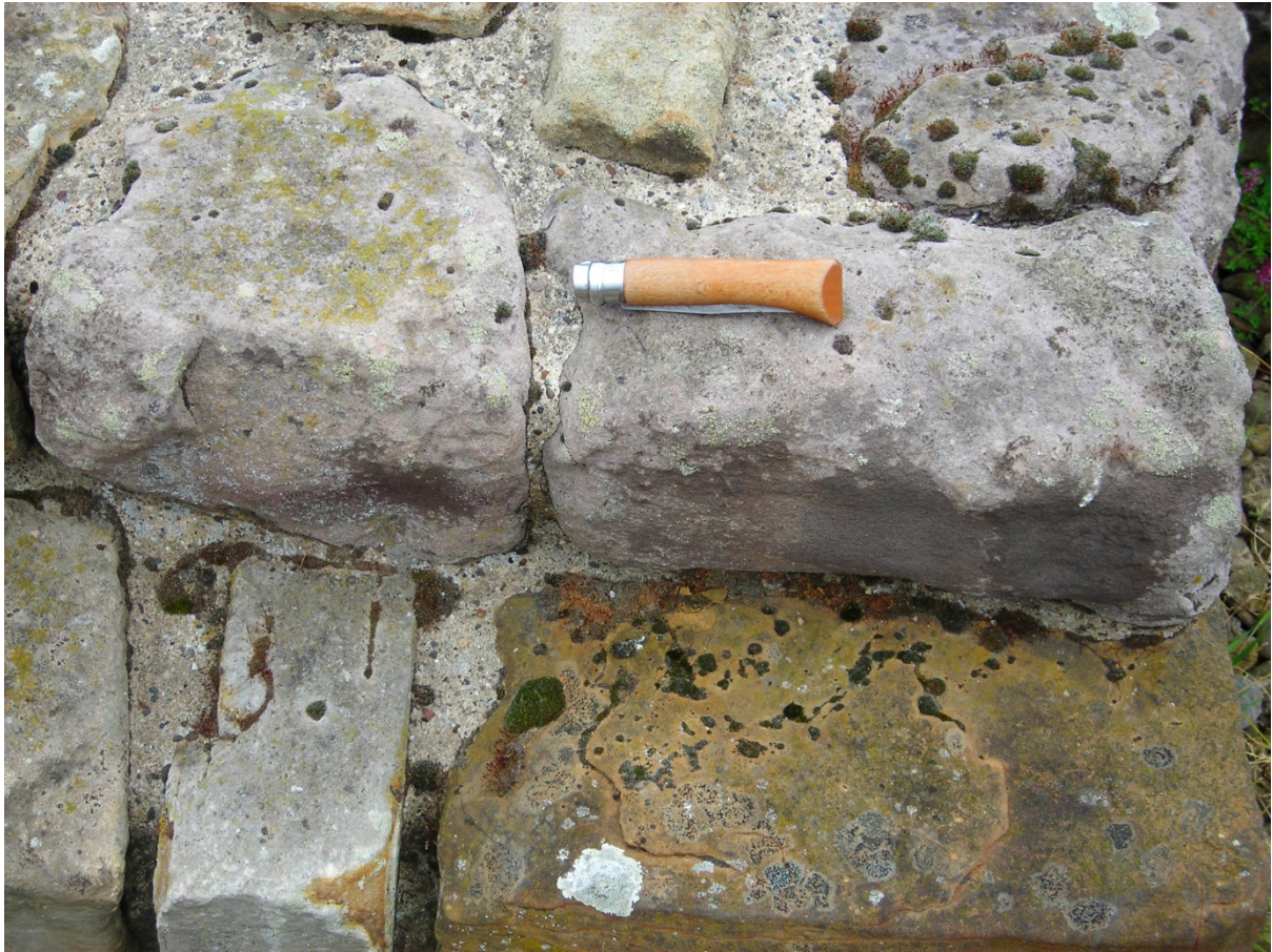
Figure 32: Arbeia: squared rubble walling in Dean Sandstone (Type B). Note the pick shade to the body colour of the stone.
