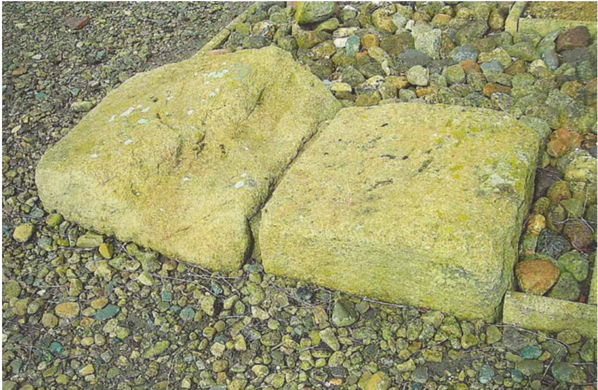
Figure 26a: Base blocks of Millstone Grit used for the East Gate at Segedunum. Bottom:
