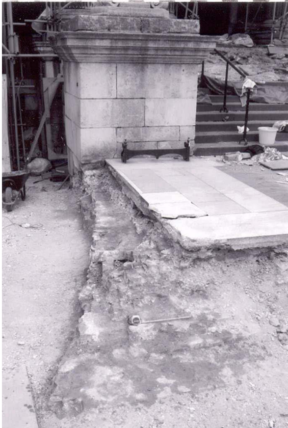
Fig 68 Original line of lower balustrade of west steps, north side, looking east
