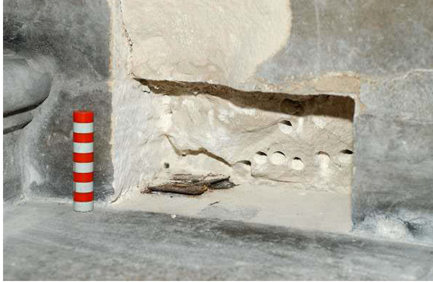
Fig 74 Detail of the investigation into the side wall of the stair. This shows the exposed iron shim which was inserted by Kempster to tighten the joint between the tread and the surrounding wall; each tread has its end inserted into the wall. Scale is 10 x 10mm units
