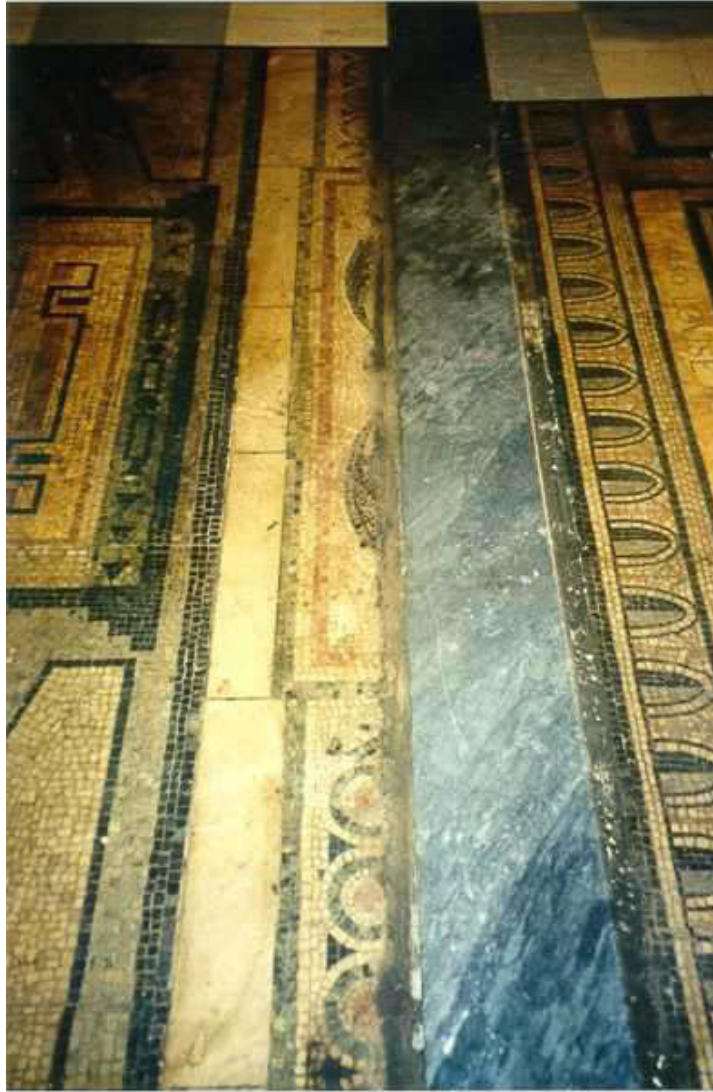
Fig 82 detail of the step between the central bay (left) and the western bay (right), looking south
