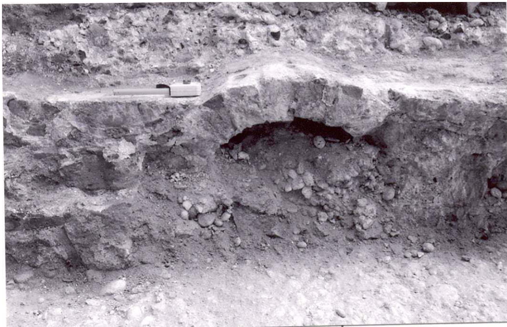
Fig 70 Brick arch in north side of foundation for lower balustrade
