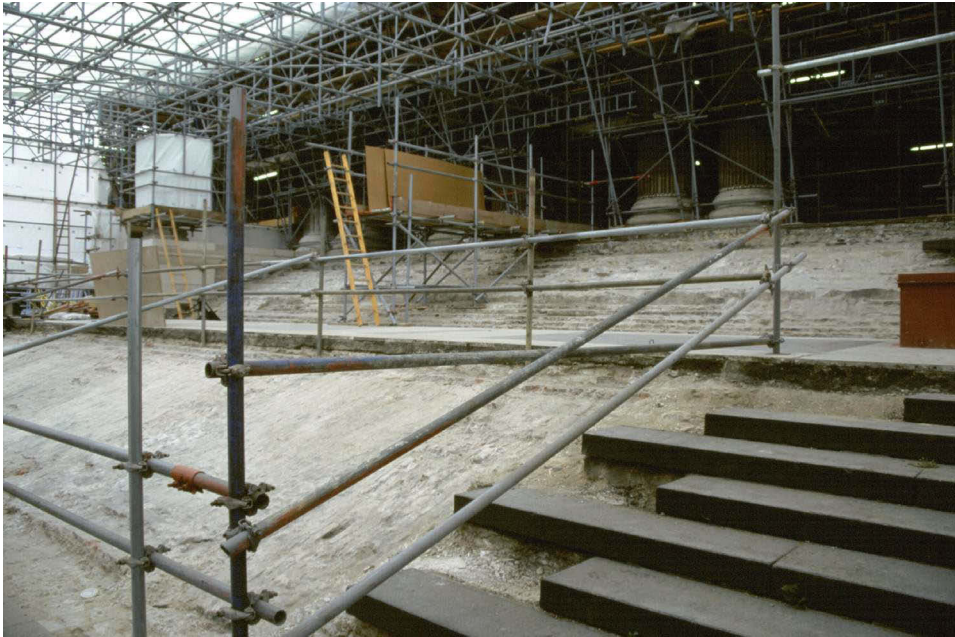
Fig 64 The west steps from the south-west, with the majority of steps removed; those on the right remain from the pre-restoration arrangement
