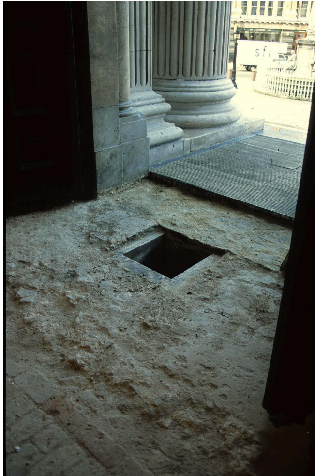
Fig 77 The NW doorway, with the former revolving door removed: socket [3], looking SW
