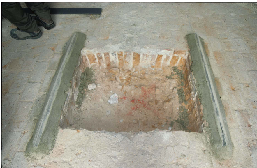
Fig 78 The area of the crypt vaulting, within the NW doorway, which had to be removed to install the new revolving door, looking E; the crown of the crypt vault is shown. This is the site of the sampled bricks [2]
