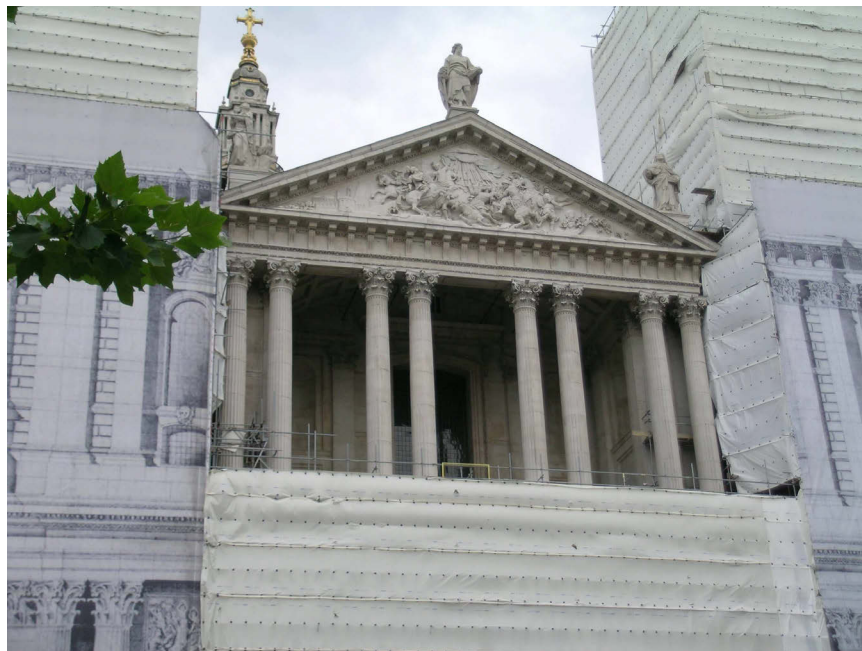
Fig 16 The central section of the west front revealed after cleaning, June 2004
