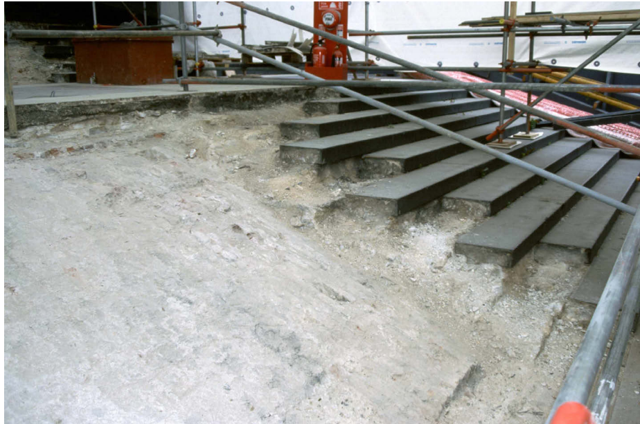
Fig 67 The substructure of the Wren steps, looking south, with the pre-restoration steps of the south part still in place
