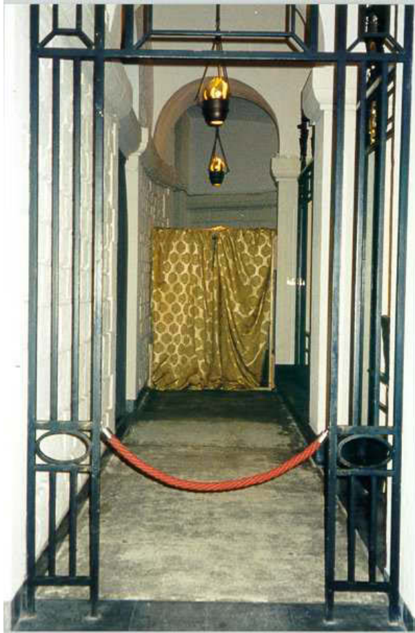
Fig 86 The north ambulatory passage, looking east; the concrete floor had been laid within living memory of cathedral works staff
