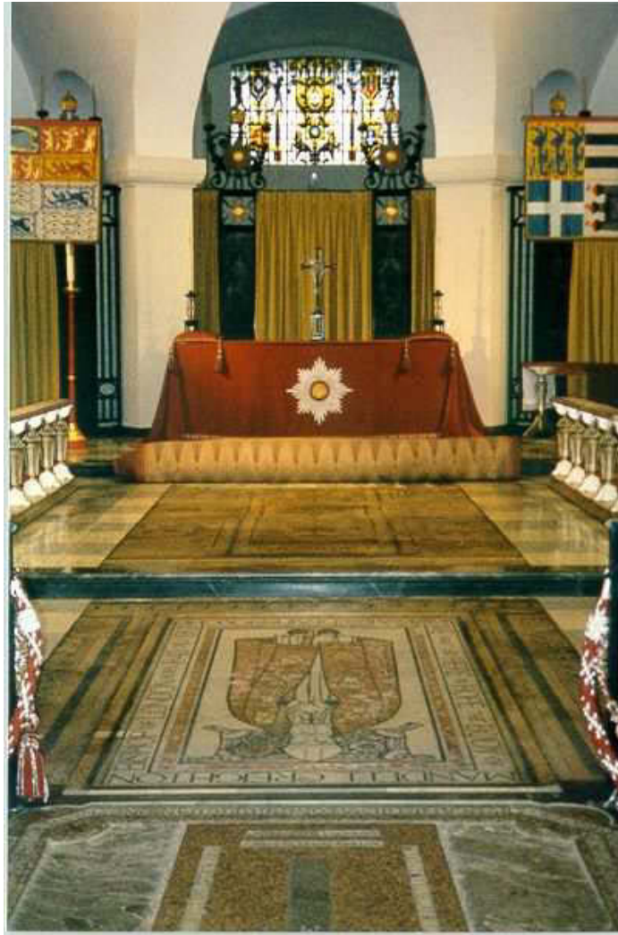
Fig 80 OBE Chapel, looking east: the ledger of Bishop Creighton in the foreground, Penrose's mosaic on both sides and to the east, and the 1950s vinyl tiles (some of which have been removed)
