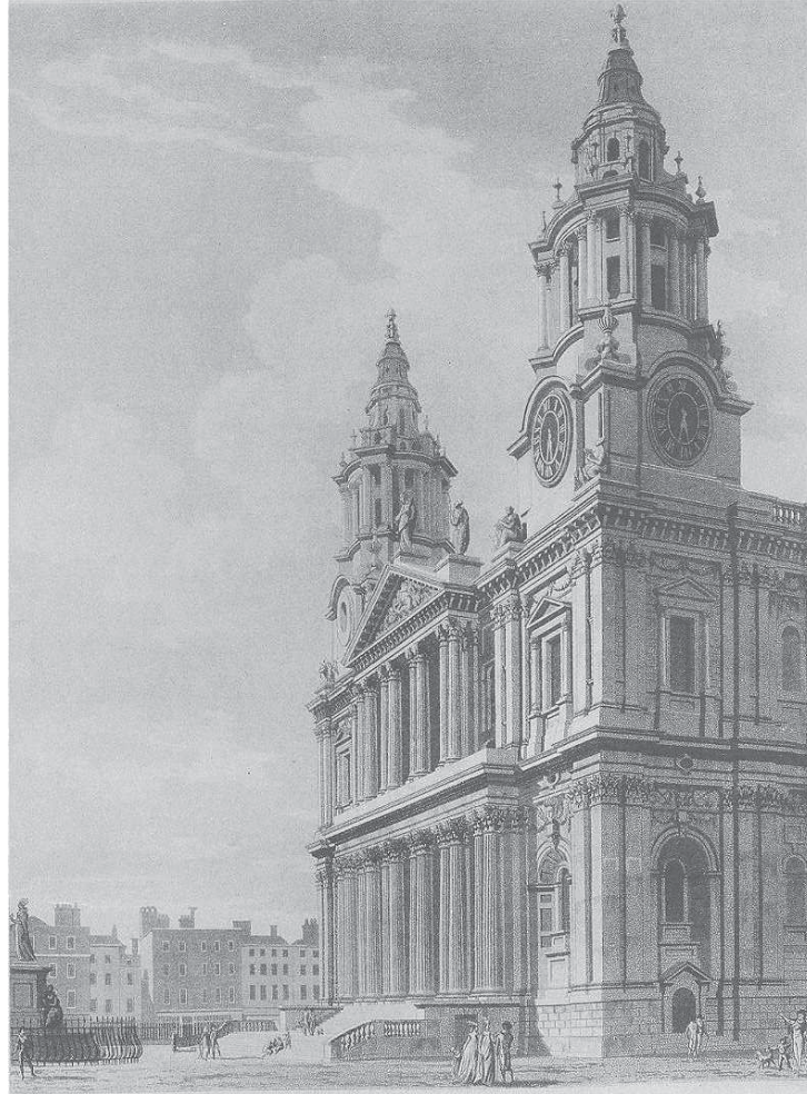
Fig 10 The west end of St Paul's from the south side, by T Malton, 1798 (from WS XIV, plate XVII). This shows the curved west steps and the cast iron railing (not Wren's original design, but the second imposed by the Commissioners) around the statue of Queen Anne (both railing and statue since replaced)
