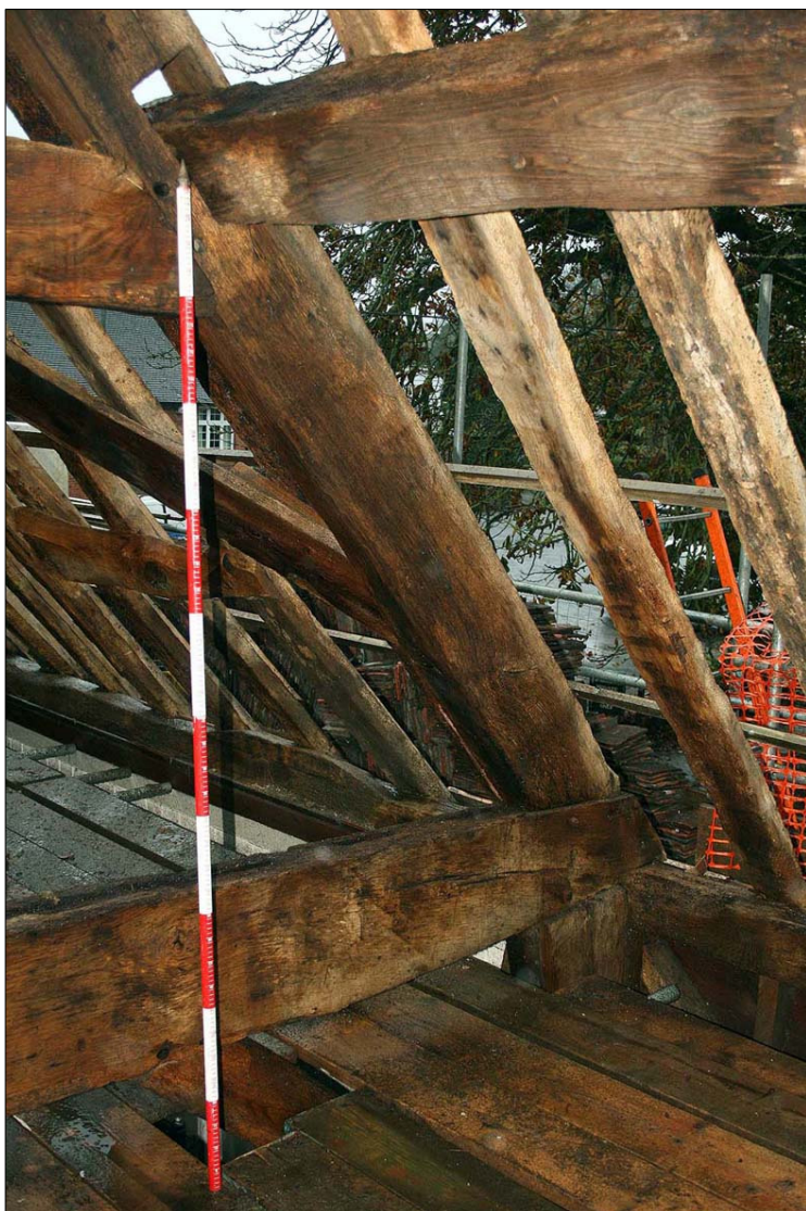
Fig.43. Bay 5. Replacement principal rafter on the north side of cross-frame 5.
