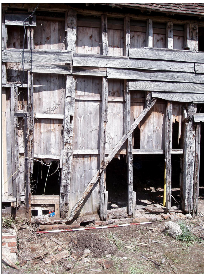
Fig.27. Bay 4. Condition of Phase 1 and Phase 2 timbers in the south elevation. Facing north.
