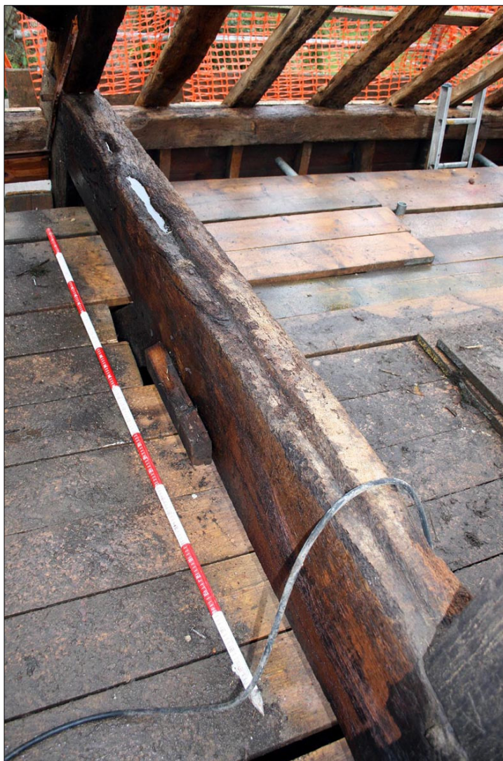
Fig.35. Bay 4, truss 5. 'V' groove on the upper side of the tie beam denoting the position of stud wall. Facing north-east.
