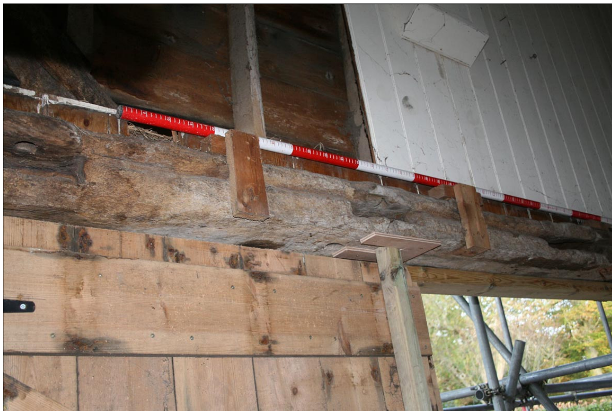
Fig.25. Bay 3. A re-used mid-rail acts as a lintel above the entrance to the Phase 2 (i.e. the 18 th / 19 th centuries) loading bay. Facing north-east
