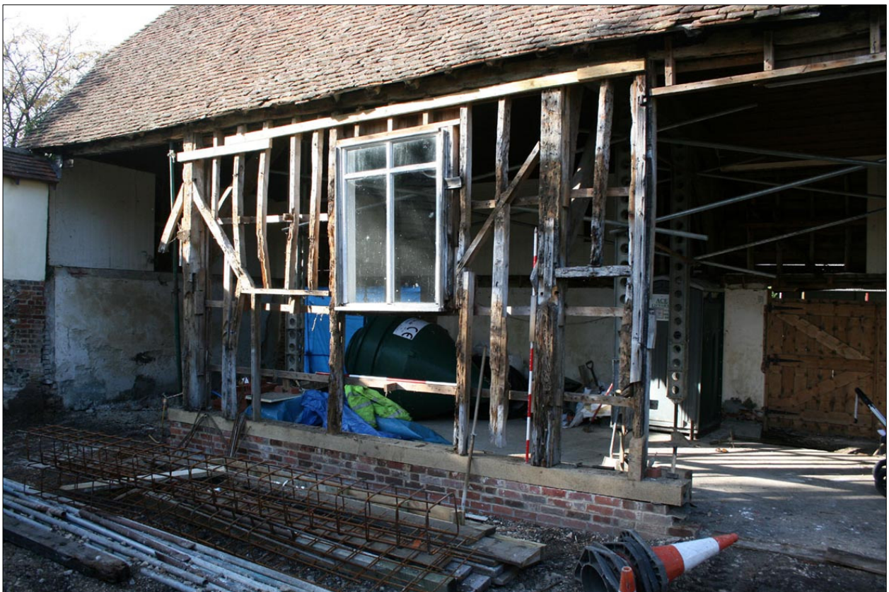
Fig. 11. Bay 1 and 2. Remains of medieval and post-medieval timber framework in the south elevation. Facing north-west.
