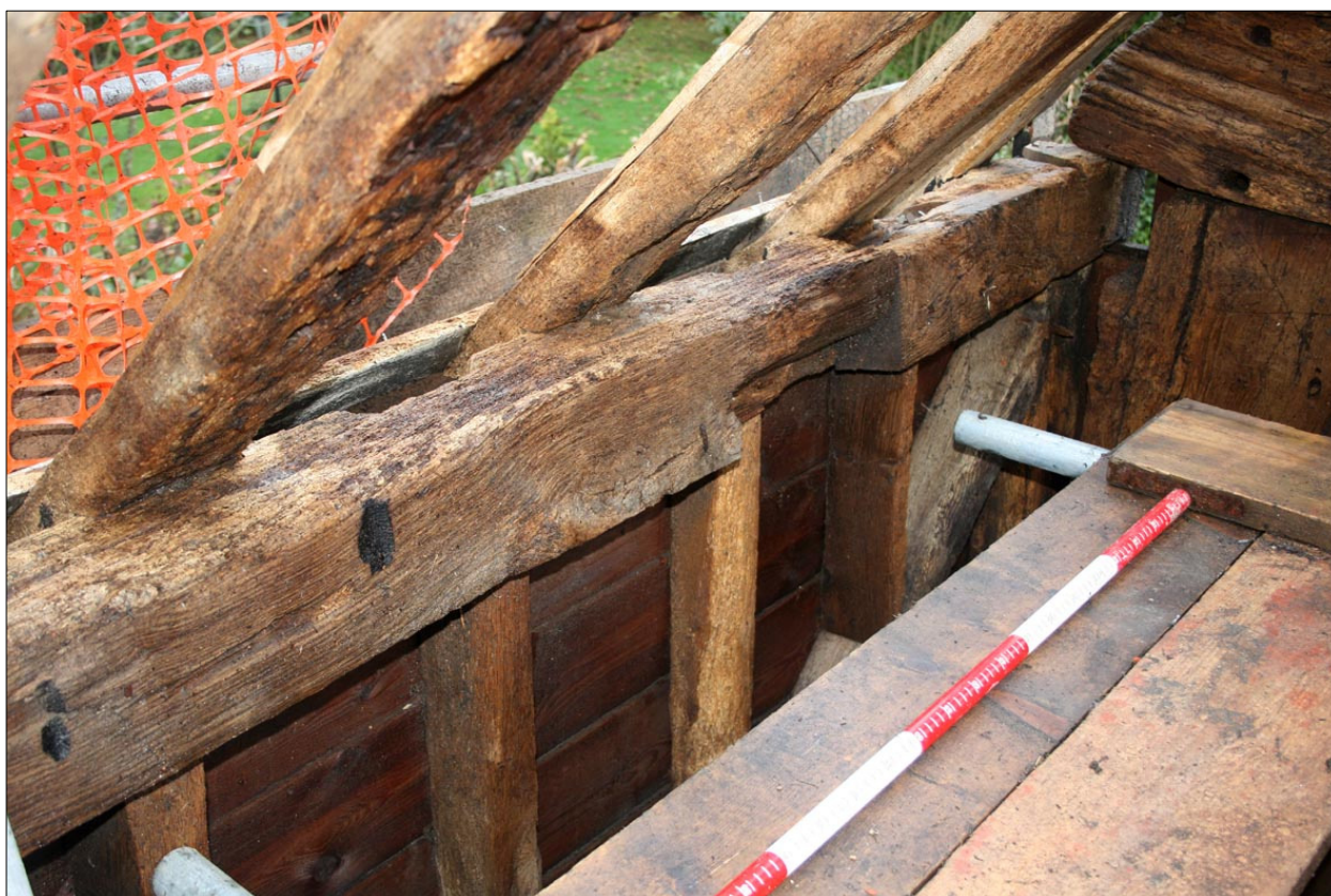
Fig.38. Bay 5. North elevation. Wall plate and post-truss (6) joint. Facing north.
