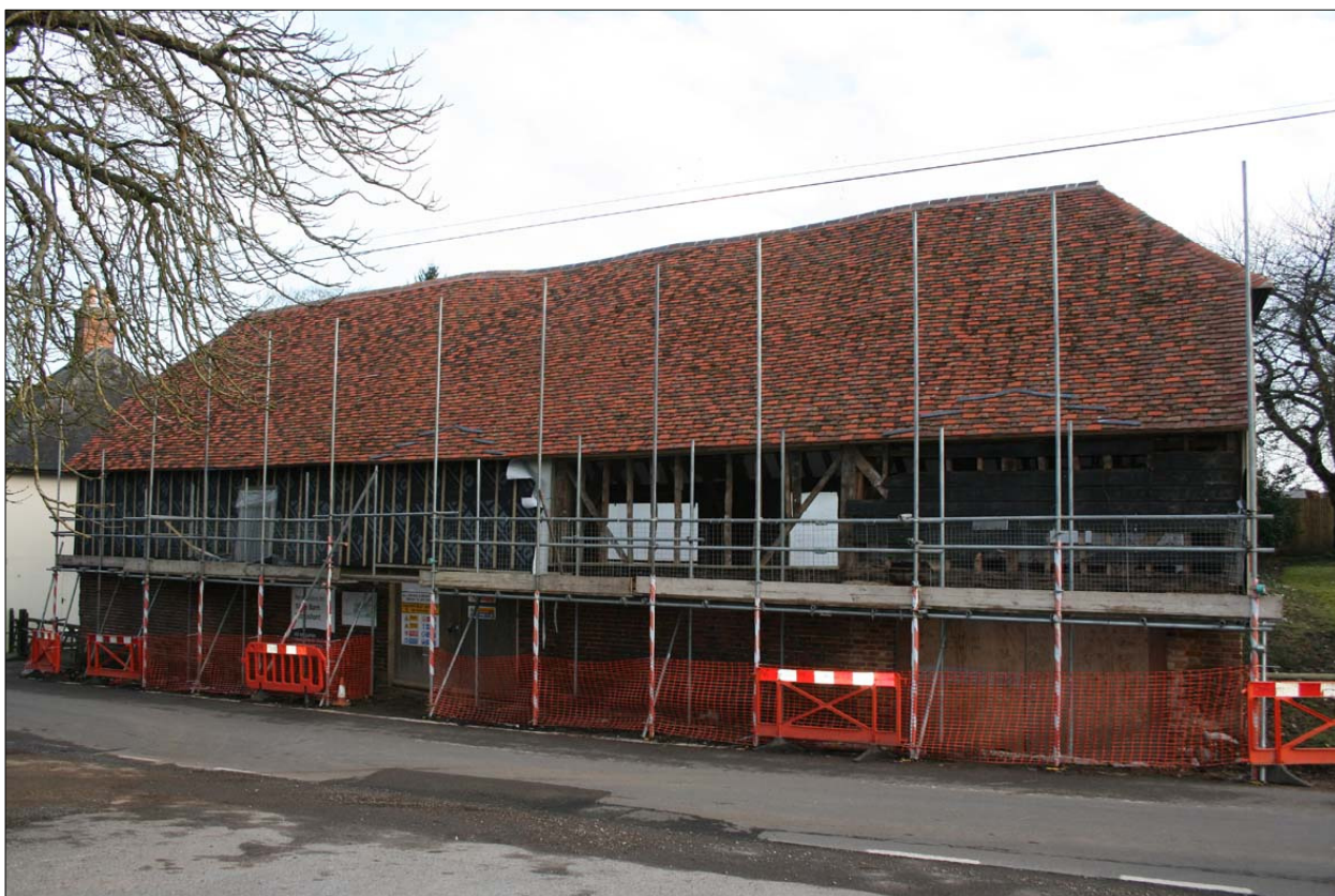
Fig. 48. North elevation after re-tiling, and during the stripping and re-cladding of the wall
