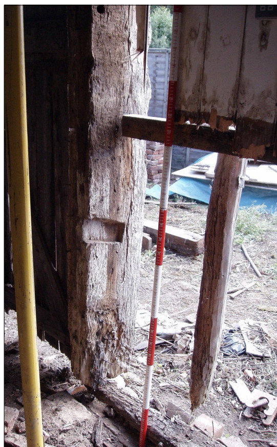
Fig.28. Bay 4. South elevation. Mortise for Phase 2 manger; principal post 4 Facing south-east.
