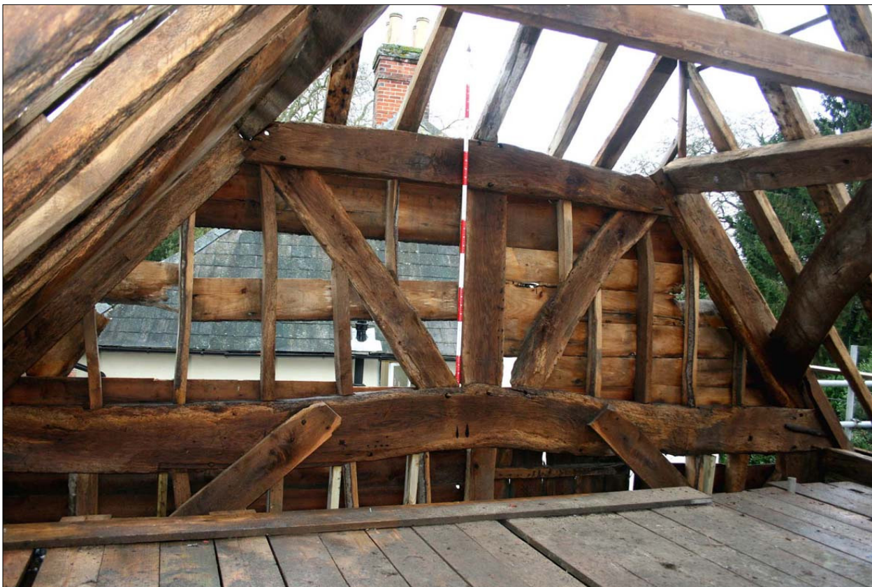
Fig.40. Bay 5. The 'fan truss' of the east end frame. Facing east.
