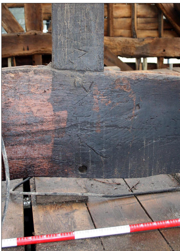
Fig.33. Bay 4, truss 5; Tie beam-crown post joint, with both medieval and 18 th century carpenter's numerals. Facing east.
