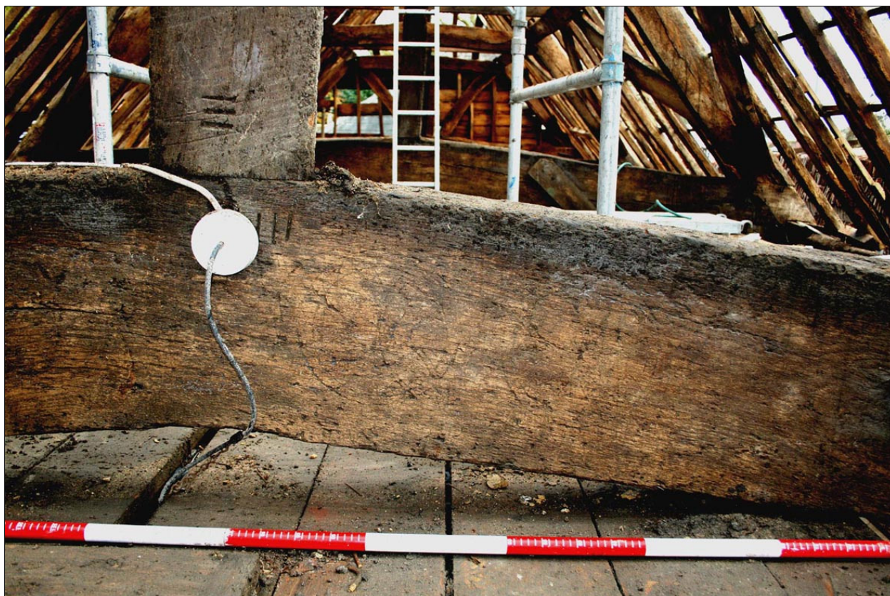
Fig.21. Bay 2, truss 3, facing side. Tie beam-crown post joint, showing a series of superimposed Phase 1 'daisy wheels' and Phase 2 numerals.
