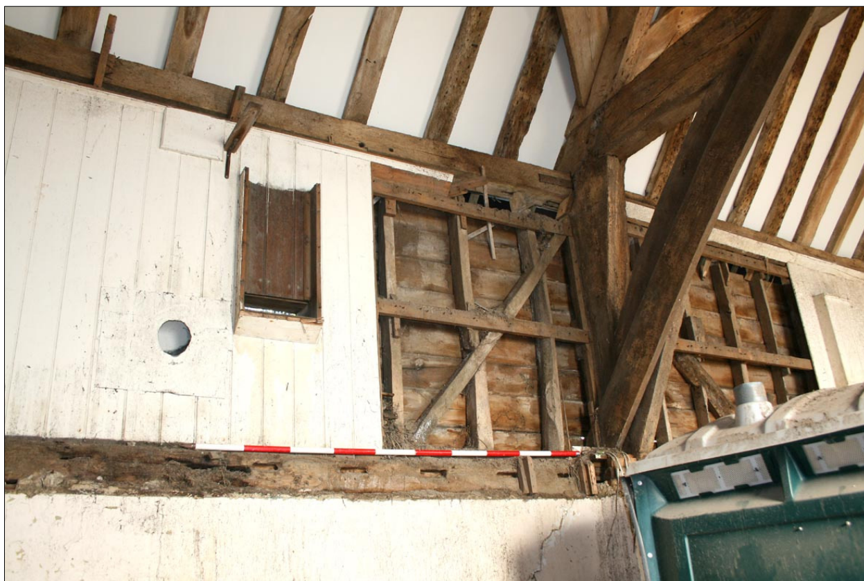
Fig.20. Bay 2. North elevation (partially exposed) and truss 3 (N).
