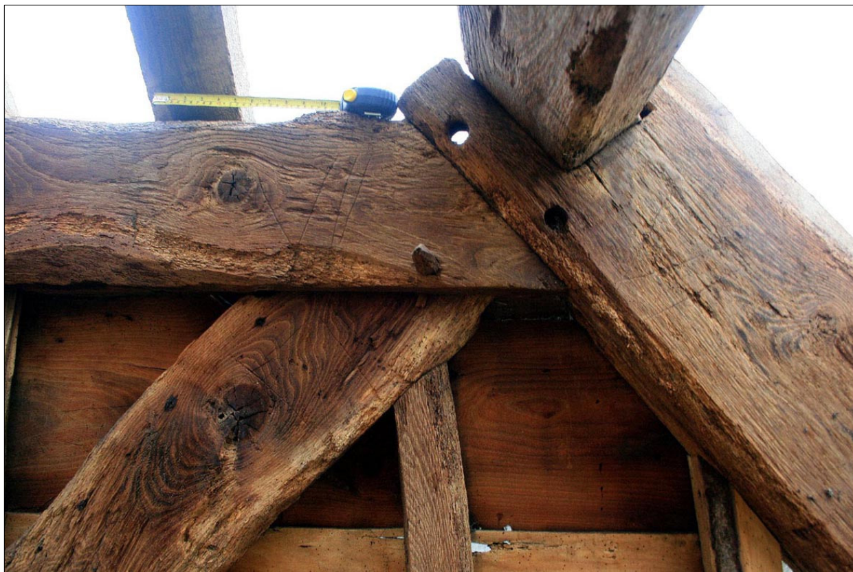
Fig.41. Bay 6, truss 6. Principal rafter-collar beam joint, with medieval carpenter's numerals. Facing east.
