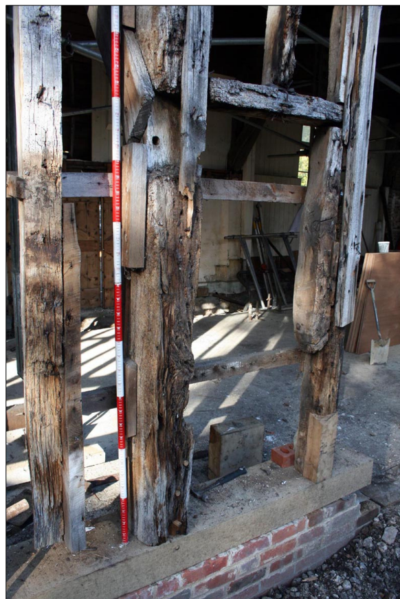
Fig.19. Cross-frame 3,(S). Principal post (centre) and Phase 2 storey posts, set upon new sill. Facing north-east.
