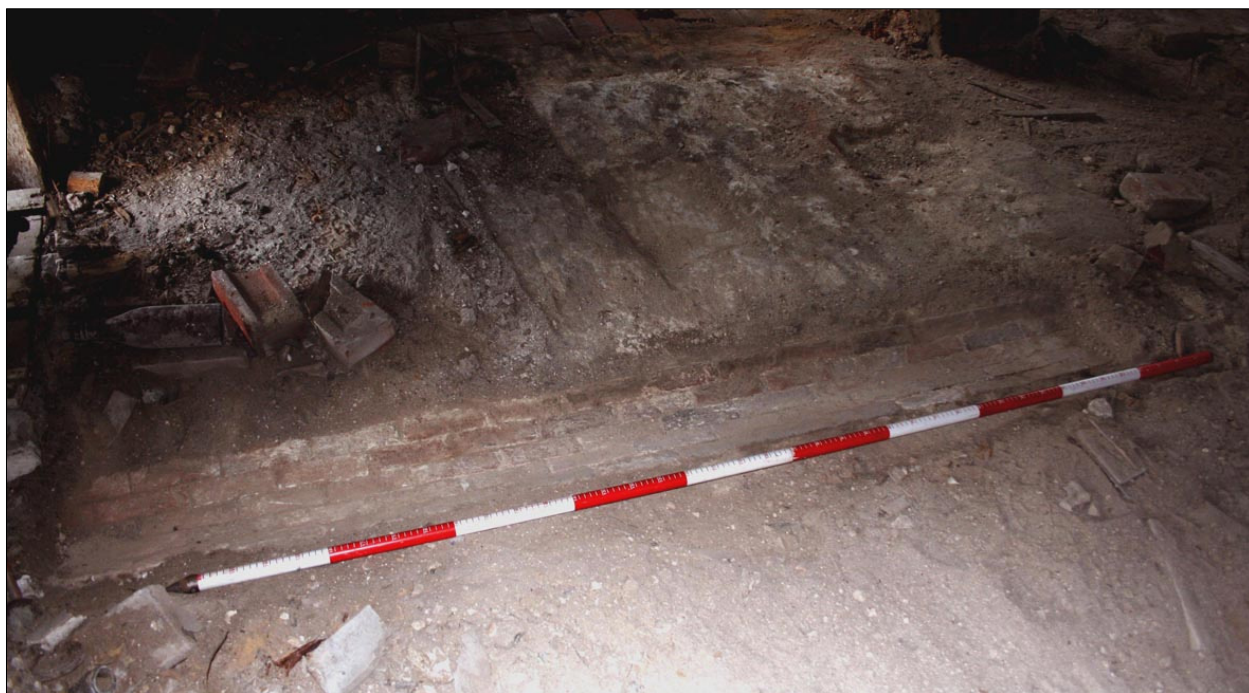
Fig. 30. Bay 4. Brick-lined drain running north-south, and beneath the north and south walls of the barn. Facing north-west.
