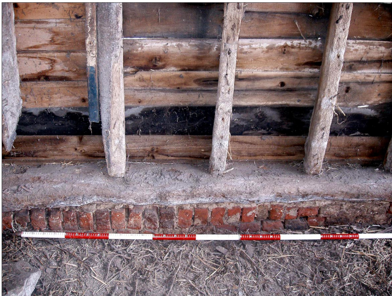
Fig.39. Bay 5, cross-frame 6. Phase 1 sill on Phase 2 brick plinth.
