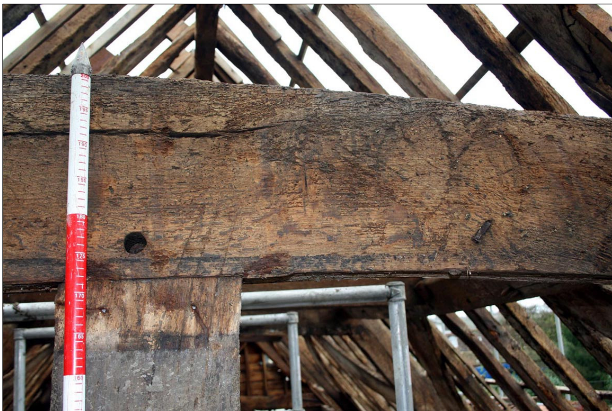
Fig.23. Bay 2, truss 3, facing side. Crown post-collar beam joint, with medieval carpenter's numerals and 'daisy wheel'. Facing east.
