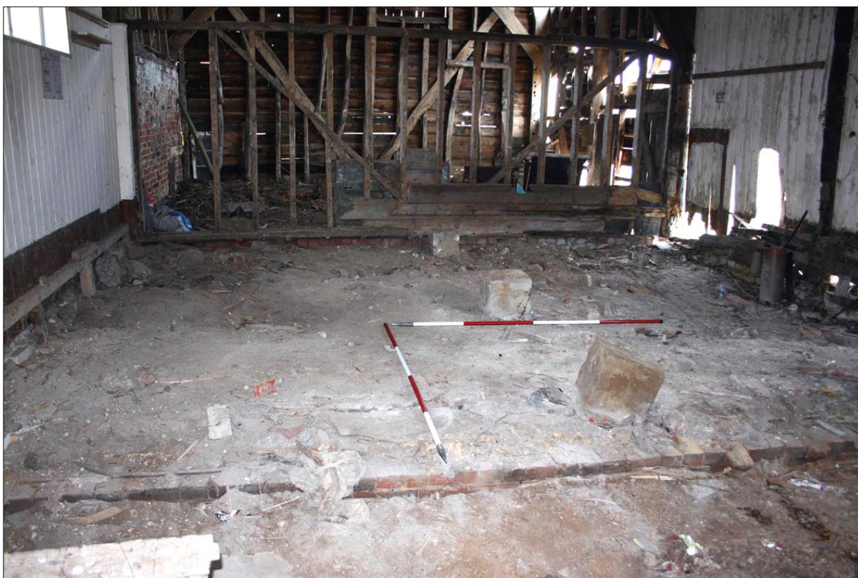
Fig.29. Bay 4. Floor of rammed chalk forming a raised area, revealed after the removal of the village hall stage. Facing east.
