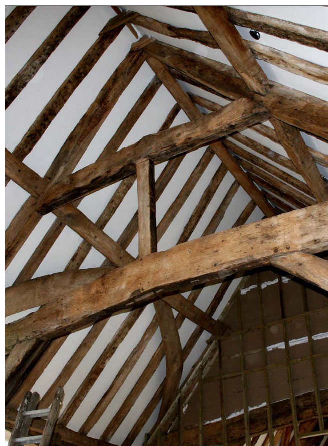
Fig.34. Bay 4, truss 5. Stave holes on the underside of the tie beam. Facing south-west.
