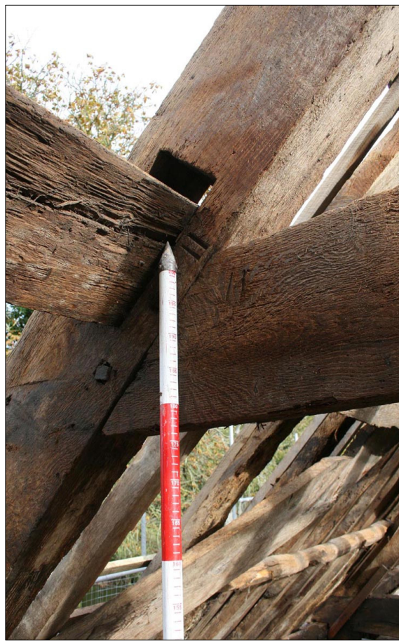
Fig.16. Bay 1, Truss 2 (N). Collar beam-principal rafter joint. Facing north-east.
