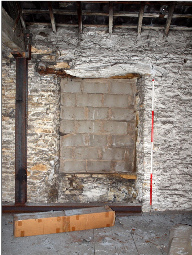
Plate 36: Detail of blocked window in west wall with hand cut timber lintel
