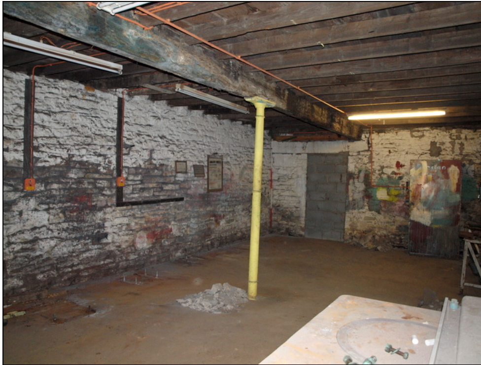
Plate 12: Basement showing blocked doorway with large lintel and inserted cast iron stanchion
