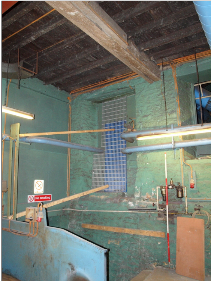
Plate 16: Doorway inserted into original window opening and then blocked above basement staircase
