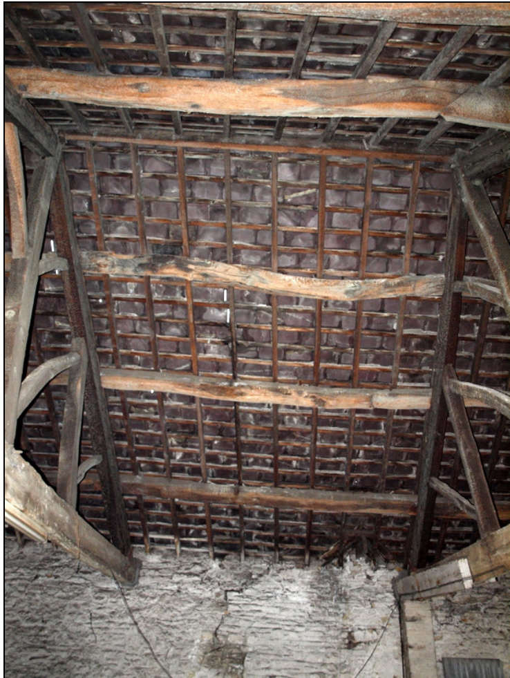
Plate 40: Detail of hand cut timber purlins
