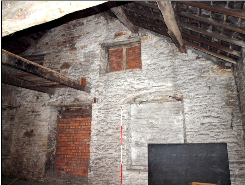
Plate 34: South wall of second floor showing blocked openings, two light stone mullions and timber platform
