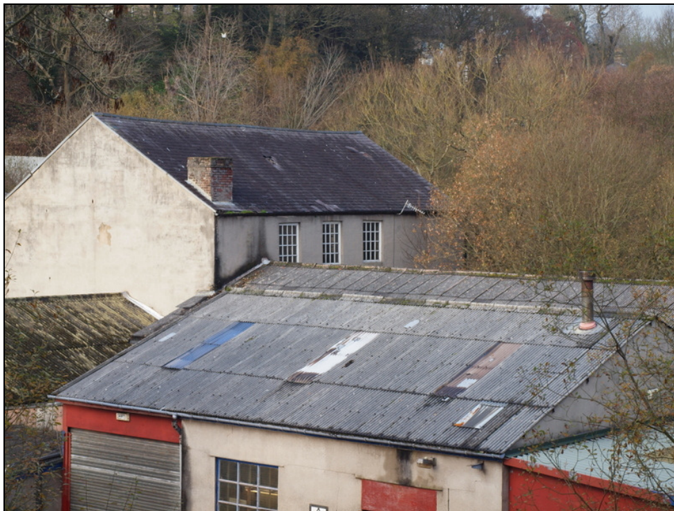
Plate 11: Second floor level east elevation, showing replaced slate roof.
