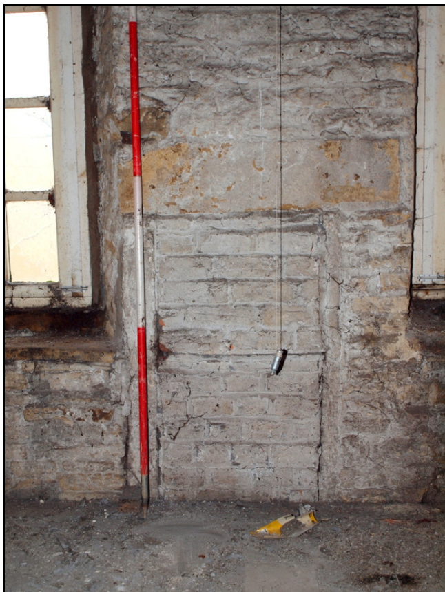
Plate 37: Detail of blocked opening in centre of north wall
