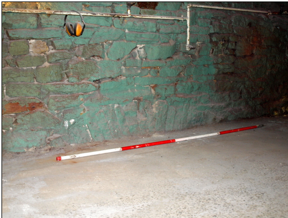
Plate 17: Arched stone lintel emerging from concrete floor in east wall
