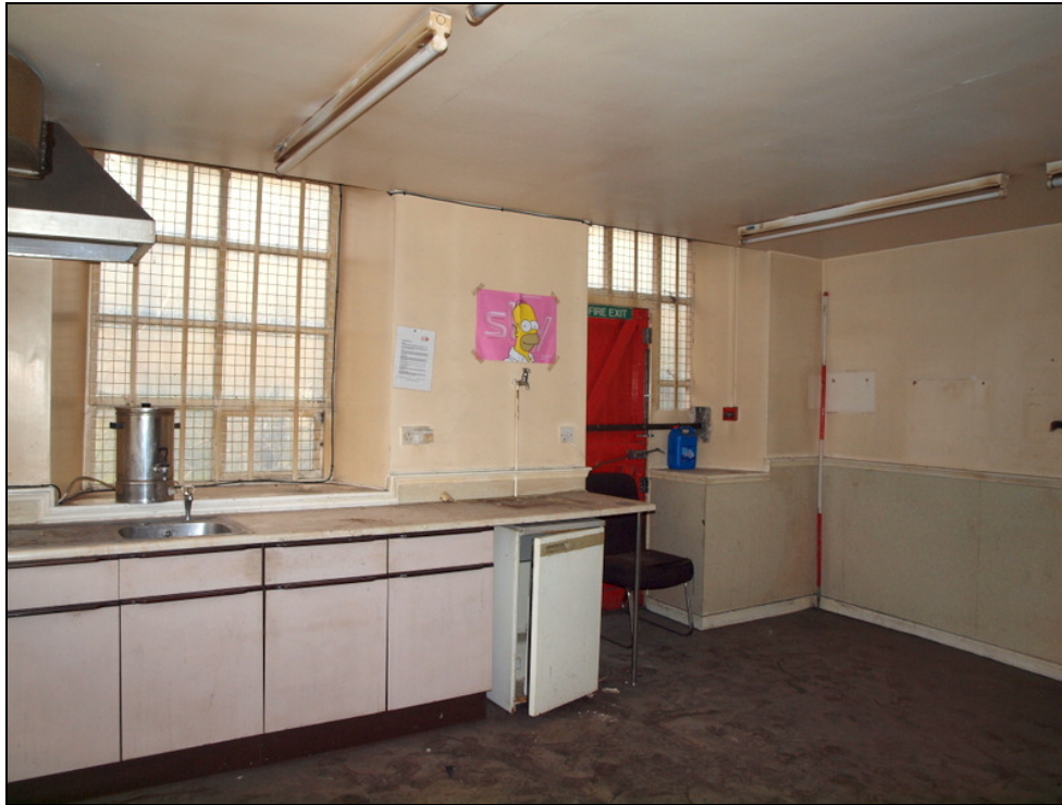
Plate 20: Ground floor kitchen area showing inserted fire door in window
