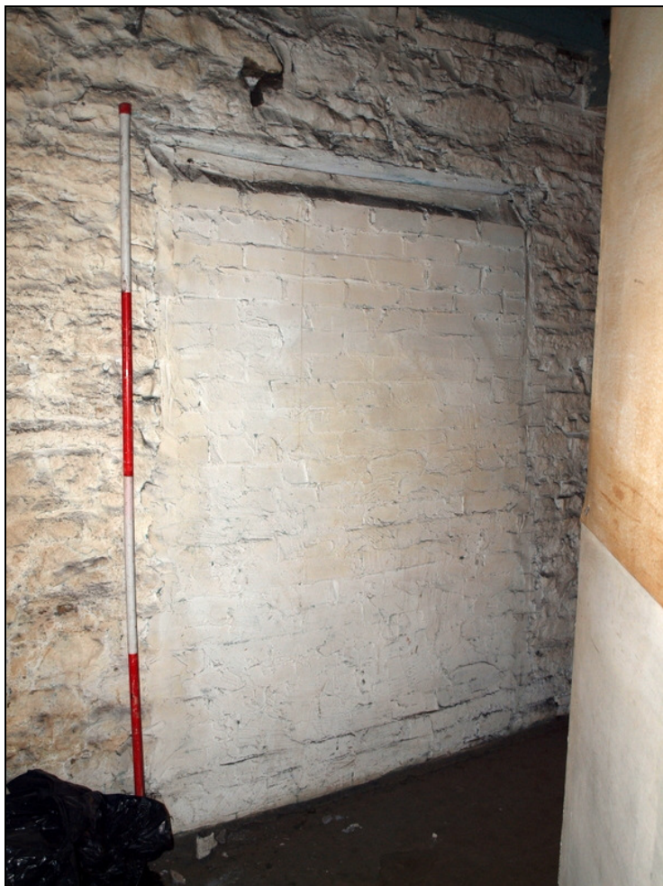
Plate 29: Blocked loading doorway in south end of west wall
