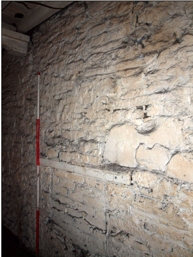
Plate 30: Blocked openings at north end of west wall.
