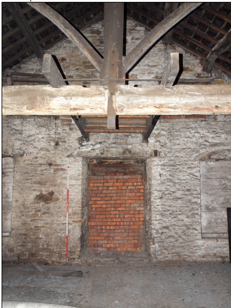
Plate 35: Detail of blocked doorway in south wall
