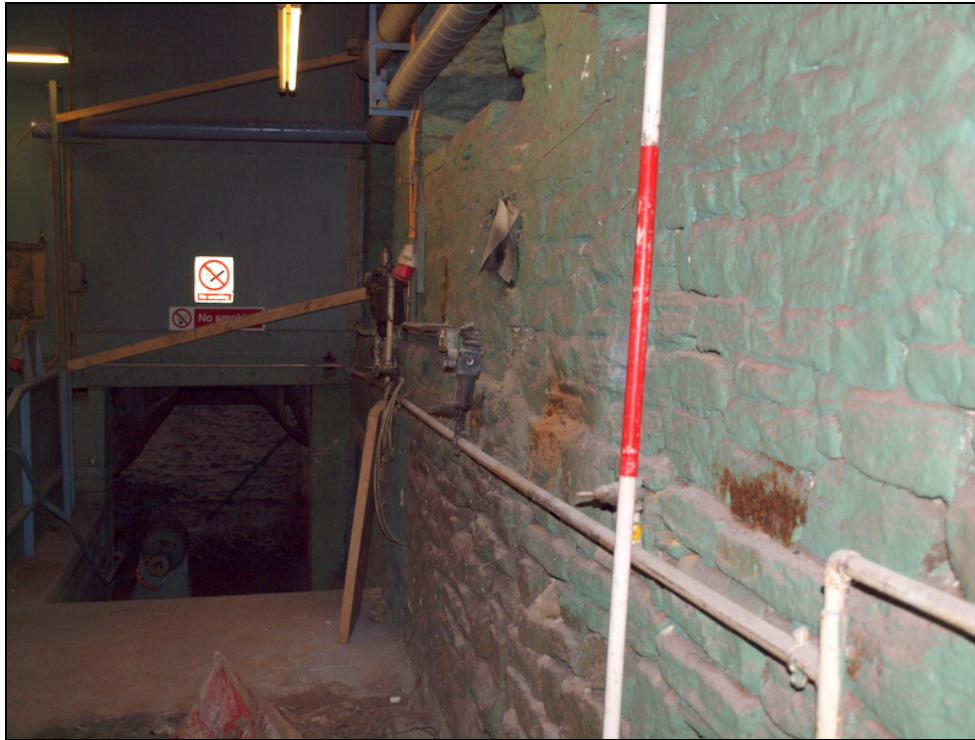
Plate 18: Slight recess in east wall showing earlier floor level
