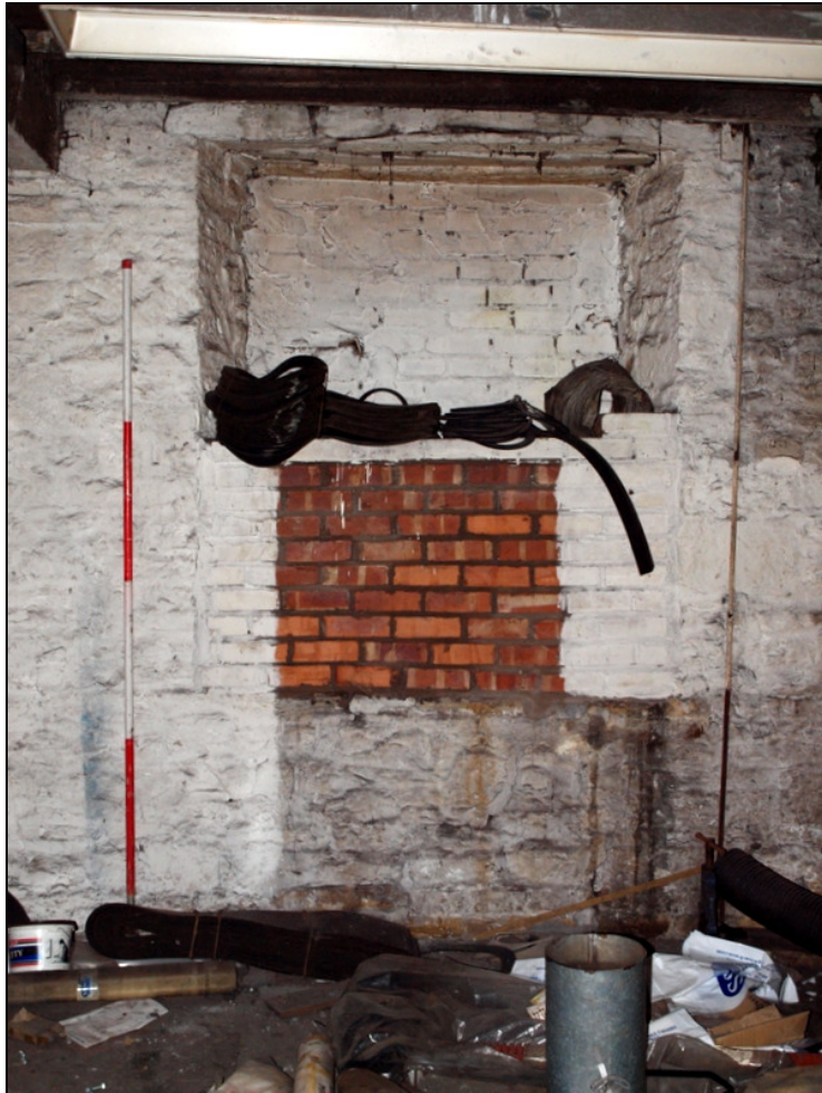
Plate 26: Blocked window in west wall bay three
