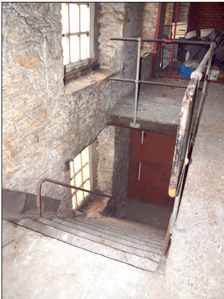
Plate 33: Inserted staircase looking down to first floor
