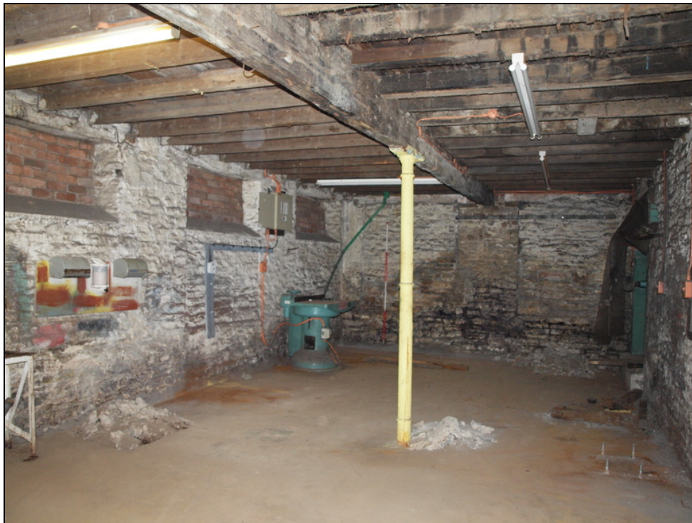
Plate 13: Basement showing twice blocked windows in north wall
