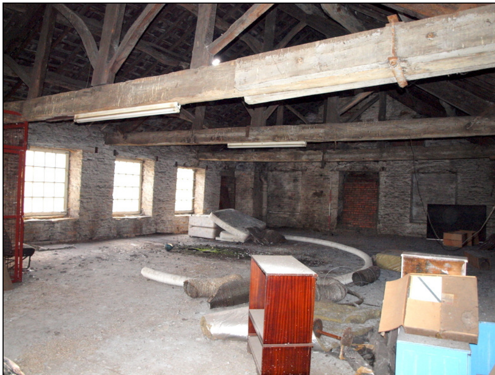
Plate 31: General view of second floor looking south showing machine-cut timber trusses.
