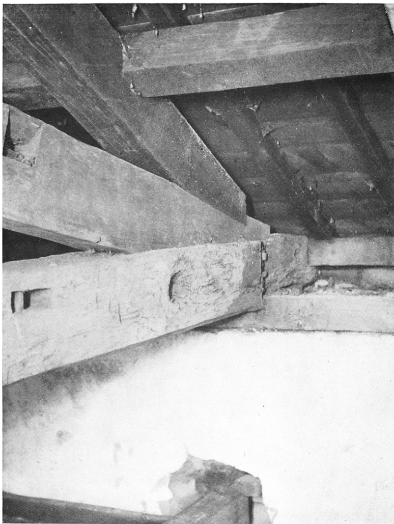
END OF PRINCIPAL RESTING ON NORTH WALL AND SHOWING NOTCHES FOR PURLIN NEAREST EAVES, HOLME CULTRAM.
