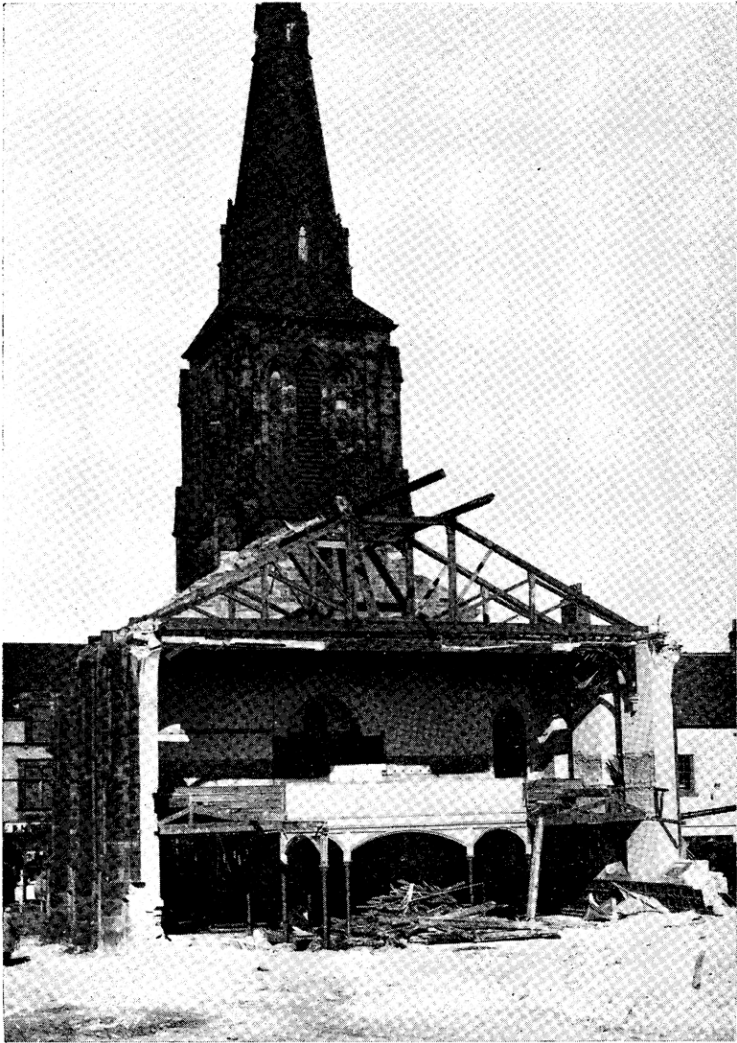
FIG. 3.—Christ Church: External view of Church during demolition.
