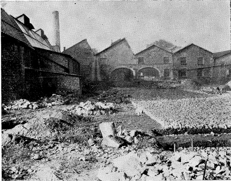
PLATE II.— Canal Head Warehouses , now Gilbert Gilkes & Gordon's Canal Iron Works , photographed from the east in 1947 from the empty (and partially filled in) canal basin. The buildings are the 1819 warehouses slightly modified. Note the two arches through which the barges passed into the covered wharfs.
