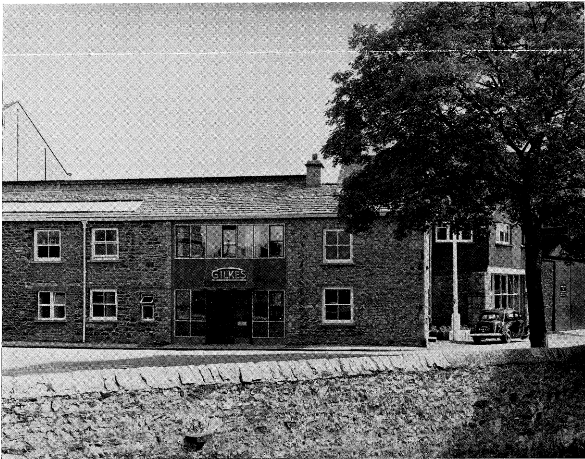
PLATE IV.—Part of Gilbert Gilkes & Gordon was office 496800168 (1056) after some modernization and tidying up. The general outline and most of the stonework is original (1819). Beams uncovered when the new entrance was built in 1956 indicate that this was the stable block.
