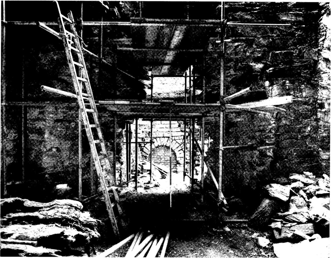
PLATE 3. Initial support system for the blowing chamber arch at Newland Furnace, early 1991. The butt-end of the original lintel beam can be seen in situ on the right hand upper corner, as can the broken remains of the beam itself (lower left). The rubble and debris had been cleared at this stage.
