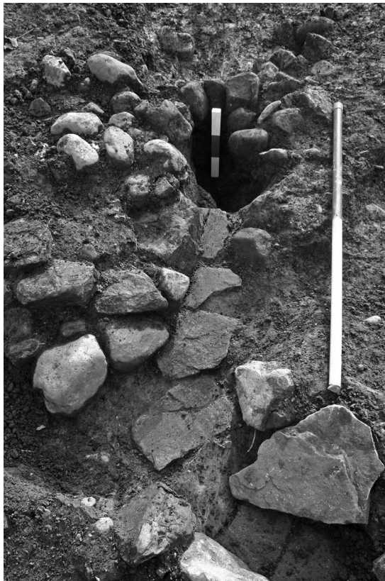
FIG. 5. Drain and sump.
