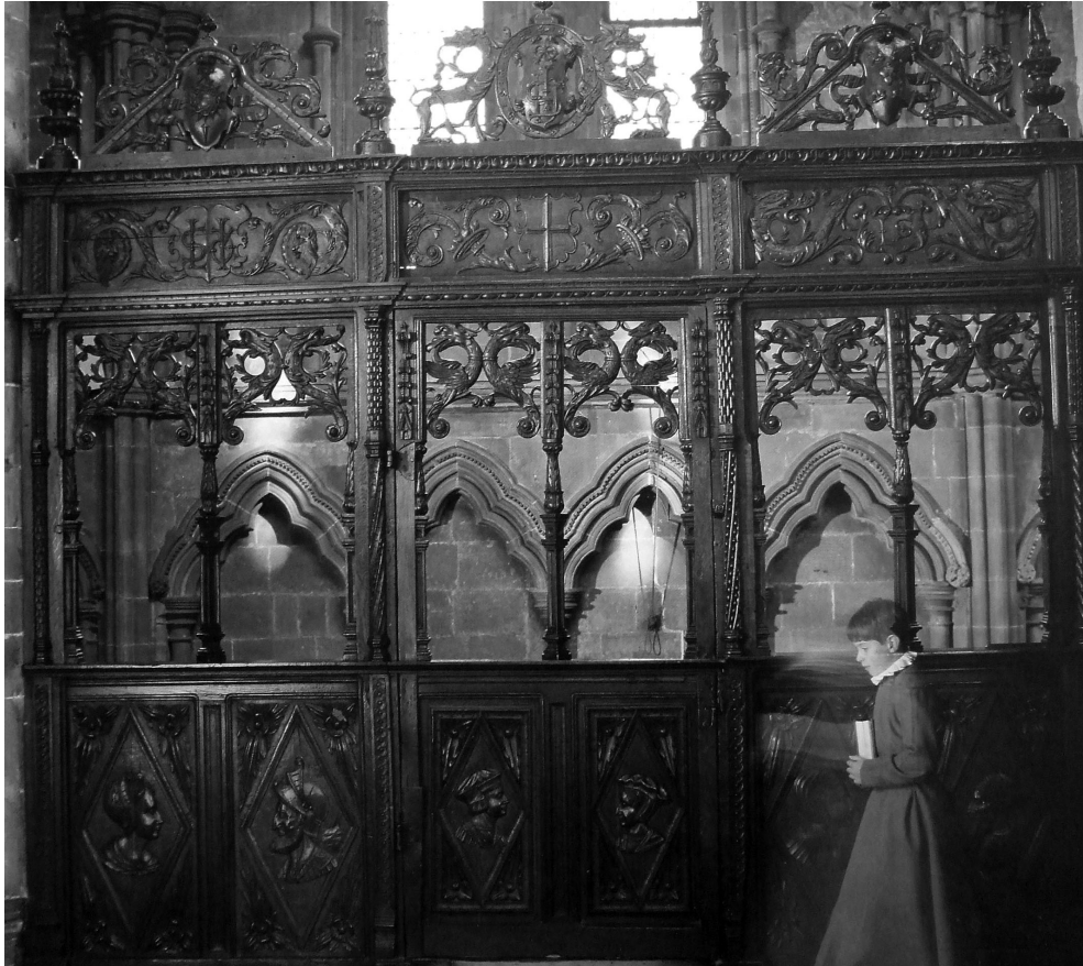
FIG. 8. The Salkeld Screen: south side
