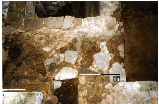
Plate 13 Church 2 wall 17/F85 abutted by Church 3 wall 17/F66 (scale 0.5m)
