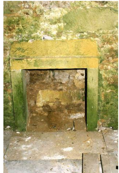
Plate 25 First-floor fireplace within laird's loft
