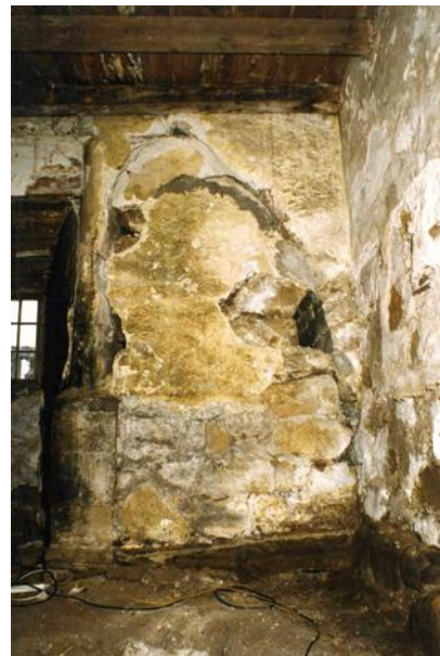
Plate 26 North column 23/C1120 with blocking 23/C1121 and plaster over 23/C1124
