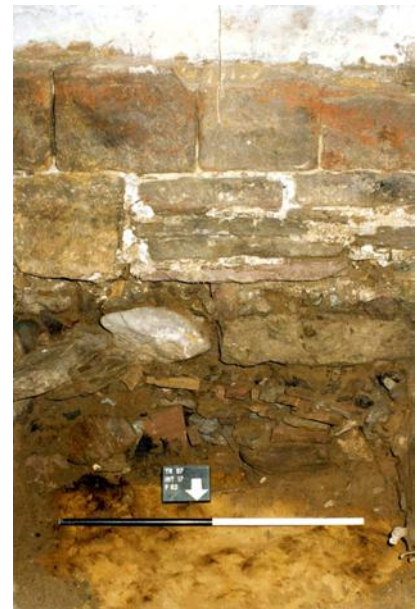
Plate 8 Church 2 south wall foundation and elevation 17/F62 and F63 (scale 1.0m)
