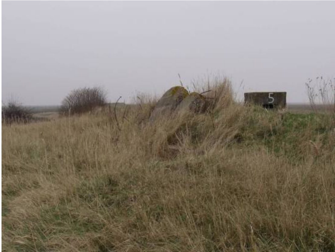
Plate 5: Observation point (Asset 169) and demolition material (Asset 168), North Site, Section 1
