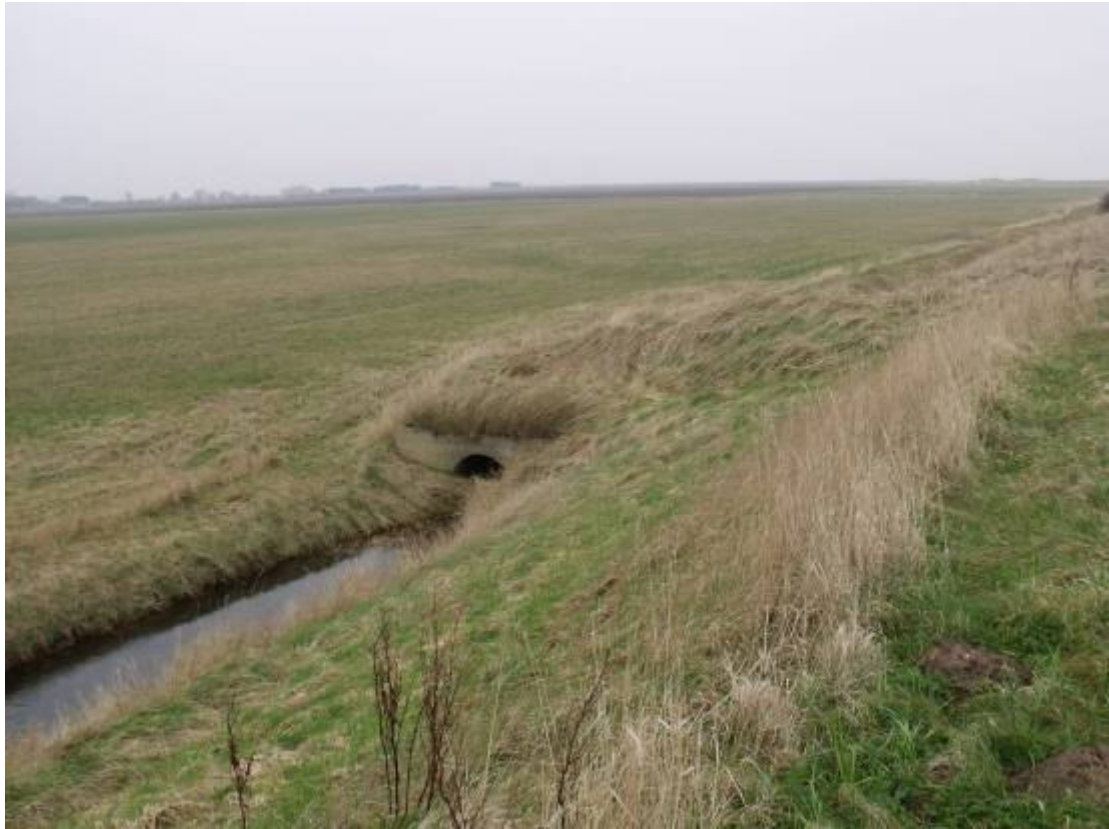
Plate 15: Causeway (Asset 172), North Site, Section 1
