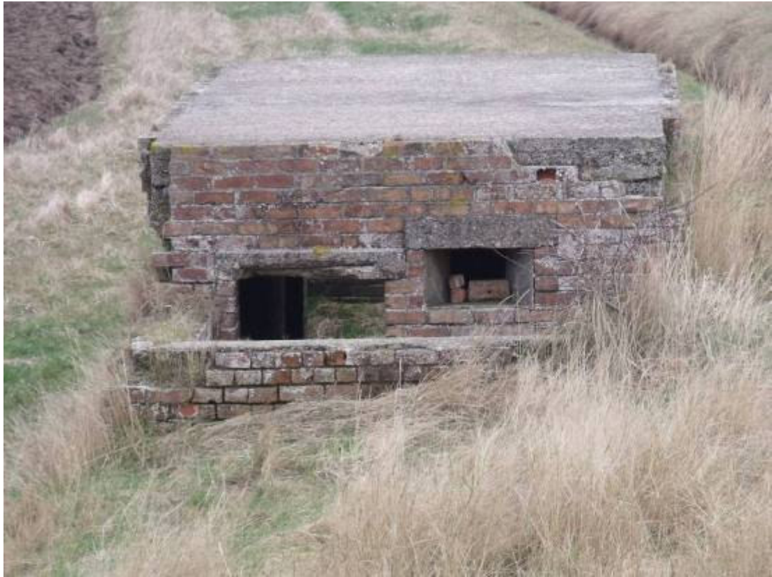
Plate 13: Possible infantry blockhouse (Asset 167), North Site, Section 1
