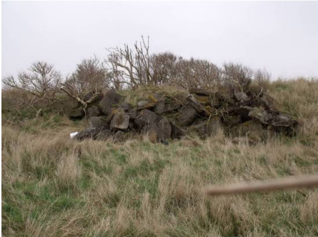
Plate 17: Demolition material (Asset 191), North Site, Section 1
