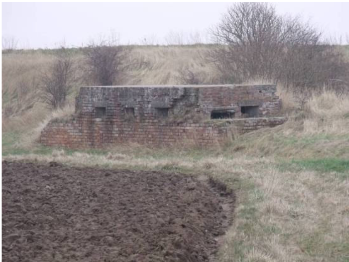
Plate 12: Possible infantry blockhouse (Asset 167), North Site, Section 1
