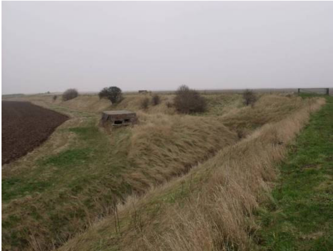
Plate 11: Possible infantry blockhouse (Asset 167), North Site, Section 1
