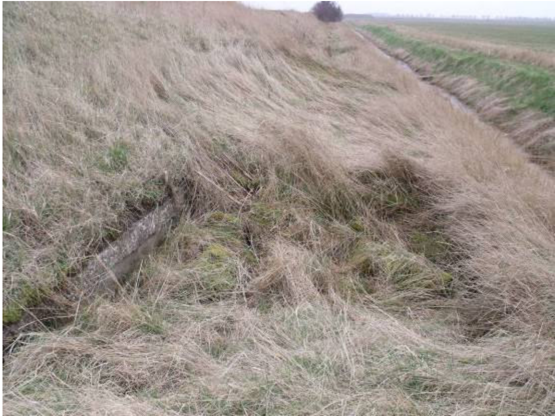
Plate 9: Collapsed structure (Asset 182), North Site, Section 1
