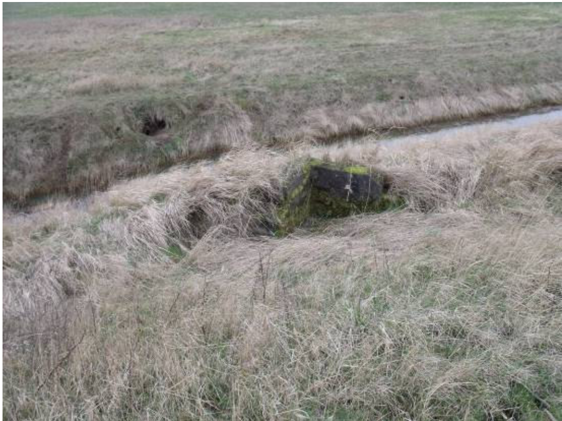
Plate 16: Causeway (Asset 189), North Site, Section 1
