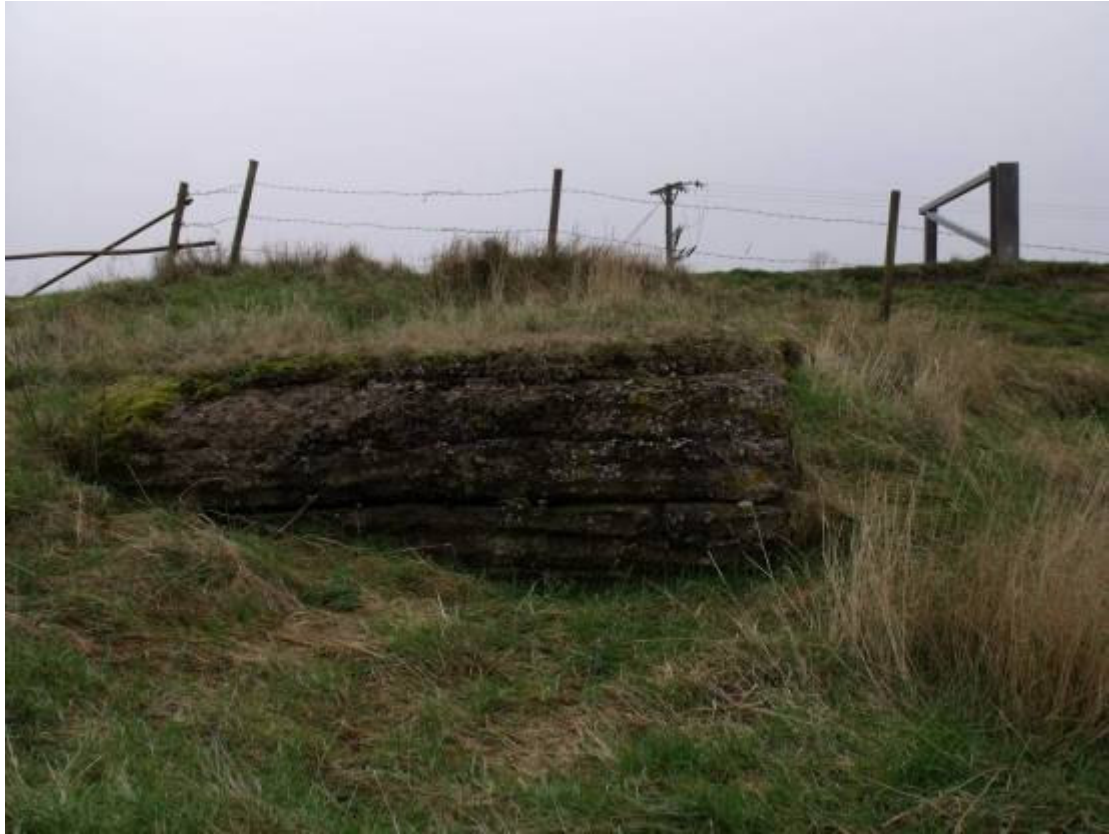
Plate 7: Concrete pad (Asset 138), North Site, Section 2
