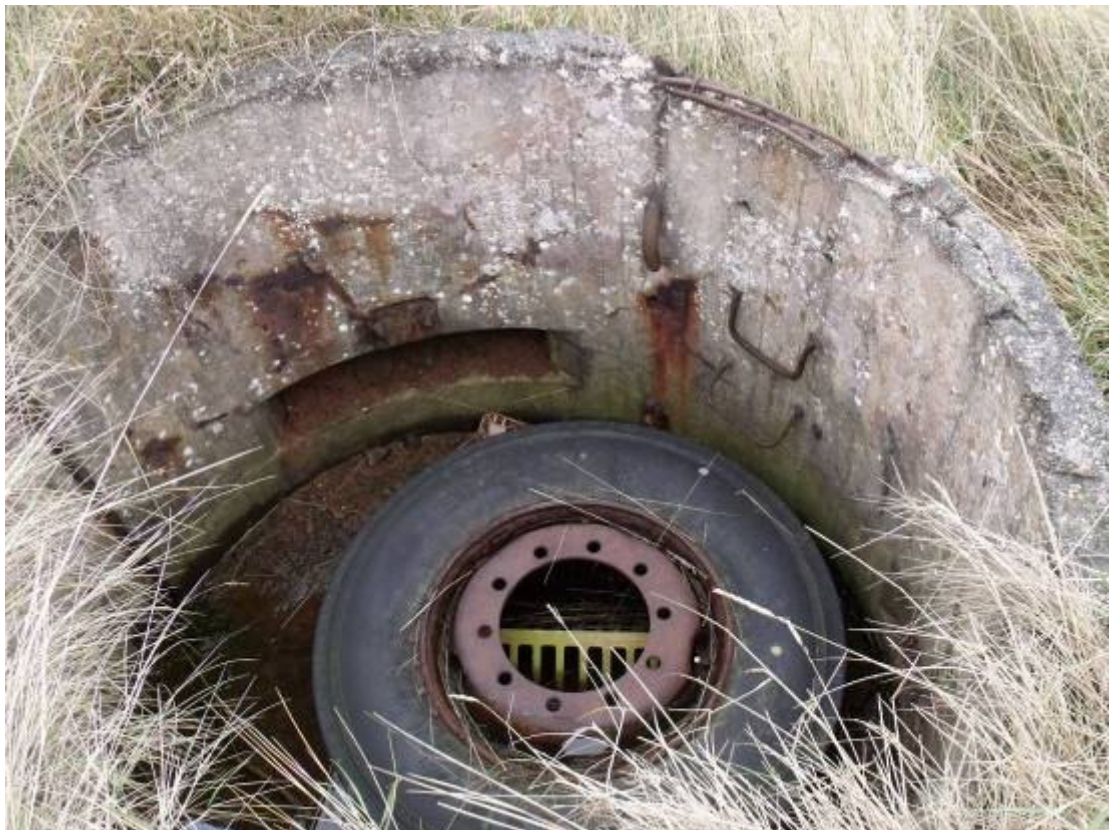
Plate 10: Semi-sunken 'turret' feature (Asset 190), North Site, Section 1
