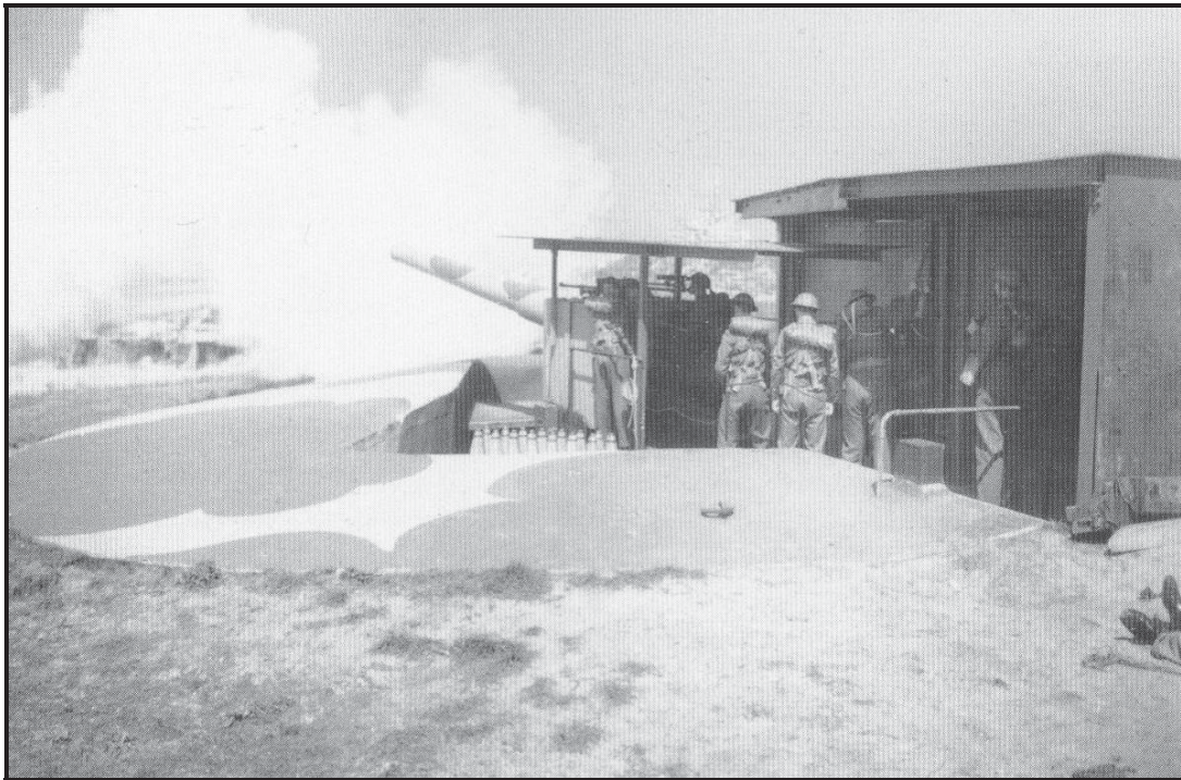
Fig.7 – 6-inch gun at Fort Crosby being fired. Though not an ECB the position has been modified to provide overhead protection and carries a shield (Lowry: 2004).
