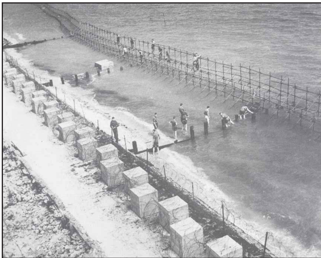
Fig 6 – The erection of scaffolding poles in addition to AT cubes and barbed wire (Wills: 1985).
