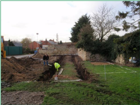
Plate 8: Work in progress, from the east
