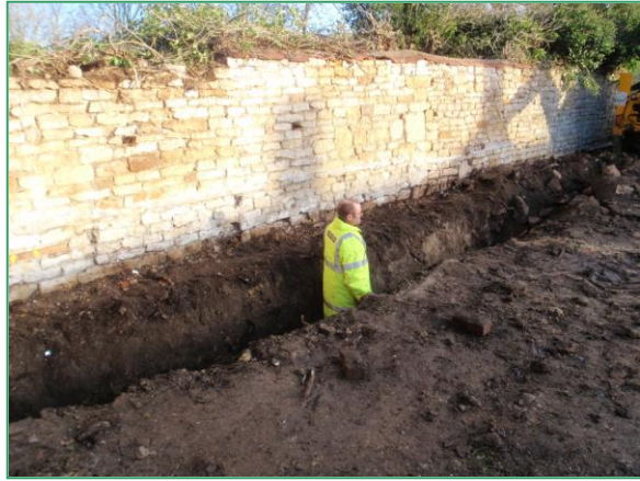
Plate 2: Work in progress, from the south-west
