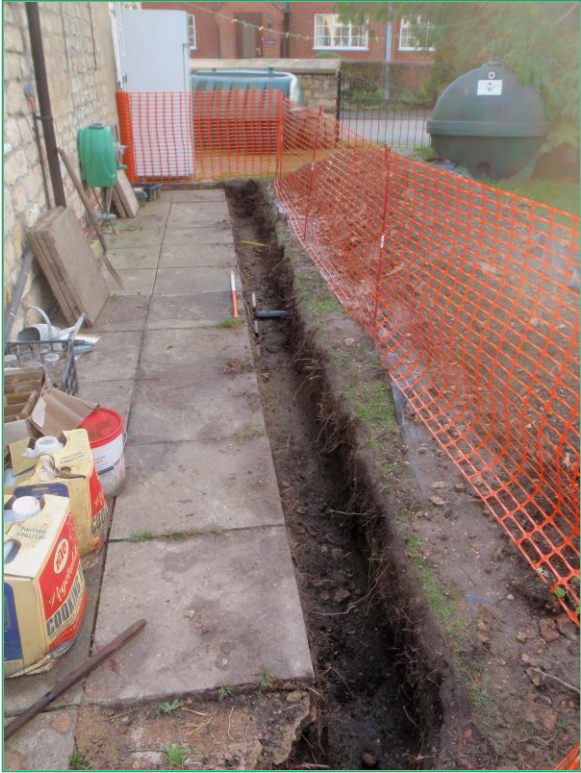
Plate 16: Service Trench, from the north
