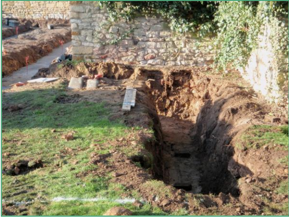
Plate 12: Work in progress, from the east
