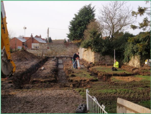
Plate 14: Completed foundation excavations, from the east
