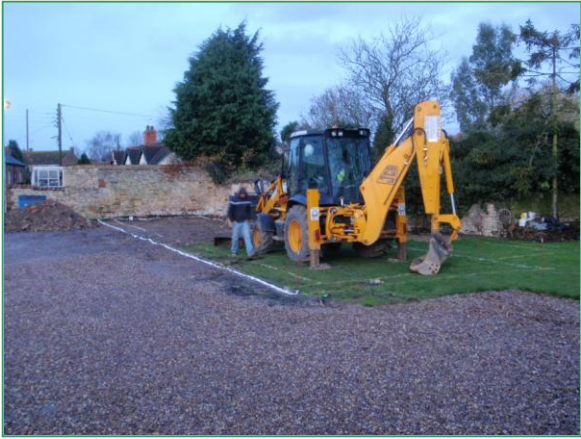
Plate 1: Pre-excavation, from the south-east
