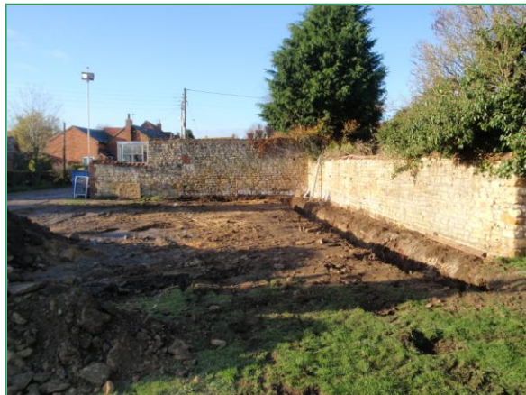
Plate 4: Work in progress, from the east
