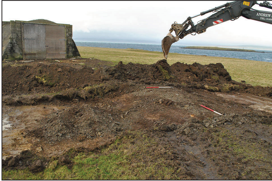
Plate 1: Area 2, showing track (103) after removal of topsoil, looking west.
