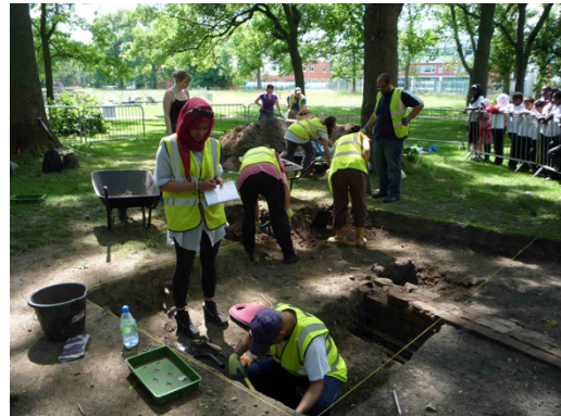
Volunteers and students digging the foundations of the band stand, 2013
