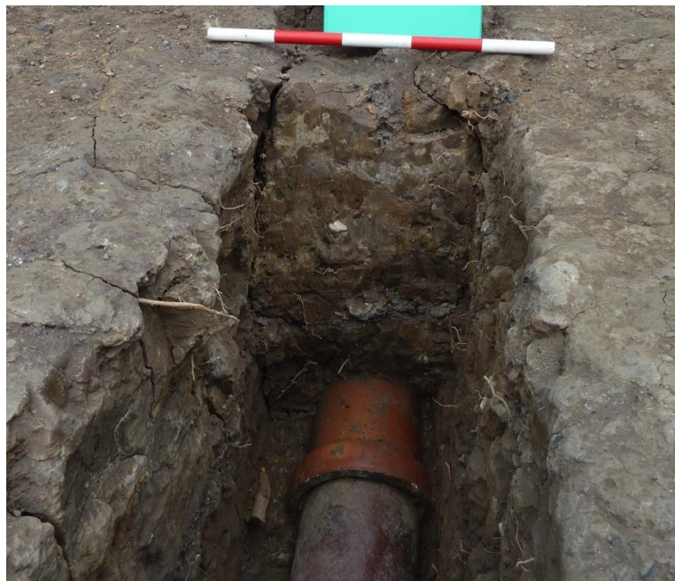
Figure 3.9: South-facing section of field drain ditch [1054]
