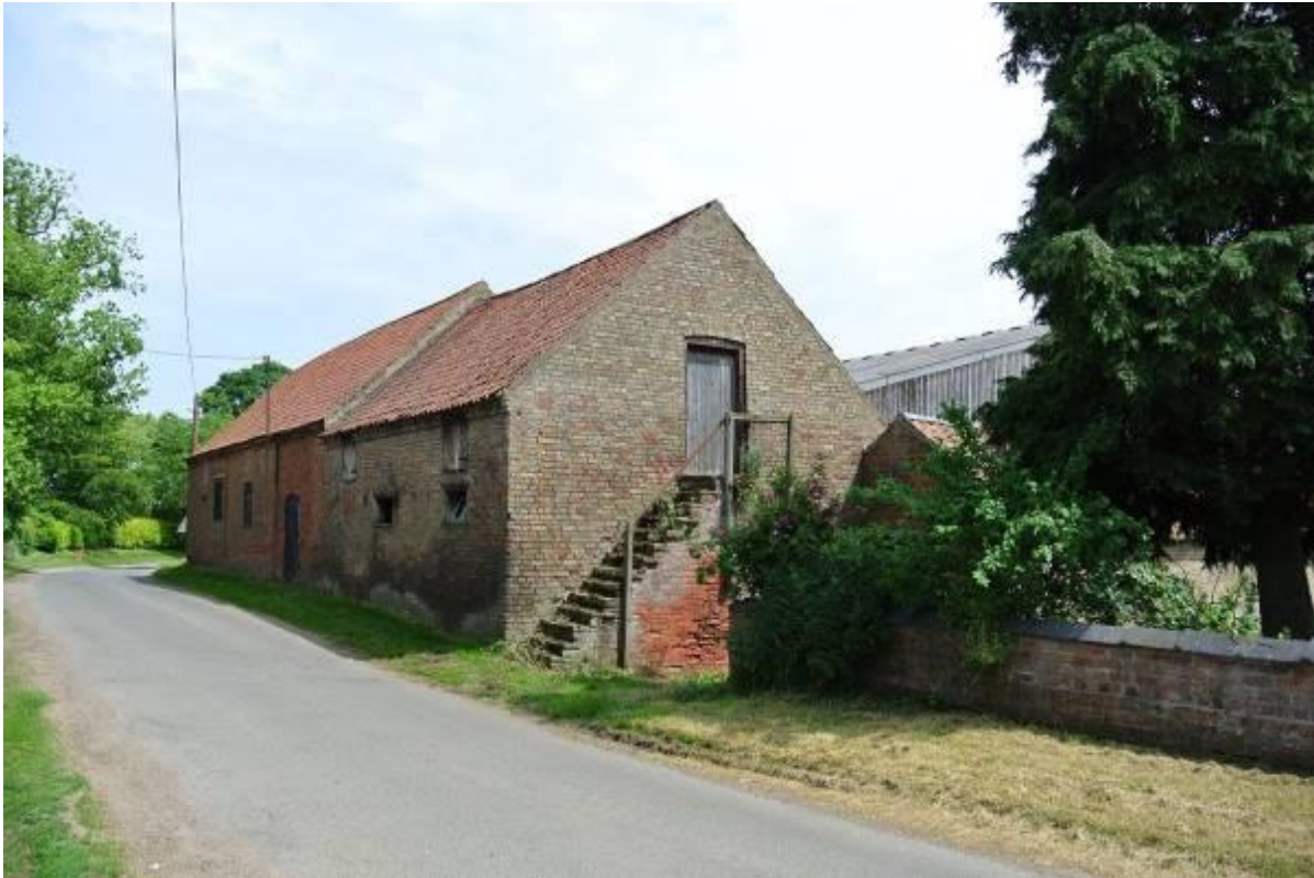
A typical central vale granary range, Toft Next Newton, constructed in brick and pantile. The development of this range is clearly visible in the change in roofline and materials, indicating a phase of expansion and improvement during the life of the building. The crew yard to the rear of the range has been covered at a later date, and may retain historic built features within its footprint
