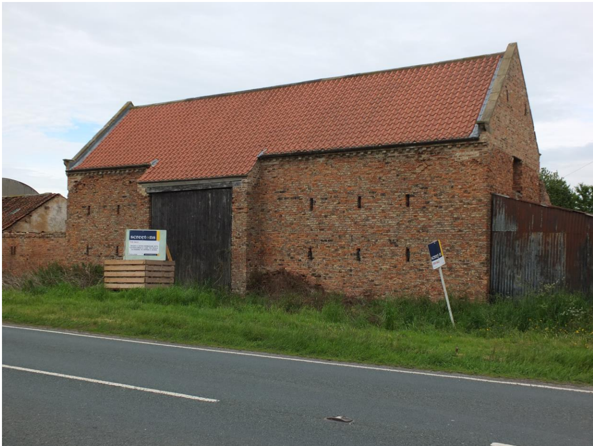
18th century roadside yard barn with porch stone kneelers and dentilled eaves. Note narrow slit air vents. (Photo © Jen Deadman)
