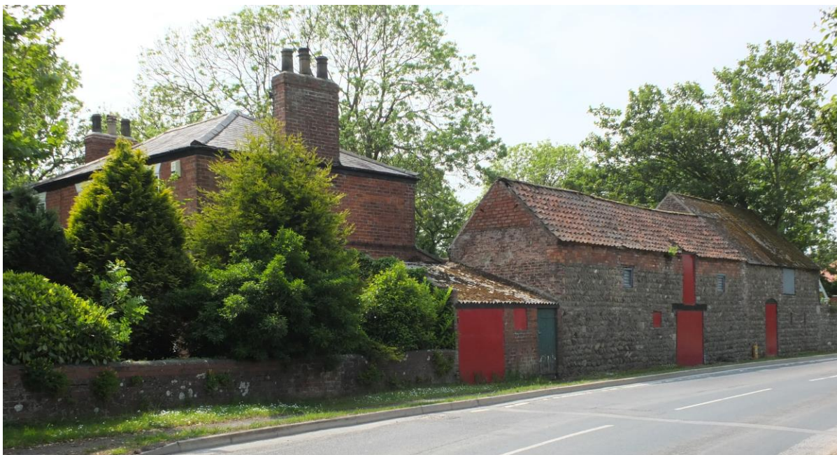
Village farm with cobble built combination and hay barn. These predate the late 19th century farmhouse with the combination barn raised in brick at a later date. (Photo © Jen Deadman)
