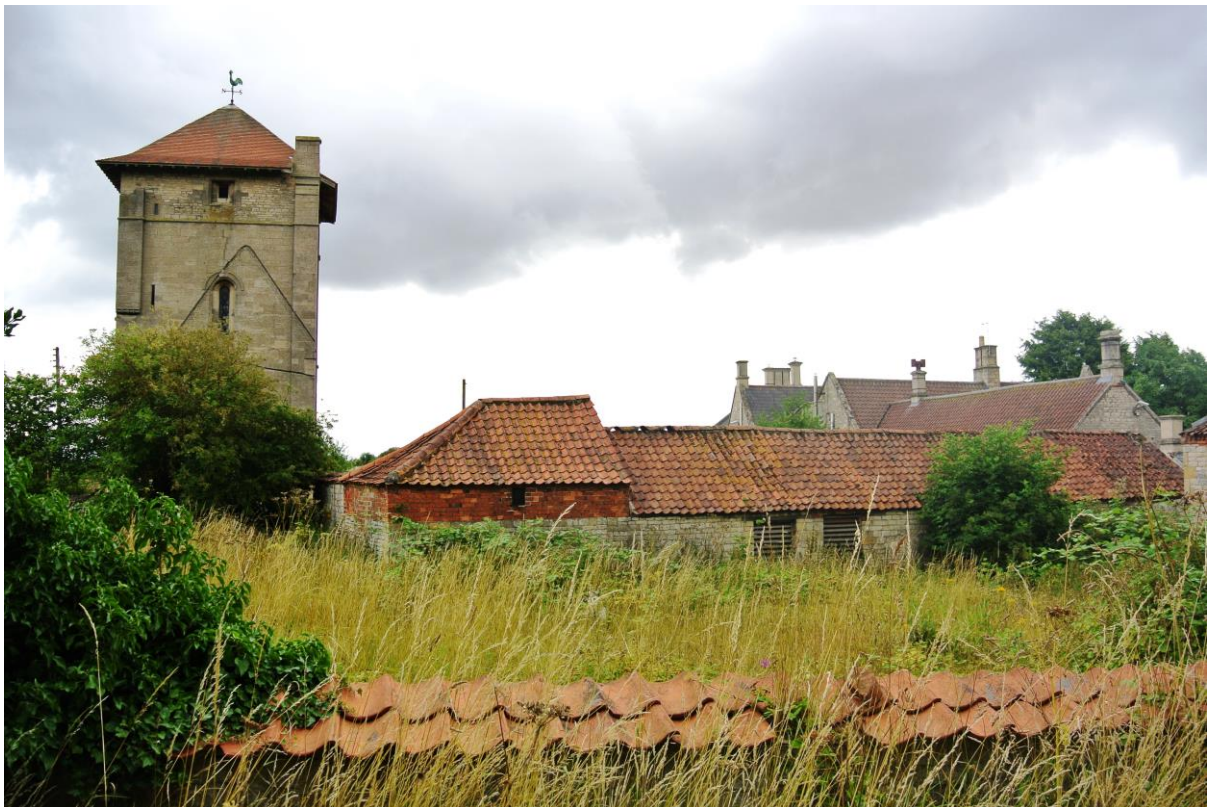
Temple Farm, Temple Bruer, near Wellingore. The present day farm is built on the site of a Templar preceptory, the tower of which can be seen above the treeline on the right of the picture. The farm buildings are constructed of the local limestone with pantile roofs and brick detailing
