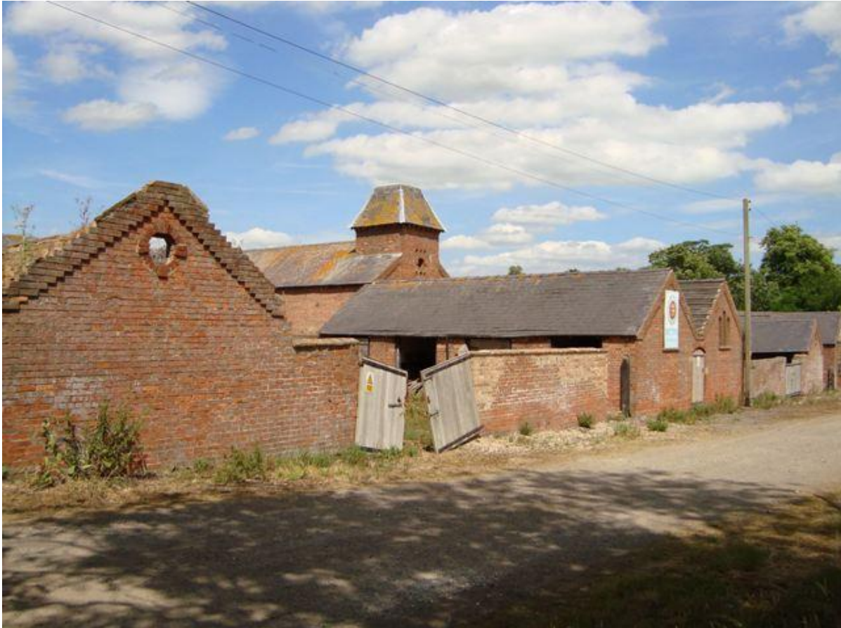
Manor Farm, Kirmond le Mire, is a very well preserved example of a planned model farmstead of the mid 19 th century. The single phase of brick and slate construction sets it apart from the more organically developed and expanded farmsteads nearby. The rigorous planning of this farmstead makes it difficult to find appropriate agricultural uses in the present day
