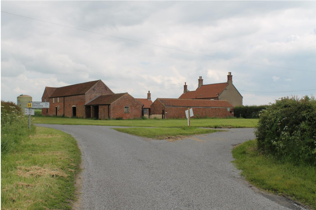
Corner Farm, Minting. A small isolated courtyard farmstead with a cartshed and combination barn facing on to the main road allowing more efficient transportation and processing of crops. The shelter shed, by contrast, faces inwards into the primary yard
