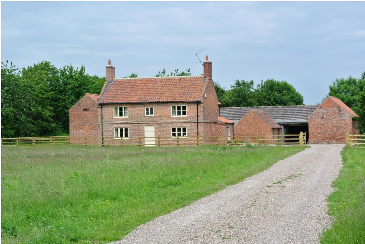
The Grange, Eagle. A regular courtyard farmstead of the early 18th century. The brick and pantile construction is typical of the area, as is the surrounding shelter-belt woodland
