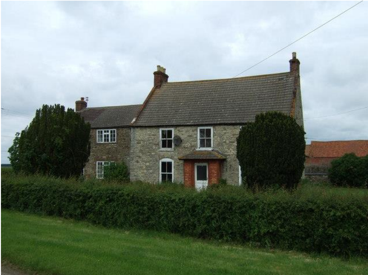
Glebe Farm, Fillingham. The farmhouse faces on to the main drove road towards the Cliff, with working buildings arranged in a regular courtyard behind. The house itself is of stone and slate, while the working buildings are of a more utilitarian brick and pantile construction. This may indicate that they post-date the farmhouse, or were constructed to show a clear difference between domestic and agricultural functions
