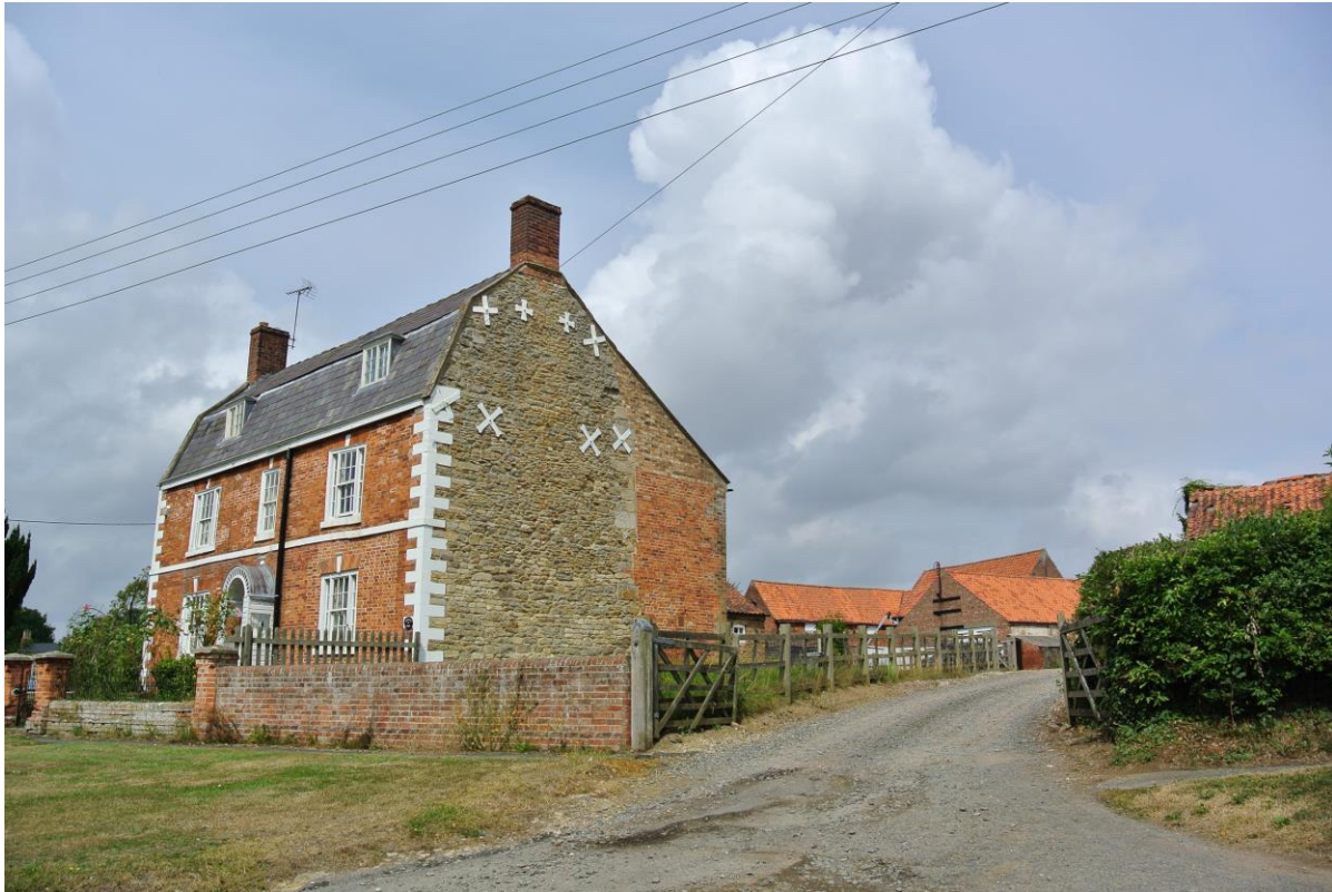
Stone built farmstead with brick facade and rear extension. A farmstead of this type reflects both the great prosperity of the area and the changes it underwent during the 18th and 19th centuries. From operating a rural economy based on the wool trade, the area became more heavily dependent on arable farming, resulting in the alteration of buildings and the construction of new outbuildings for cattle and farm equipment, as seen here to the rear of the complex. The later buildings are constructed in brick and pantile.
