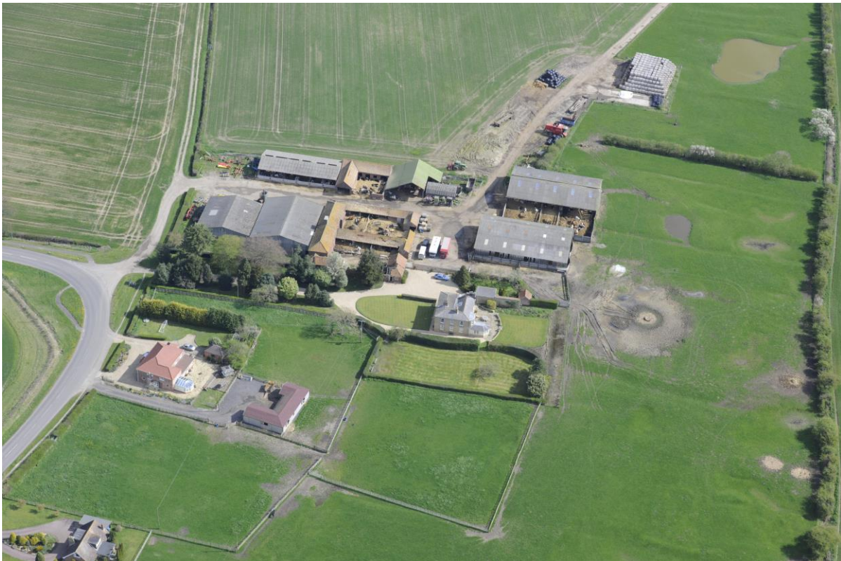
Lynwode house, a regular E-plan farmstead in the Central Vale. The farmhouse is situated at some distance from the working buildings, and presents its main aspect to the wider landscape rather than the farm itself. Although modern buildings have been added to increase the capacity of the farm, the historic shelter sheds and crew yards are still in agricultural use, demonstrating the ongoing application of mixed farming practices in the area.
