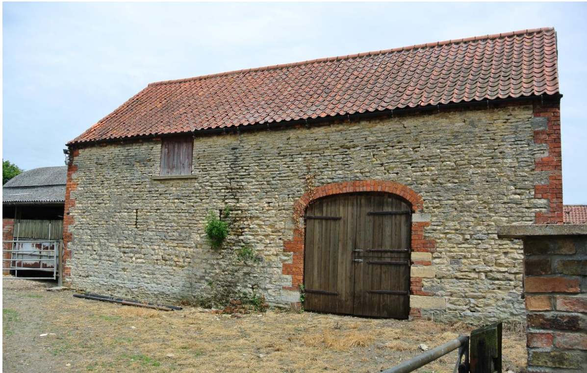
Stone built threshing barn in Saxby. Brick detailing is used to provide strength where the degraded local limestone would be unsuitable. The small window to the left of the building indicates an internal grain loft
