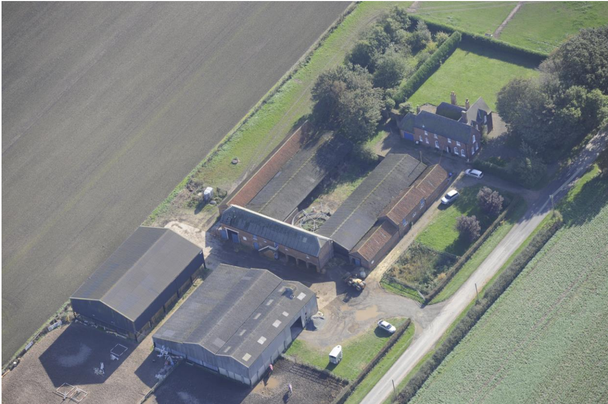
Large courtyard farmstead, showing features associated with mixed farming techniques e.g. cartsheds, barn and granary in a single range with cattle accommodation and crew yard behind.
