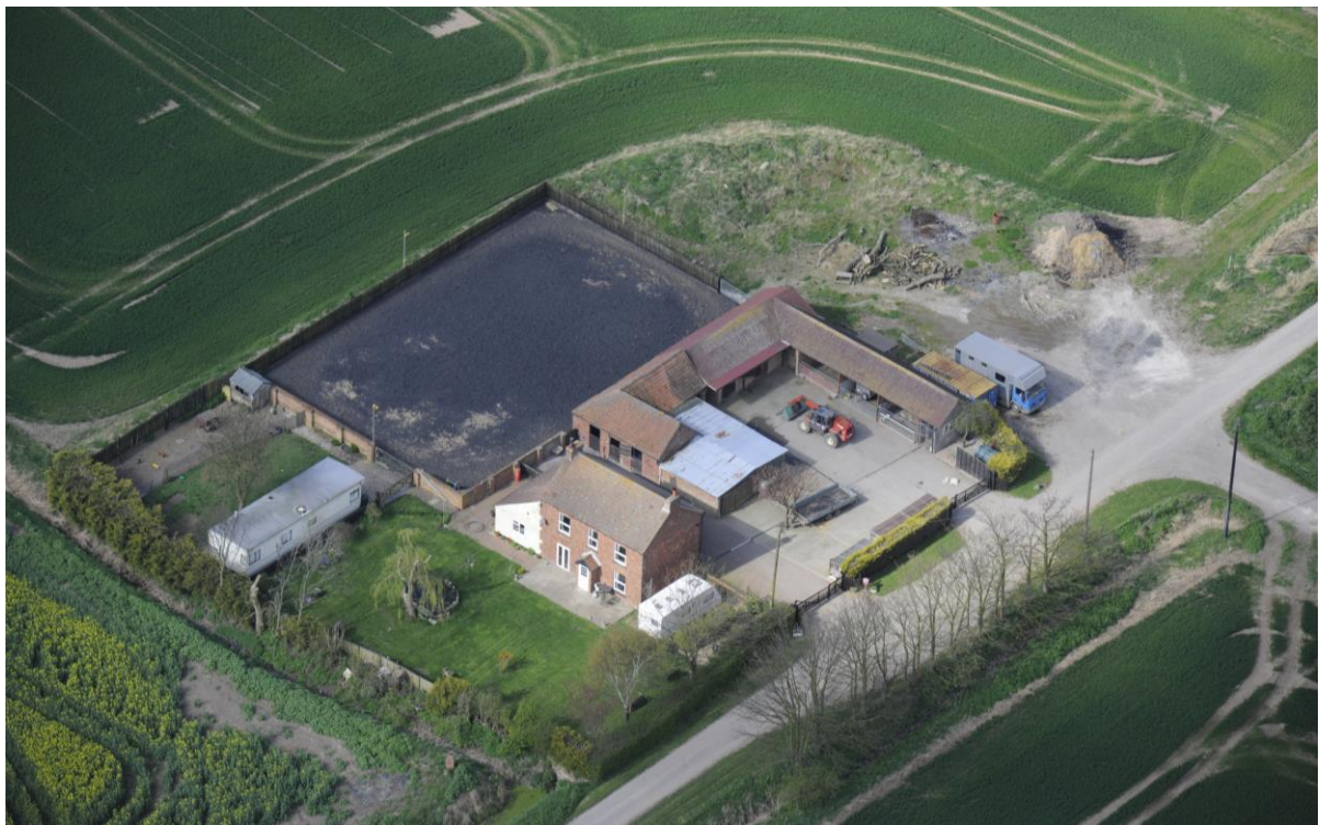
Regular L-plan courtyard farmstead, possibly extended, incorporating a barn, stables and cowsheds. There is a clear difference in the orientation of domestic and agricultural functions, with working buildings to the rear of the farmhouse facing the main access route
