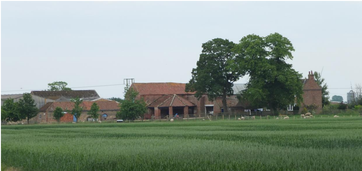
Once a common component of the yard, few horse engine sheds now remain. Evidence for them can be found occasionally in roof lines discernible on the rear walls of some barns, while some, as here, still survive. (Photo © Jen Deadman)
