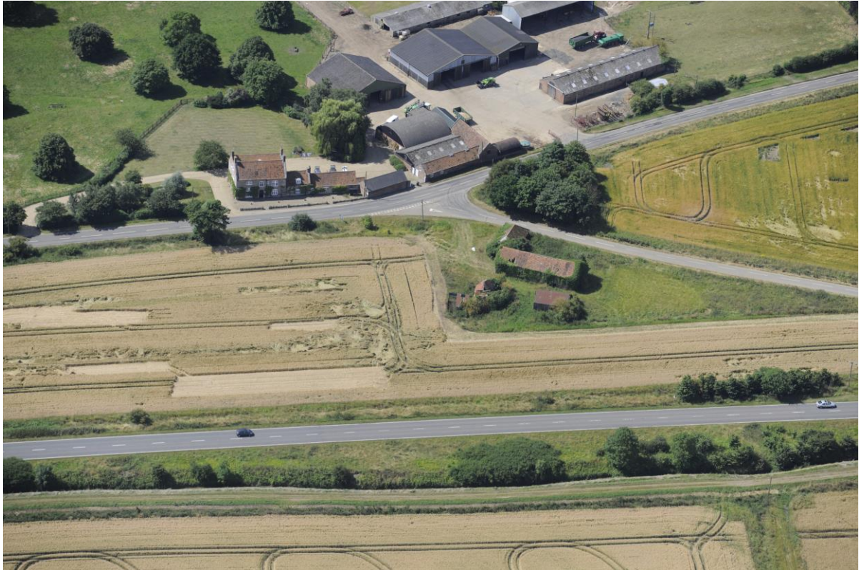
Priors Farm, Bridge End. An 18th century dispersed multi-yard complex set at one end of an ancient causeway across the western fens. The farmhouse appears to be an older linear farmstead with working buildings attached in line. Large modern buildings have been added to the complex while historic buildings typically used for housing livestock are disused
