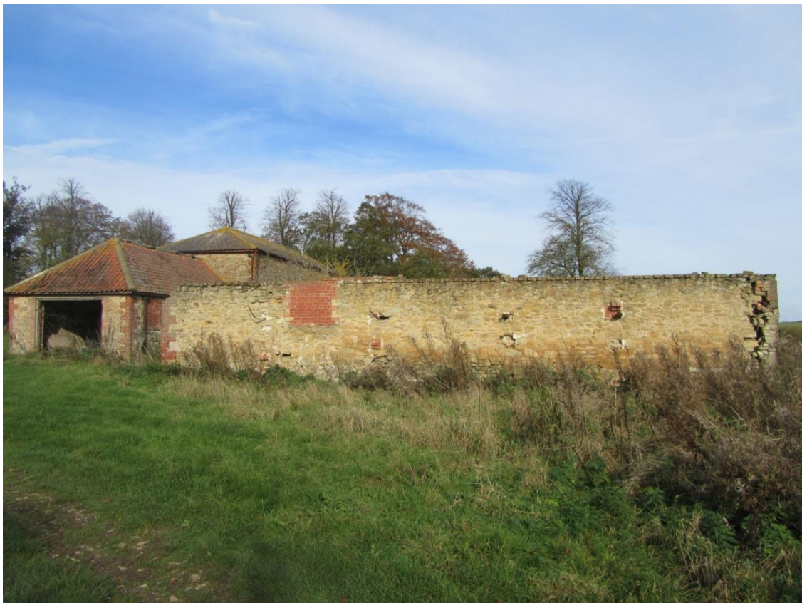
View of southern end of working buildings
