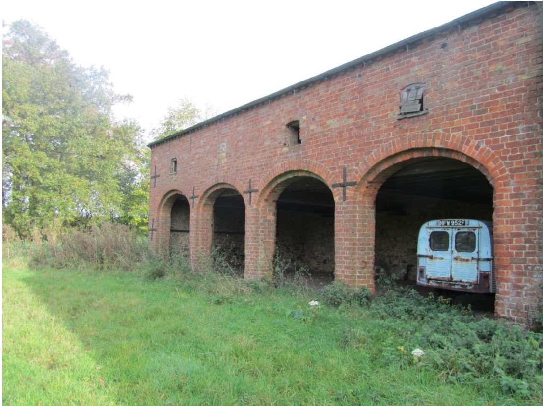
View of cart shed and granary
