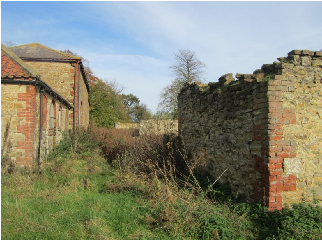
View looking north between working buildings
