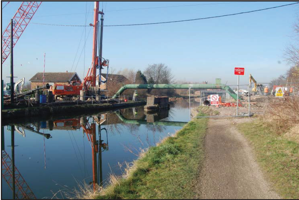
Plate 51: Watery Lane Bridge.
