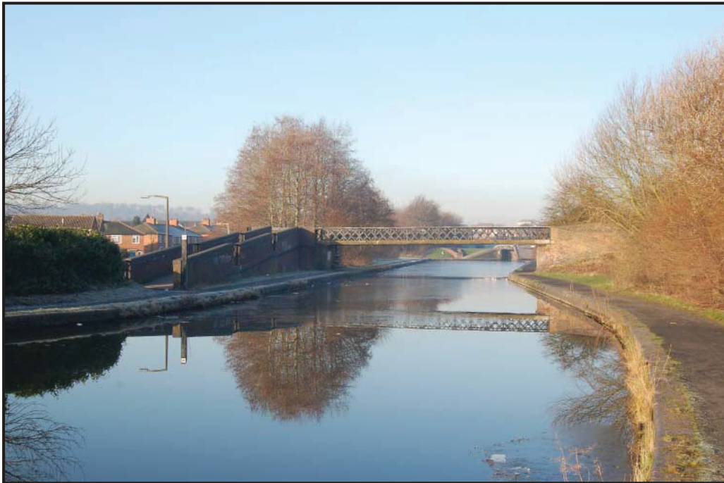
Plate 3: Wood Street Footbridge.
