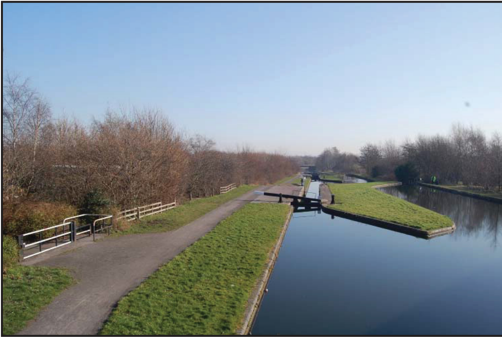
Plate 1: Factory Locks from the West.
