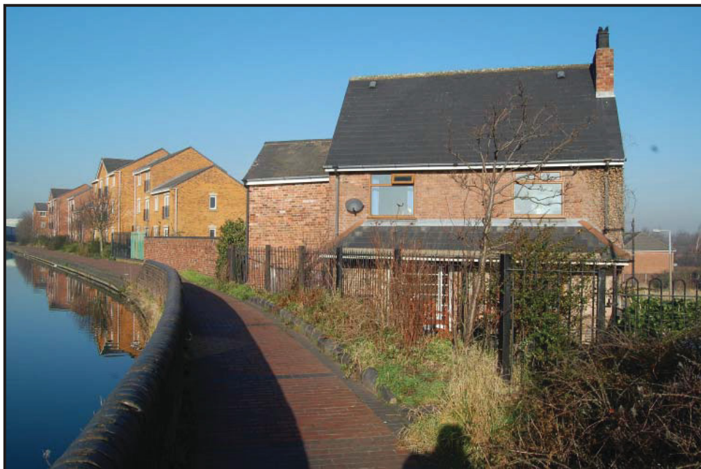
Plate 39: (19) Canalside House, Factory Road.
