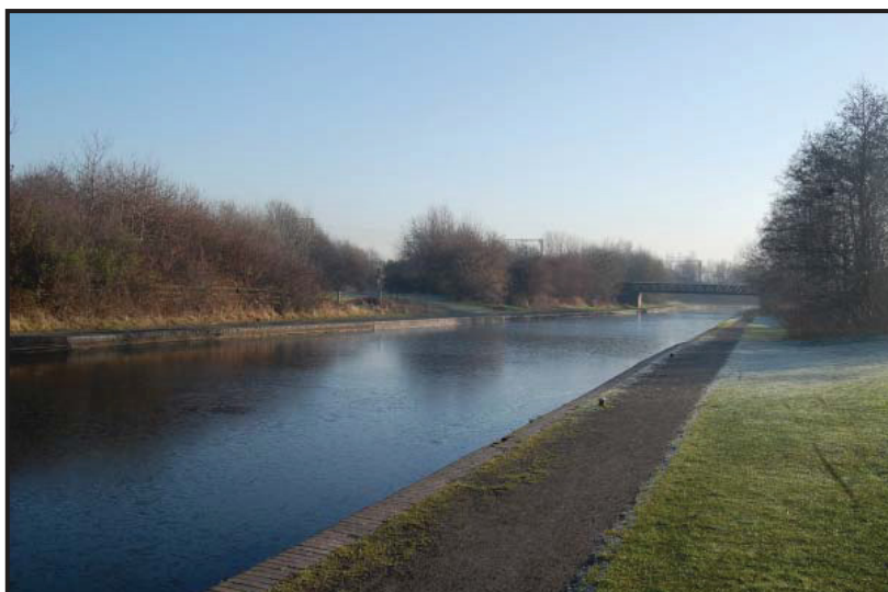
Plate 18: New Line from Waterloo Road Footbridge.
