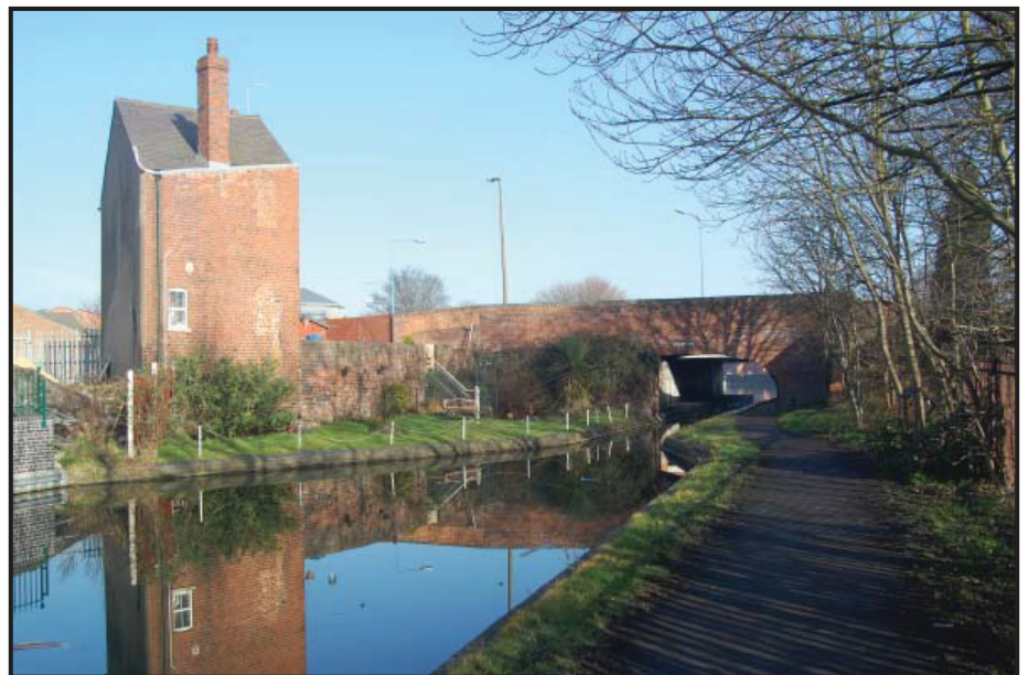
Plate 14: Tipton Green Bridge from the South.
