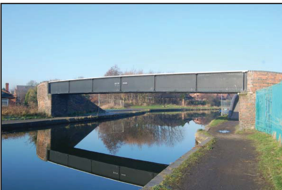
Plate 33: (16) Watery Lane Junction Roving Bridge.
