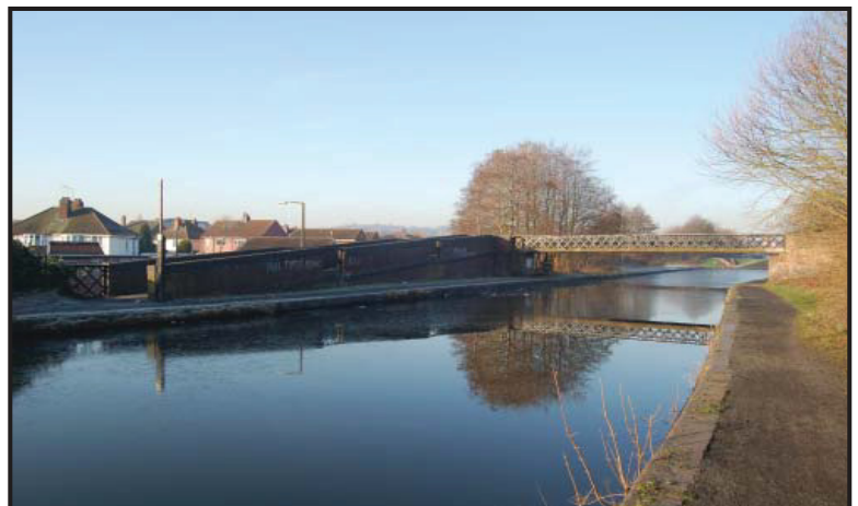
Plate 27: (1) Wood Street Footbridge.
