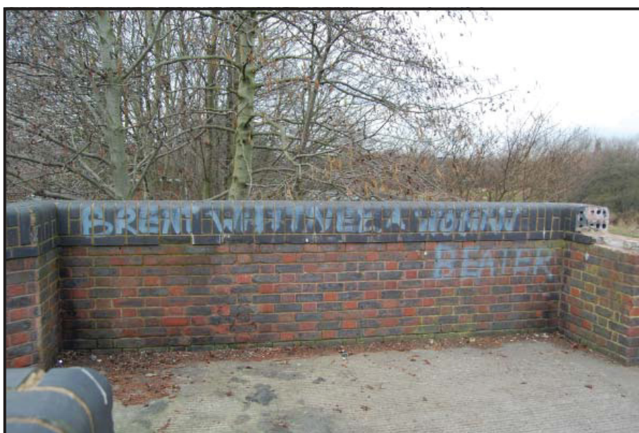
Plate 48: Wood Street Footbridge.
