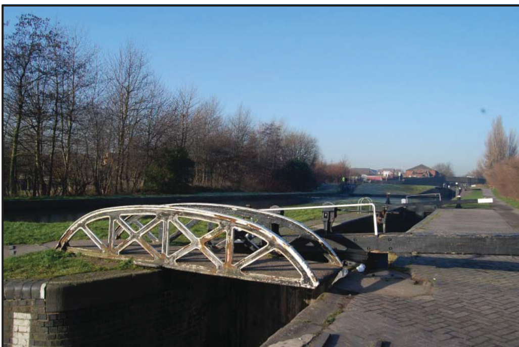
Plate 6: Cantilever Footbridge.
