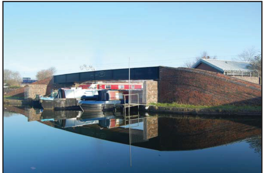
Plate 32: (15) Toll End Communication Canal Roving Bridge.
