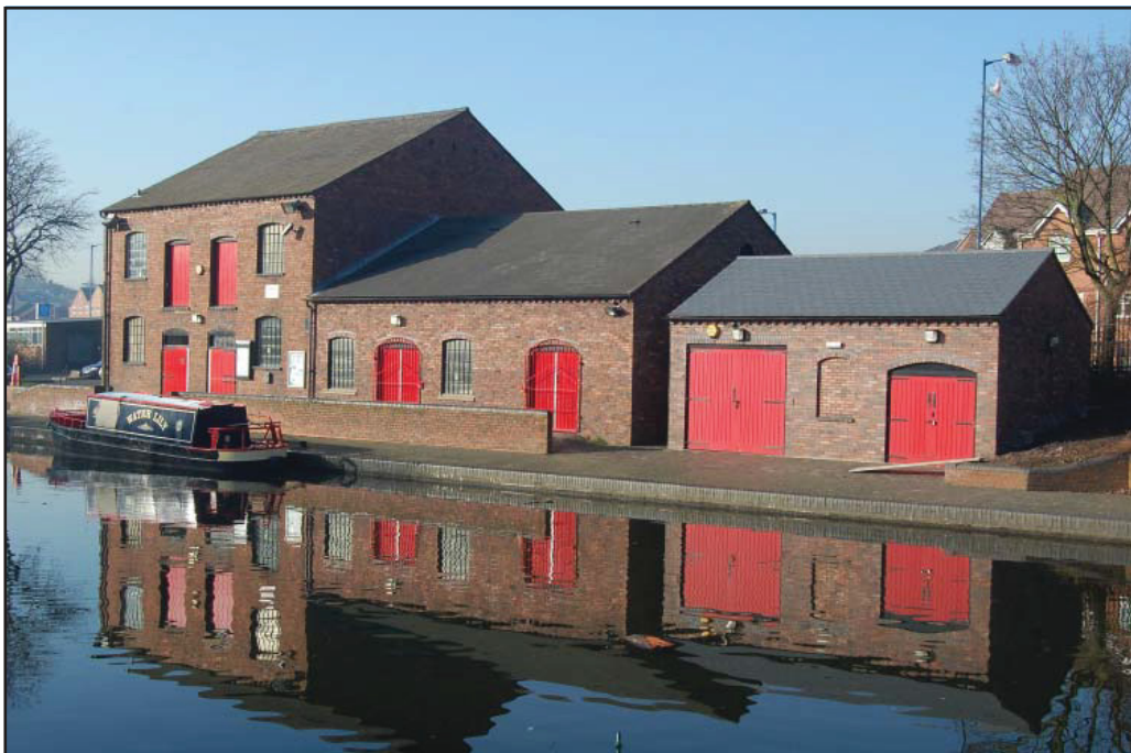
Plate 8: Old Malthouse Stables.
