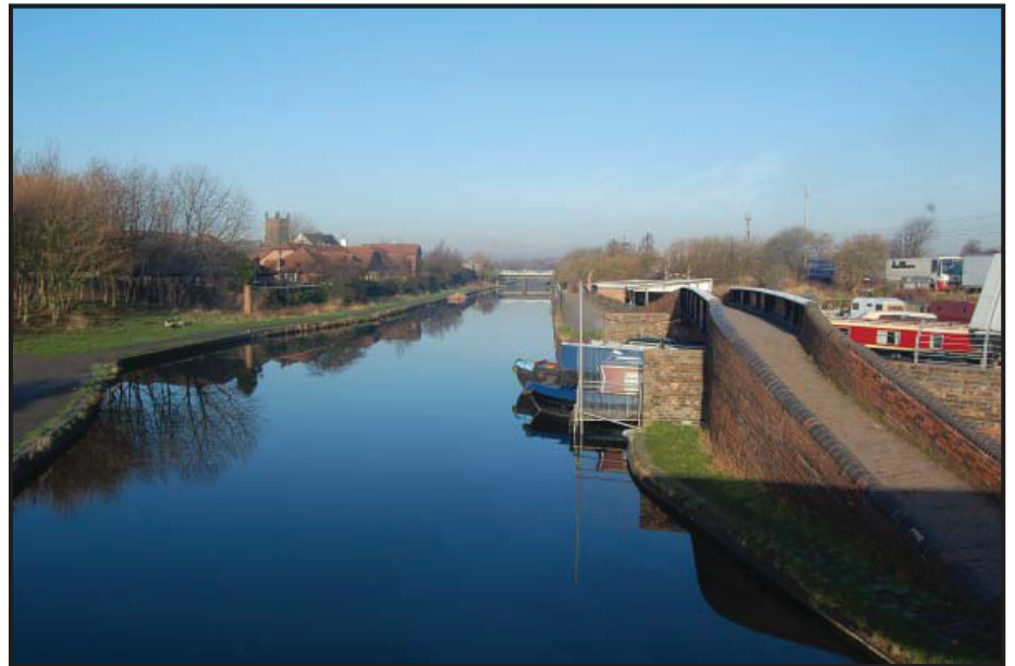
Plate 11: New Line from Waterloo Road Footbridge.
