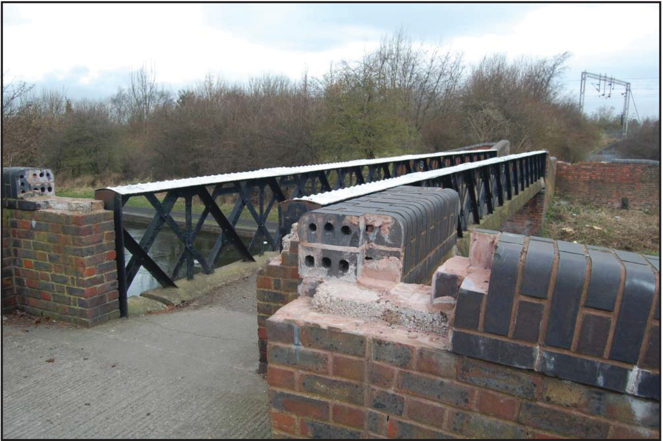
Plate 57: Wood Street Footbridge.
